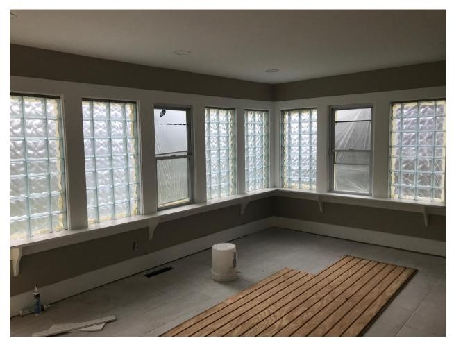
Interior of 1773 Parker Three Season Room, where 6" of additional trim just above the window ledge will allow for a balanced look upon install of Andersen 400 Series windows. Openings are currently 27"x54." The adjustments will be made for a 48" window.
