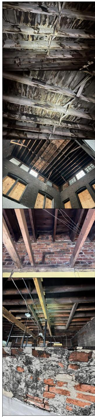
**P-31:** STAINING, MOLD AND ROT ON ROOF SHEATHING AND JOISTS. SUBSTANTIAL REPLACEMENT OF ROOF SHEATHING AND JOISTS REQUIRED. NOTE RIPPED 2X FILLER USED TO CREATE DRAINAGE SADDLES.
