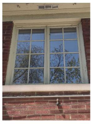
Rotting at frame is allowing moisture into 1st floor ceiling beneath window
