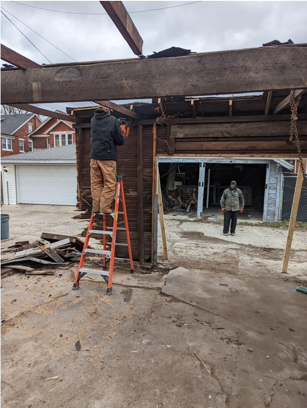
Figure 12 - Most of garage has been demolished and materials hauled away
