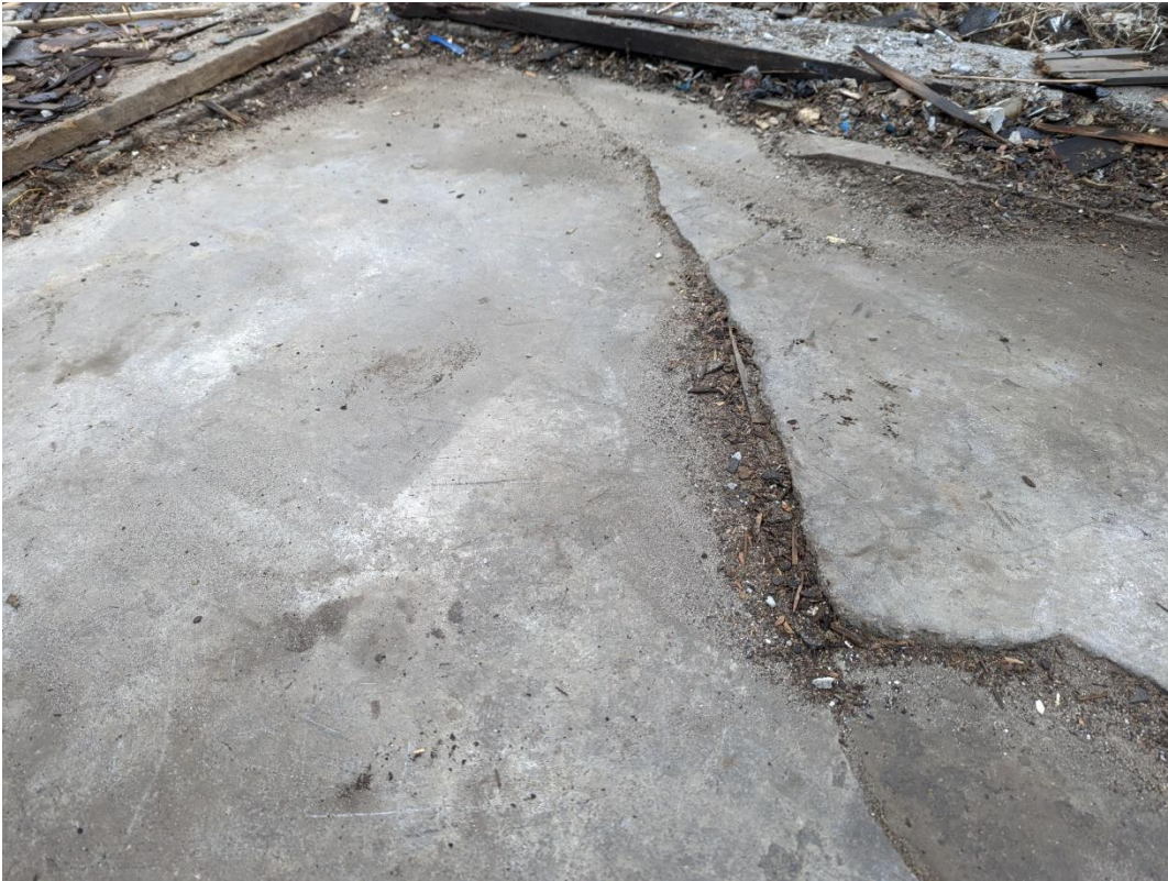
Figure 9 - Concrete slab damaged, needs to be leveled
