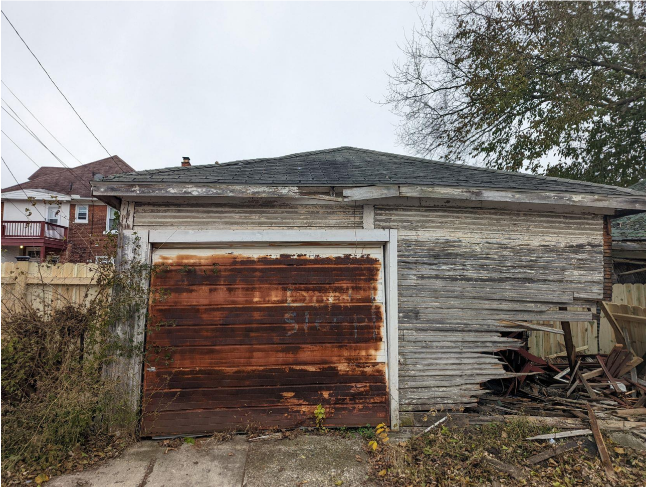
Figure 3 - Back of Garage (alley side) - see corner
