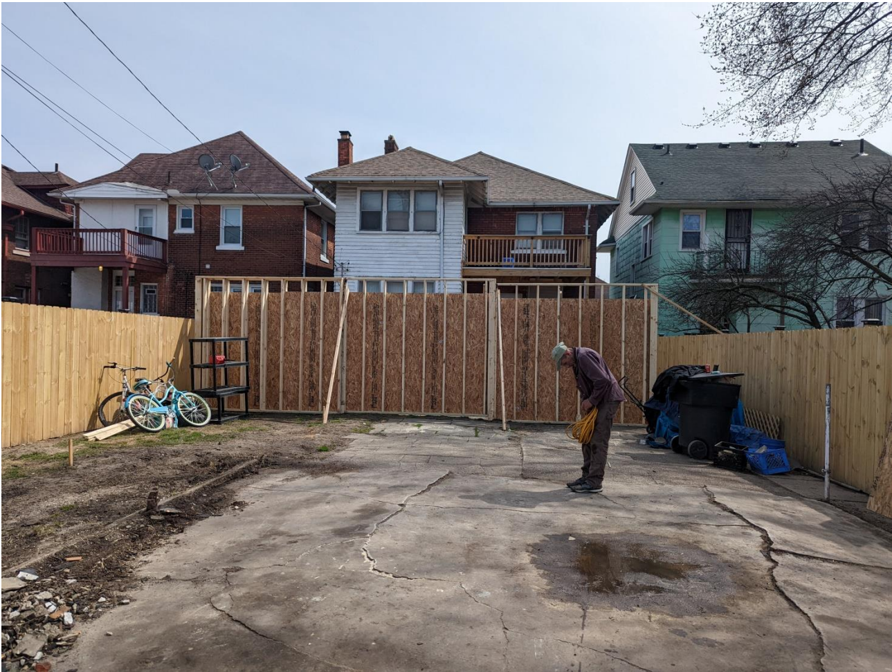
Figure 14 - Demolition completed. New garage to be erected in same area
