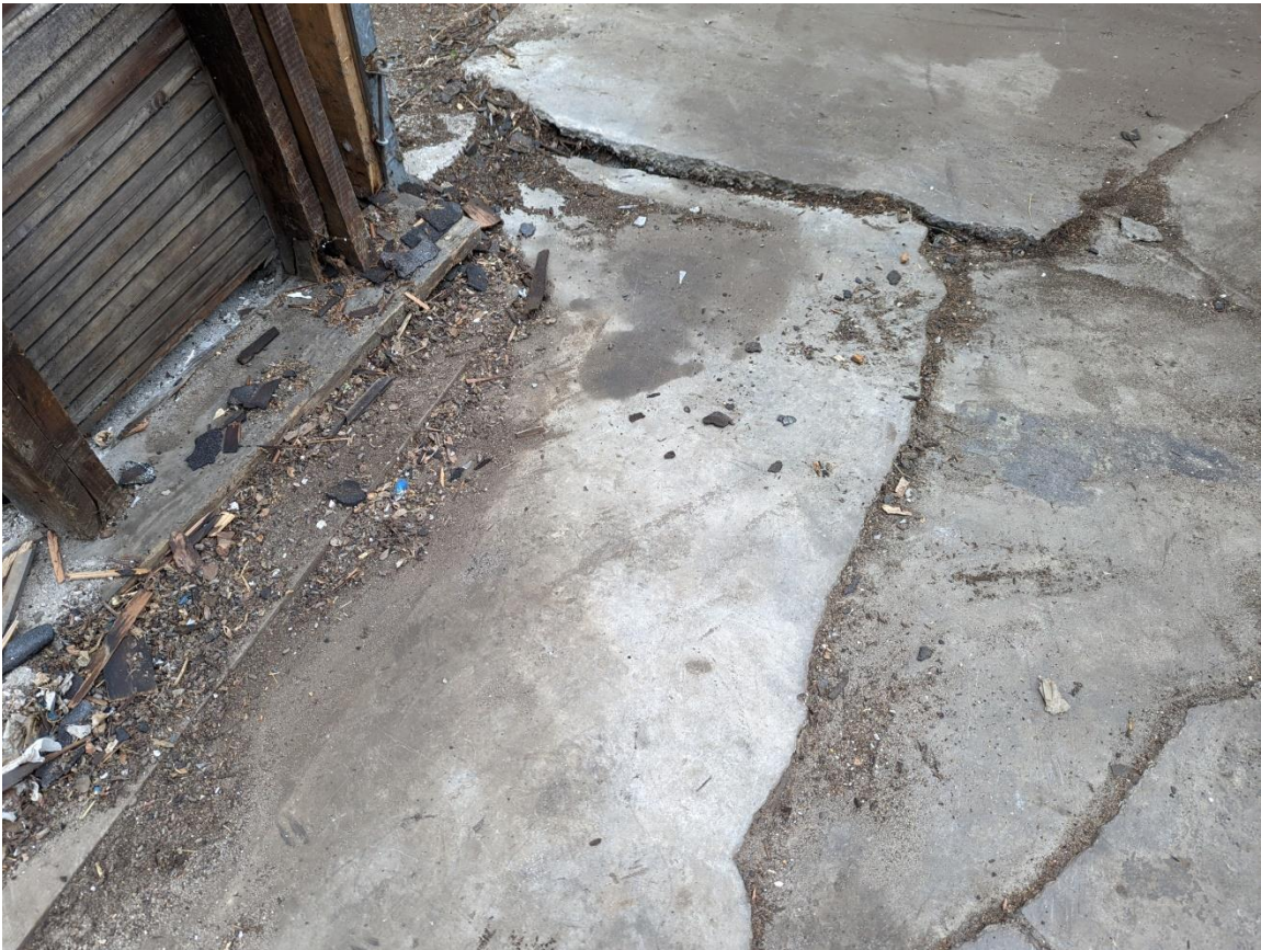
Figure 9 - Concrete slab damaged, needs to be leveled
