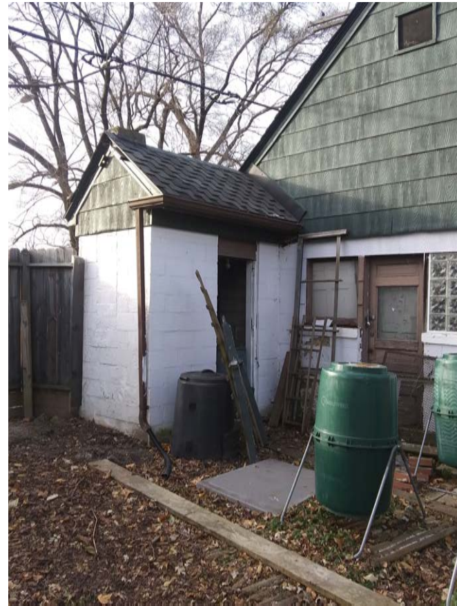
VIEW OF SHED FROM SOUTHEAST
