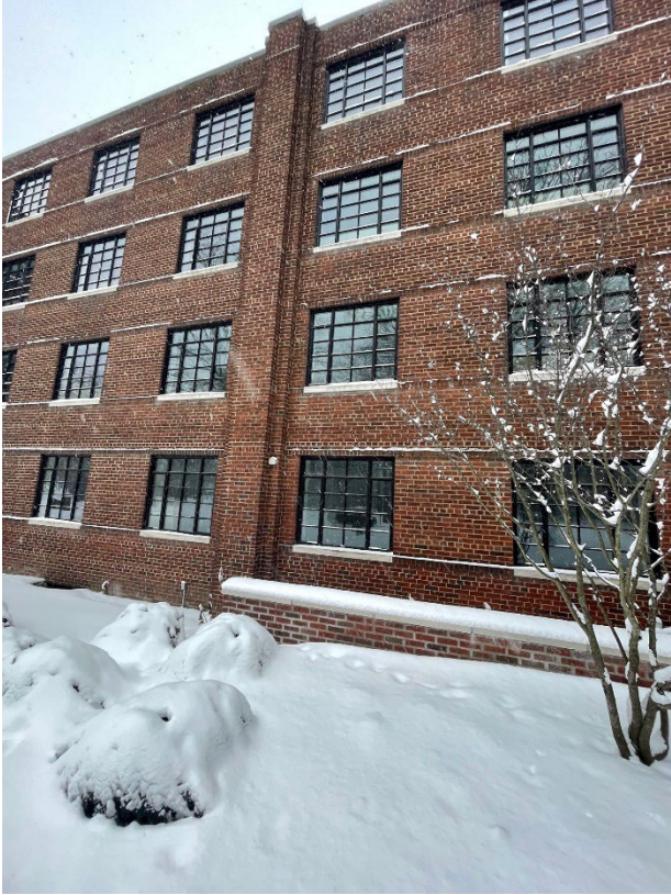
Photo 6: View of 931 Covington (Replacement Windows)
