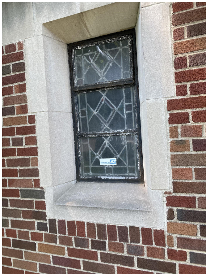
East elevation - Window #1
