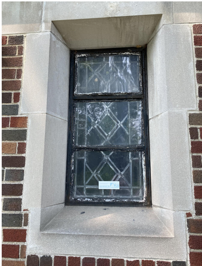
East Elevation - Window #2
