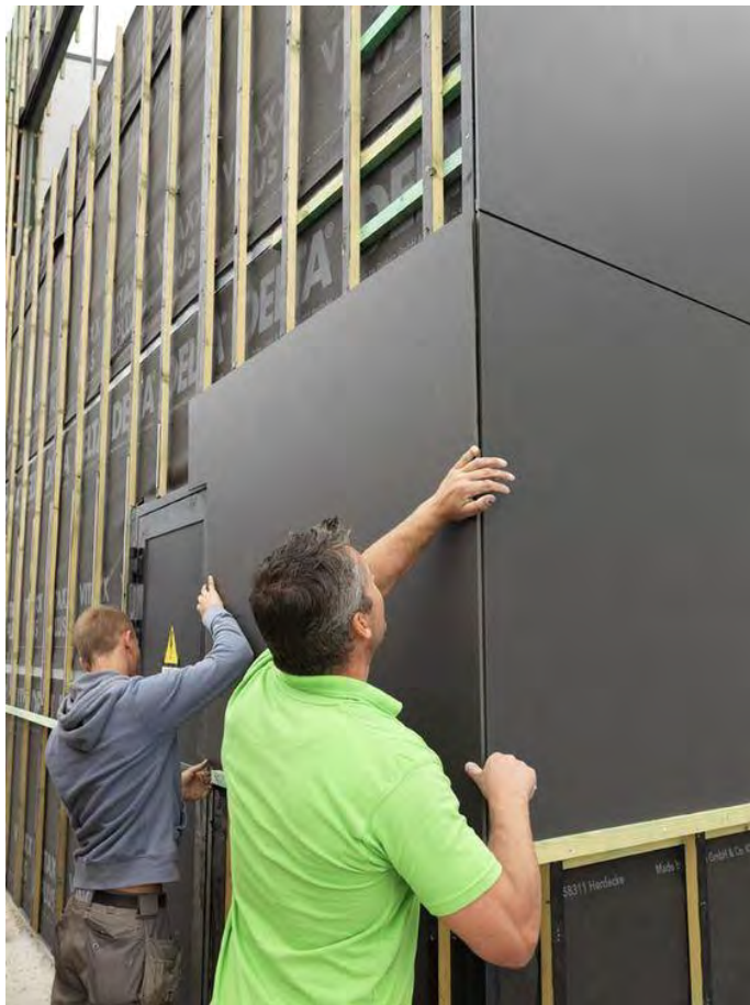
Above: Example photo of HardiePanel vertical siding boards. 4x8 sheets, butt joined with caulking at vertical joints
