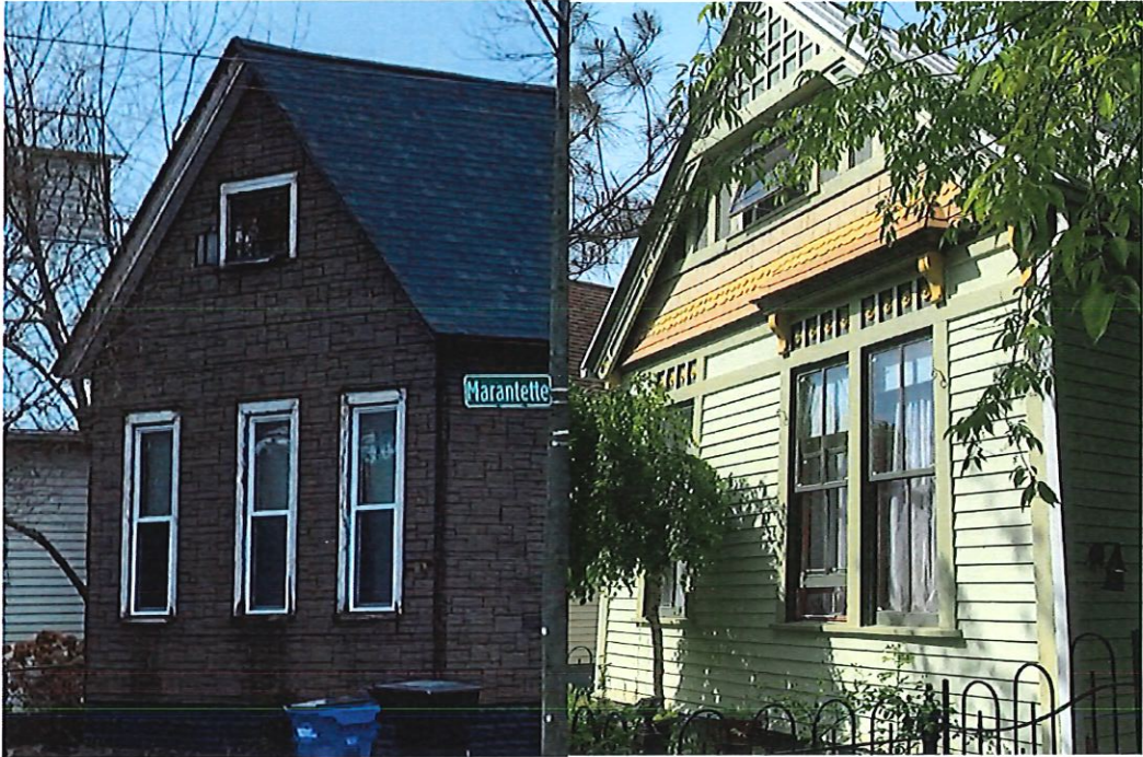
Comparison of neighboring house detail and our house:
