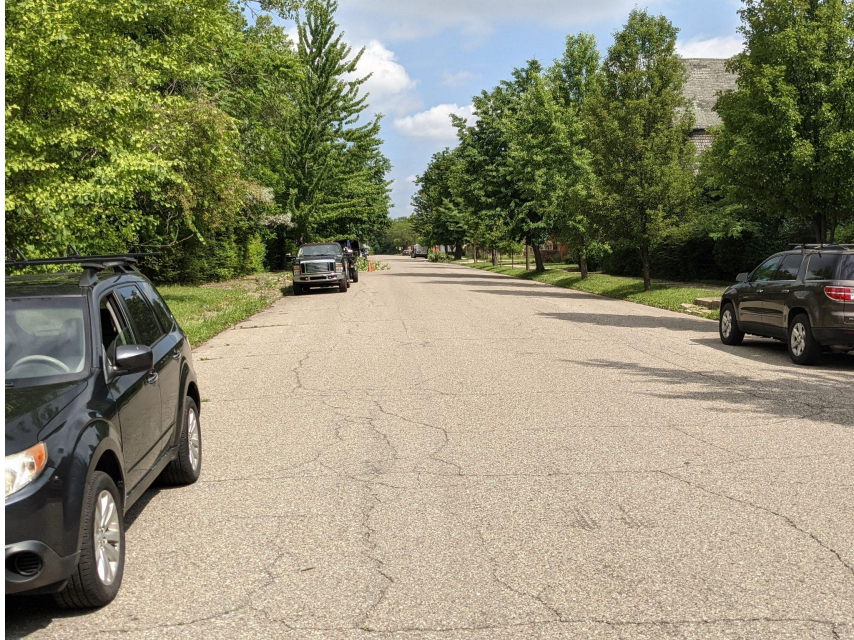
At Alexandrine, looking North towards Willis
