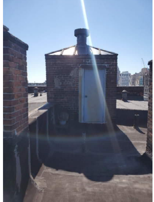
West Elevation of Structure to be Replaced
