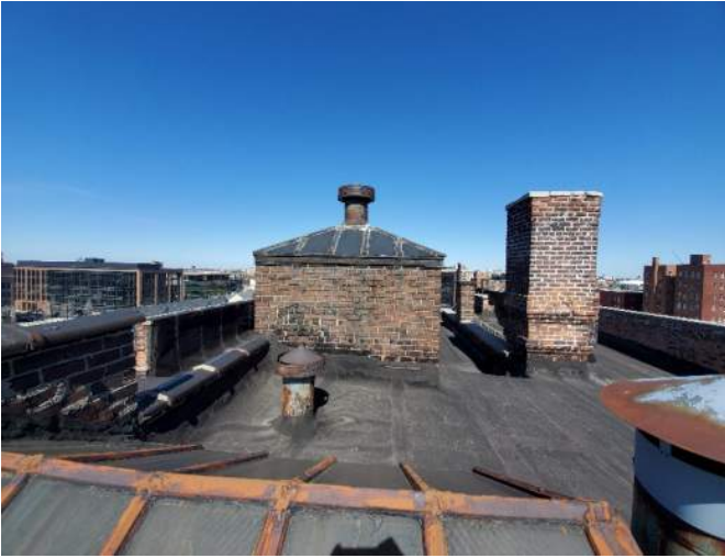
East Elevation of Structure to be Replaced
