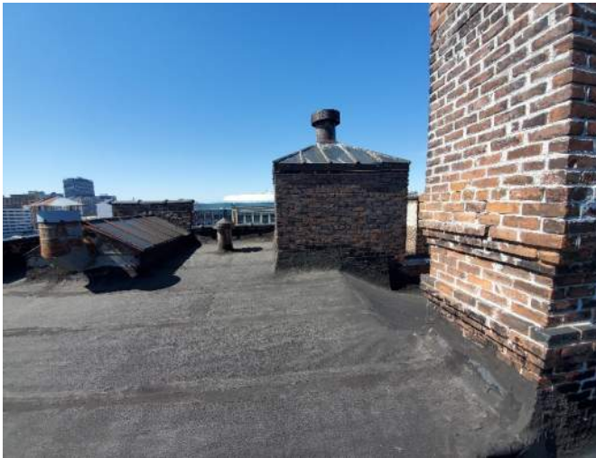
North Elevation of Structure to be Replaced
