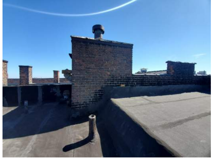
South Elevation of Structure to be Replaced
