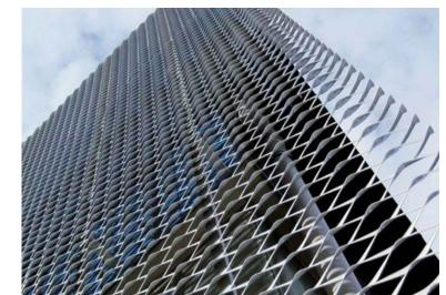
MCNICHOLS EXPANDED METAL MESH FOR STAIRWELL SCREENING
