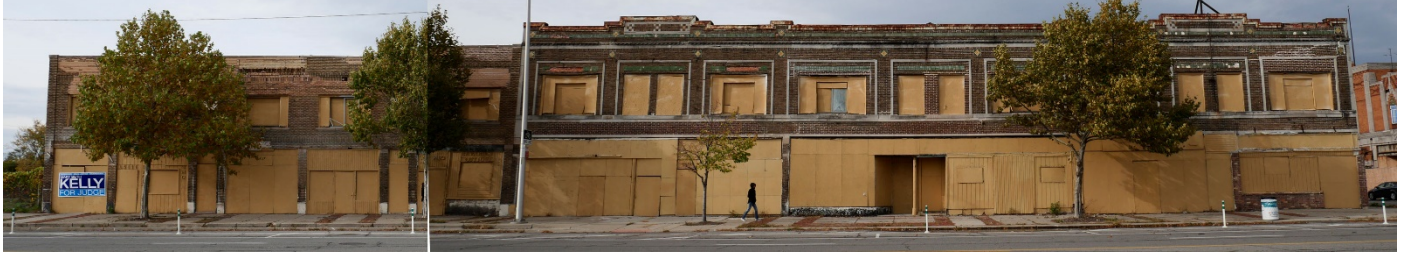
South Facade 14131 (East Jefferson Ave. side)
