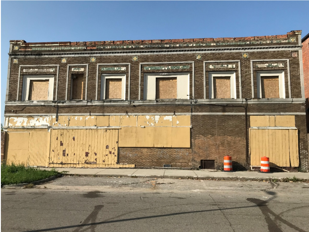
East Facade 14131 (Newport St. side)
