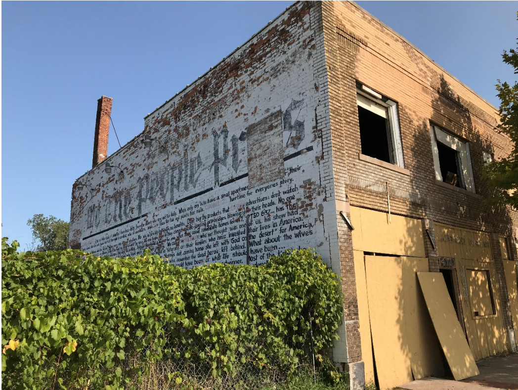
West Facade 14111 (Eastland St. side)
