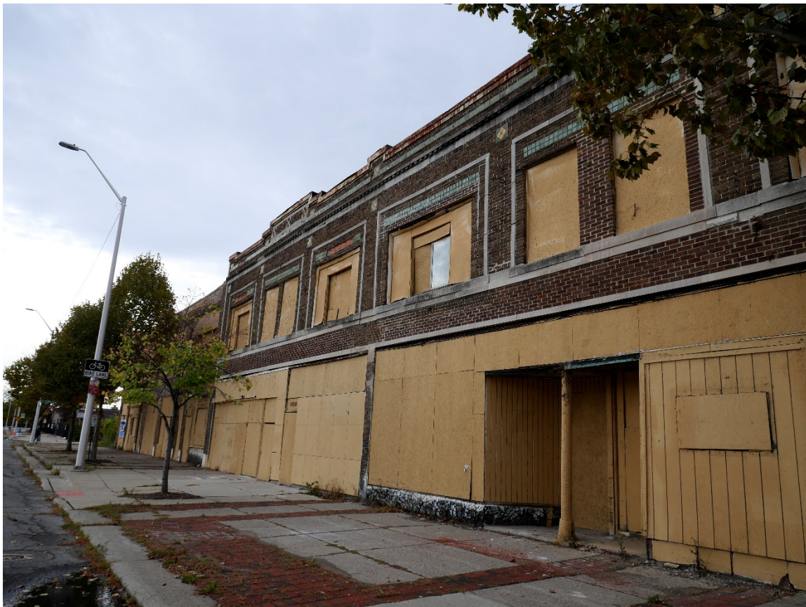
South Facade 14131 (East Jefferson Ave. side)
