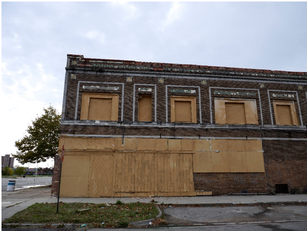
East Facade 14131 (Newport St. side)
