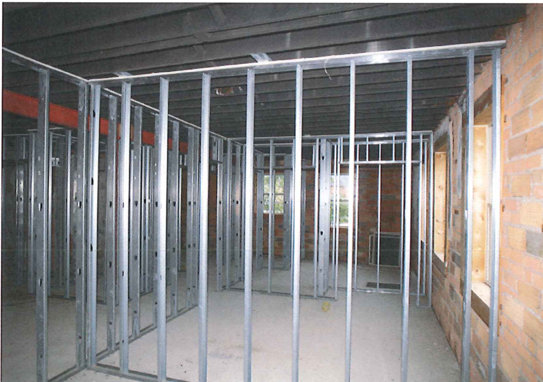
18. Interior View, Second Floor at Southwest, Looking E
