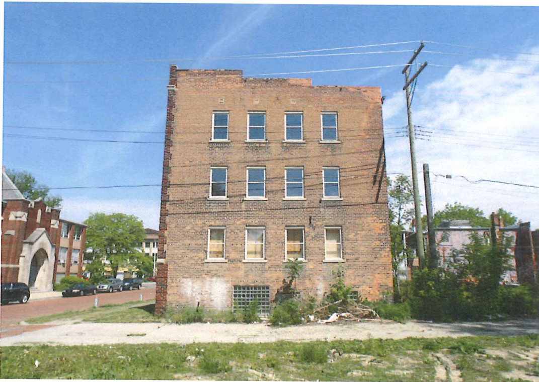
6. Exterior View, South Elevation, Looking N
