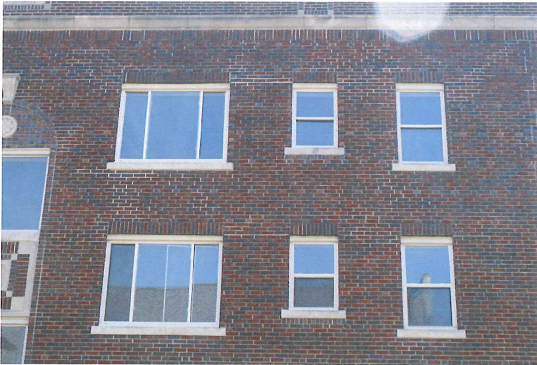
3. Exterior Detail, West Elevation at South, Upper Floors, Looking W
