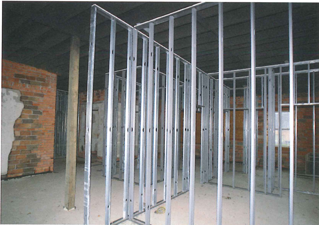
22. Interior View, Third Floor at Southwest, Looking NE
