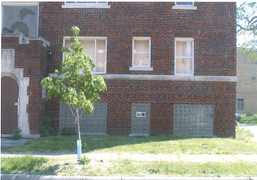
4. Exterior Detail, West Elevation at South, Lower Floors, Looking W
