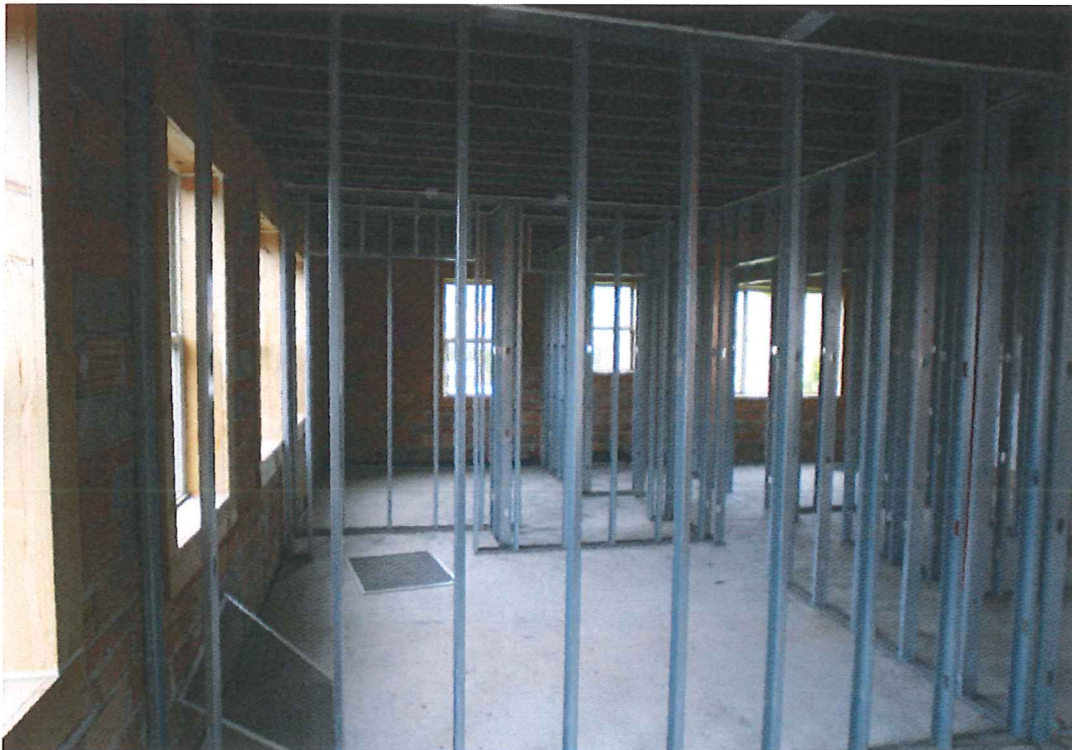
16. Interior View, Second Floor at Center-West, Looking N
