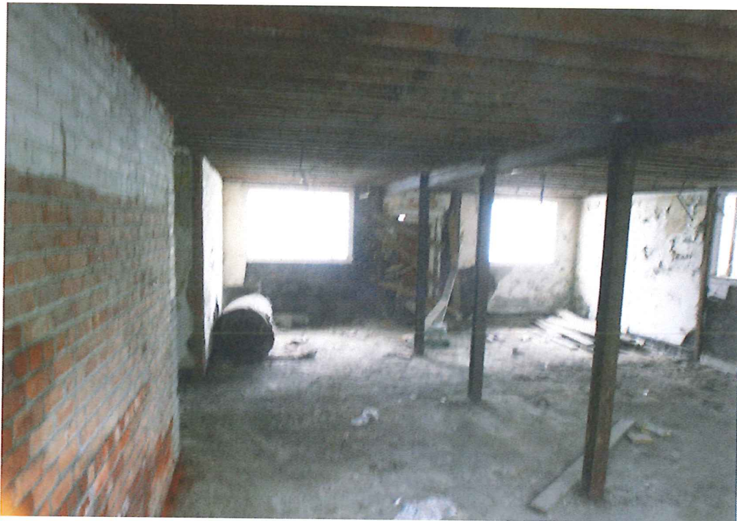
24. Interior View, Basement at Center-East, Looking NW
