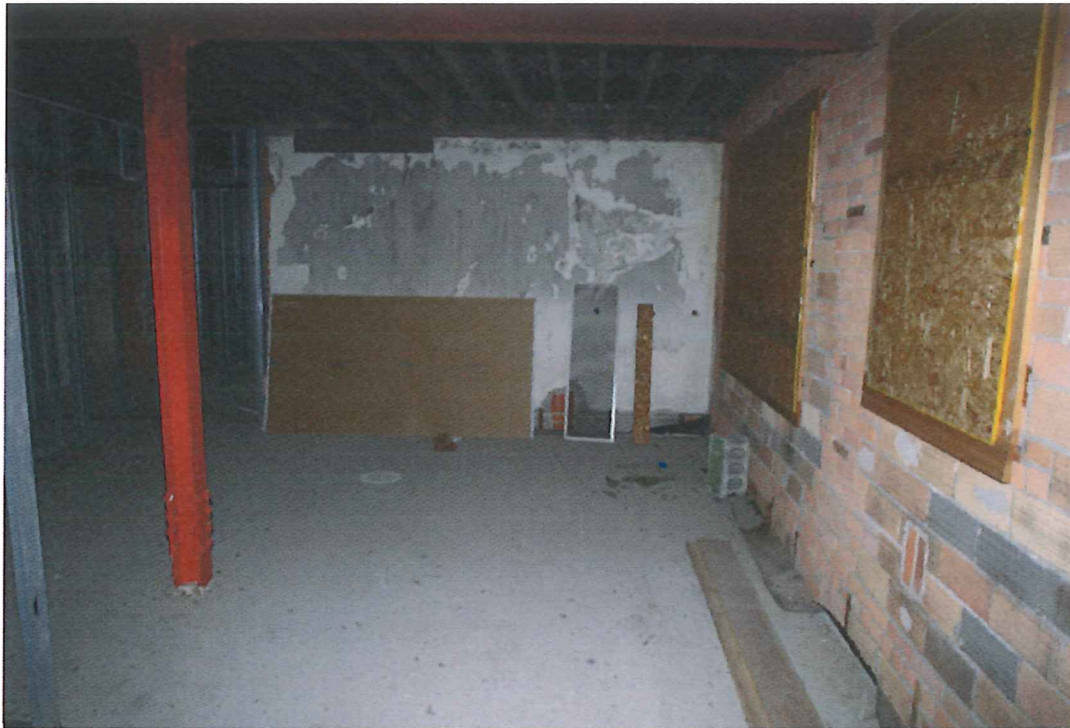
13. Interior View, First Floor at Northwest, Looking S
