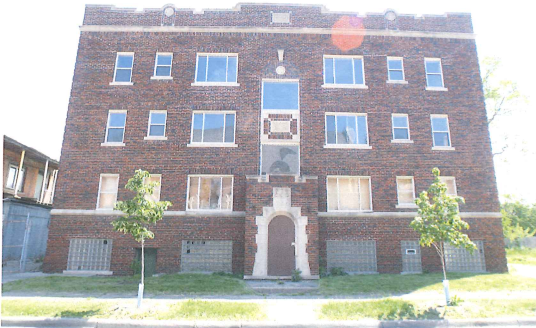
1. Exterior View, West Elevation, Looking E
