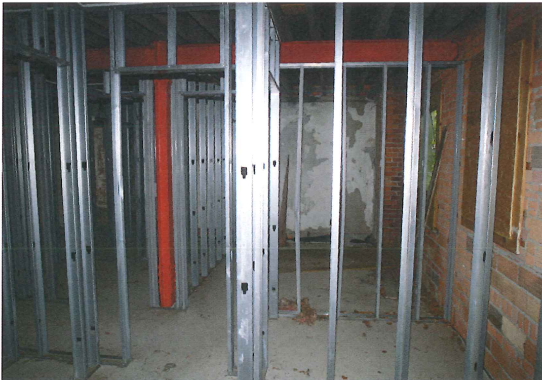
14. Interior View, First Floor at Southeast, Looking N
