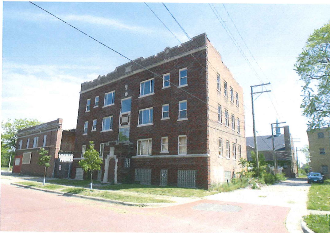
2. Exterior View, West and South Elevations, Looking NE
