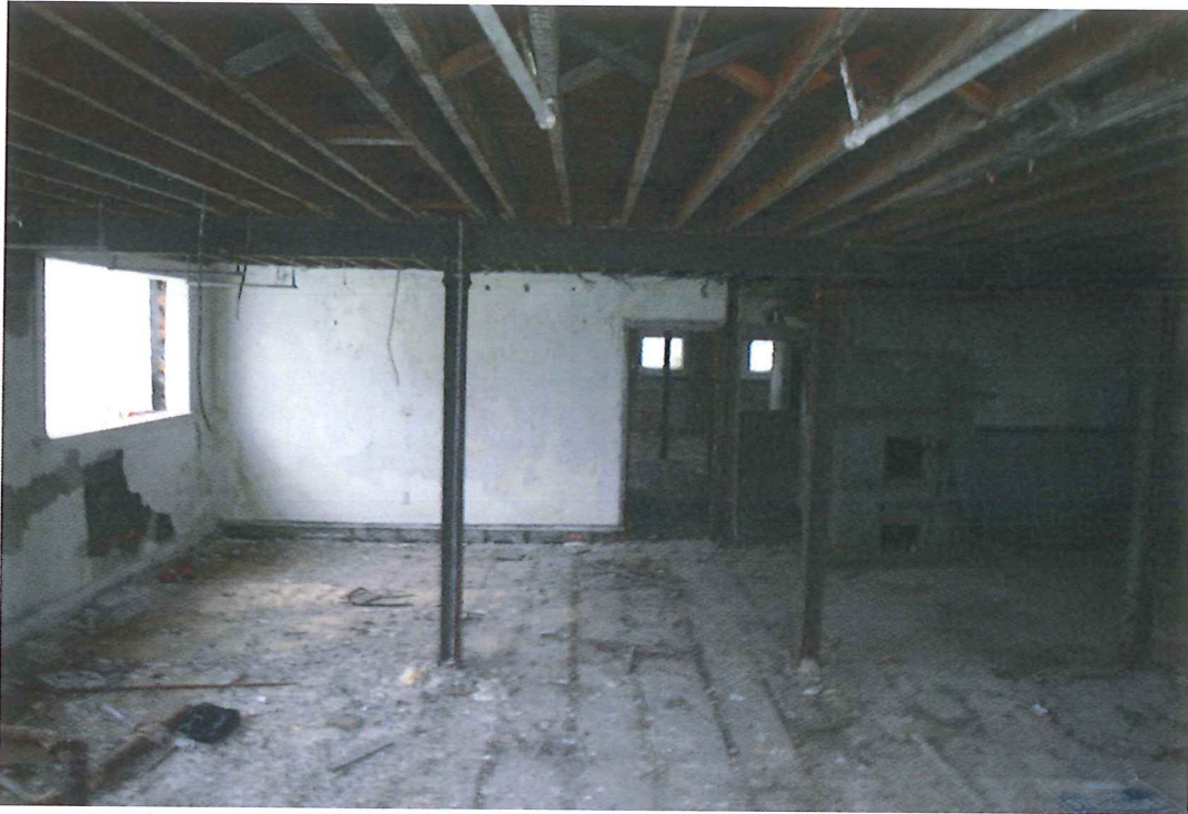
25. Interior View, Basement at Center-South, Looking N
