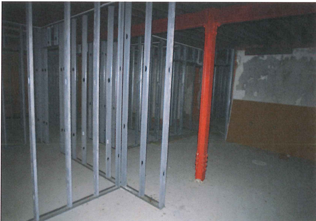
12. Interior View, First Floor at Northwest, Looking SE
