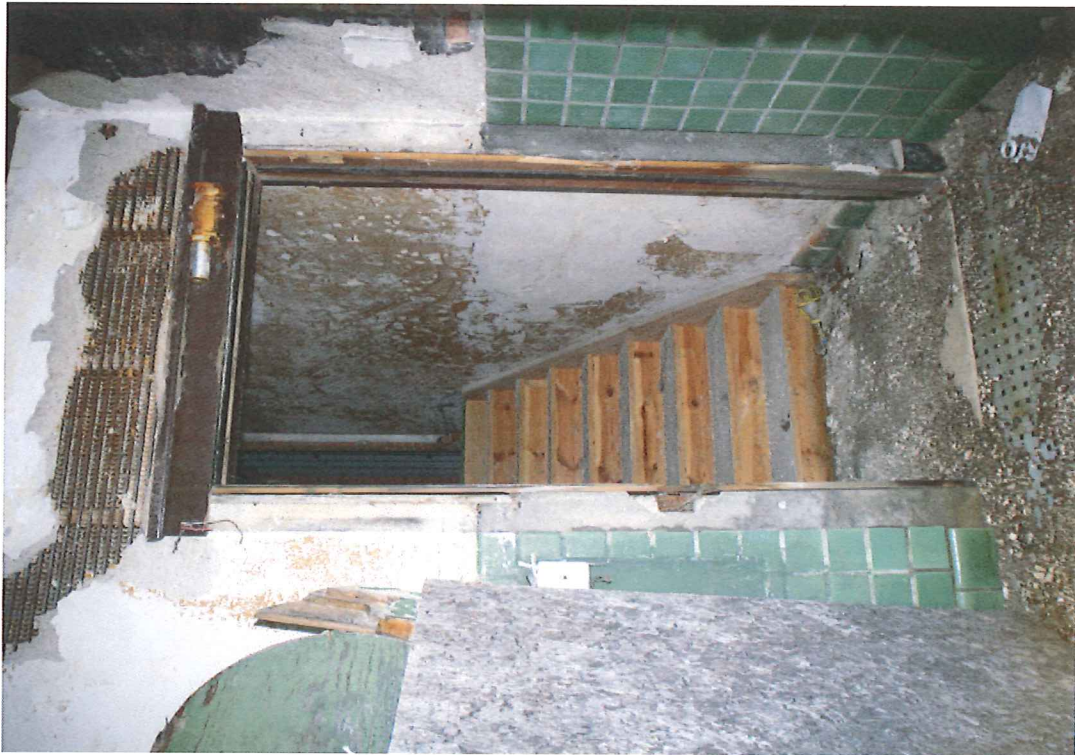
10. Interior View, First Floor, Entry, Looking W
