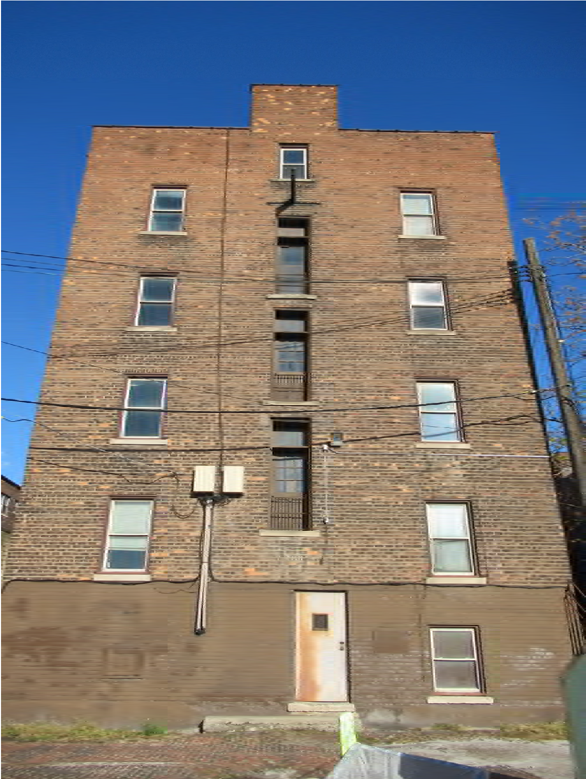
Figure #02: Exterior, South façade, Looking North. 10/28/20.
