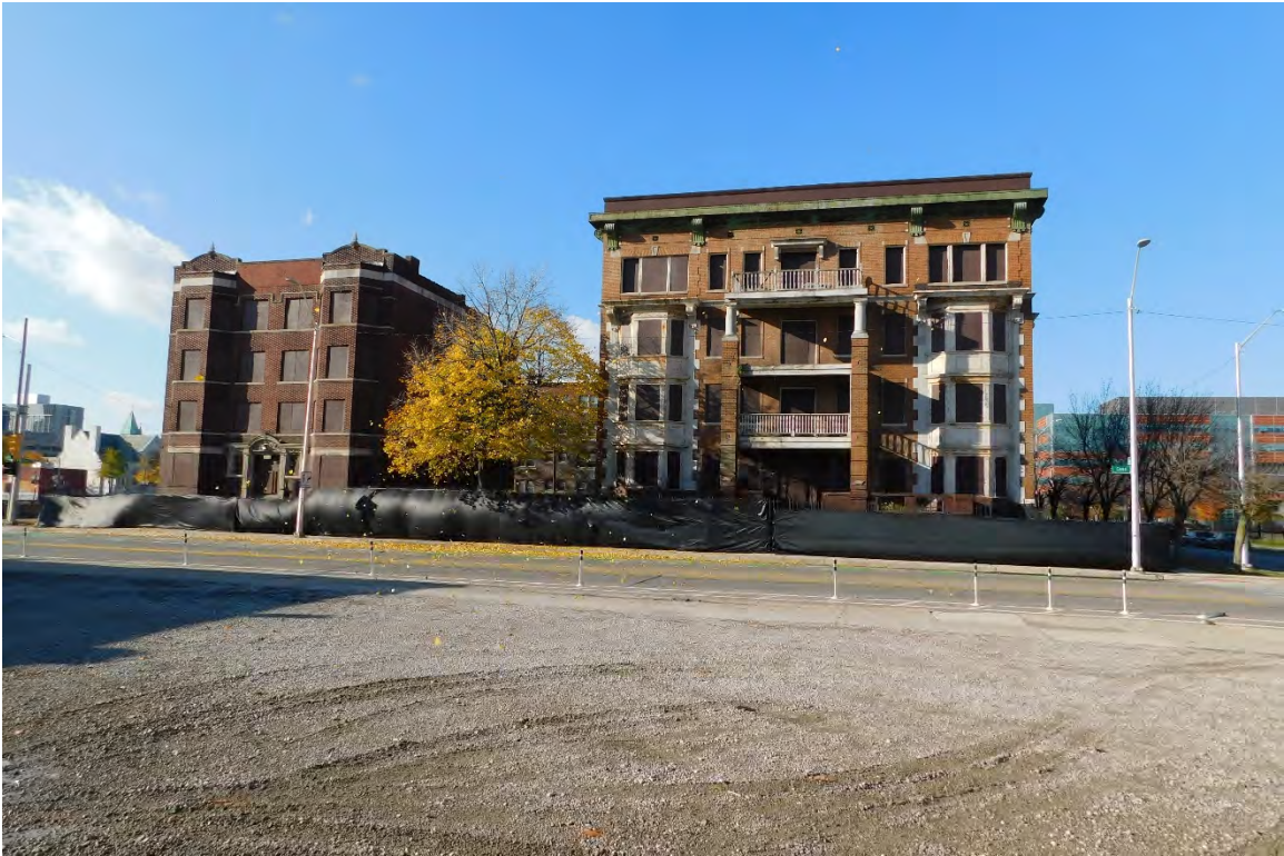
Figure #01: Exterior, 2467 and 2447 Cass, Looking West. 10/28/20.
