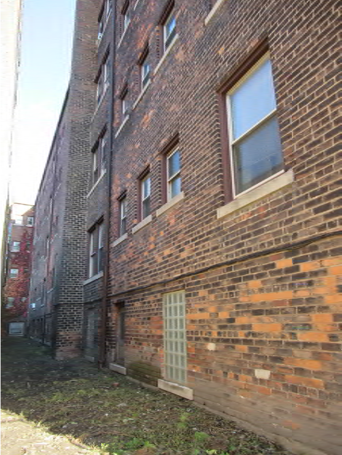
Figure #05: Exterior, West façade detail, Looking Northeast. 10/28/20.
