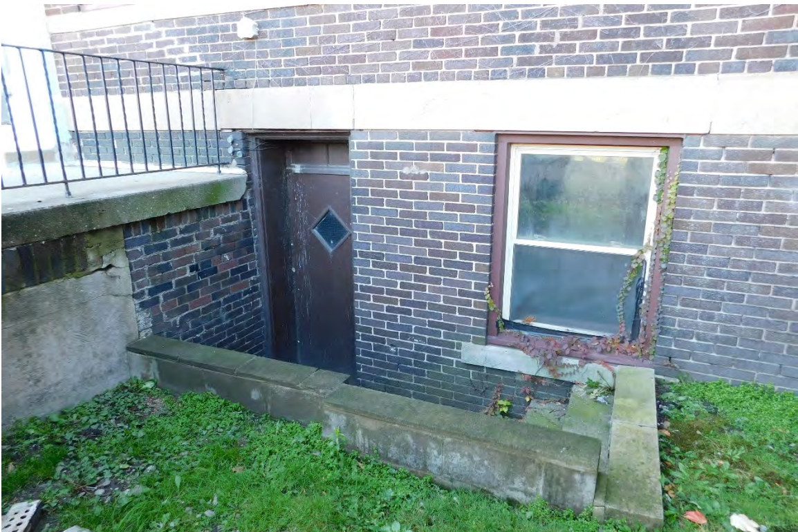
Figure #09: Exterior, Eastern side of North façade, Exterior access to basement, South. 10/28/20.
