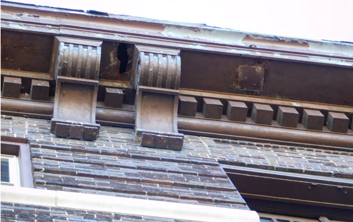
Figure #11: Exterior, North façade pressed tin cornice detail, Looking Up. 10/28/20.
