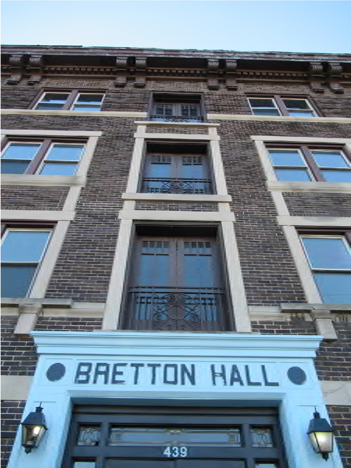
Figure #10: Exterior, North façade Juliet balcony detail, Looking Up. 10/28/20.
