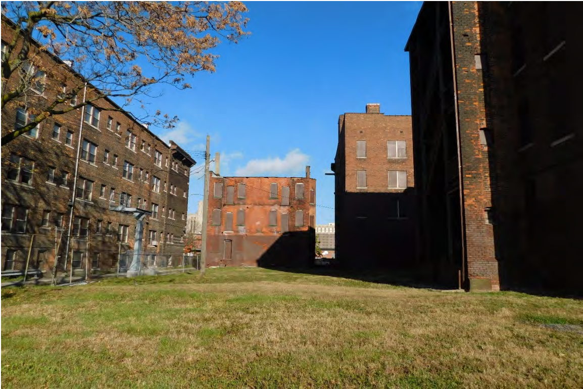
Figure #05: Exterior, Grassy area flanked by 439 Henry, 427 Henry, 2467 Cass, and 2447 Cass, Looking North. 10/28/20.
