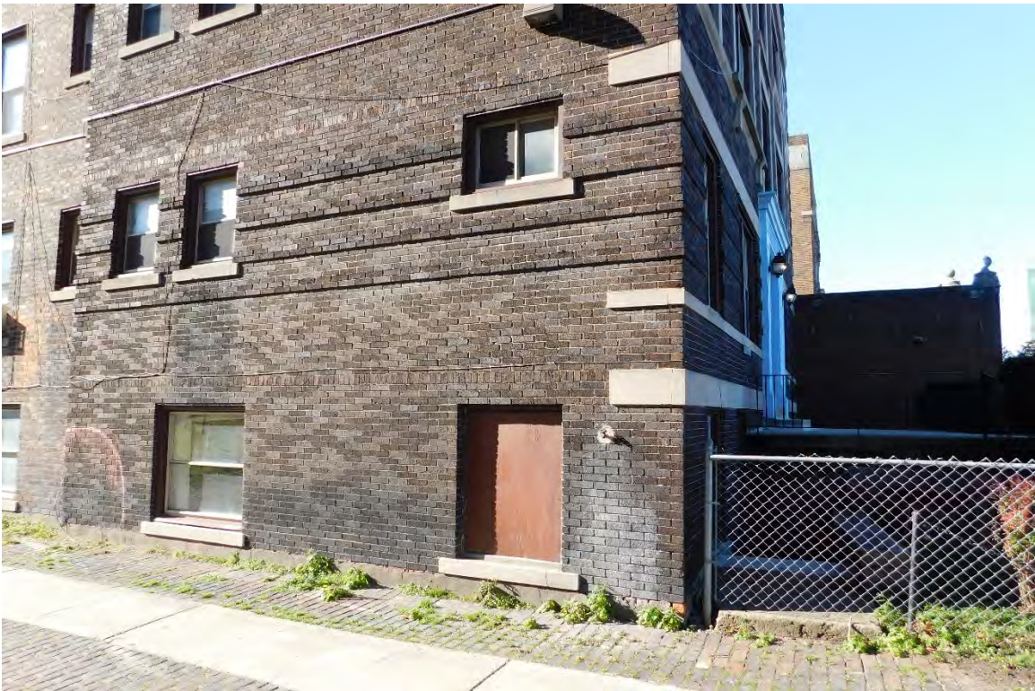
Figure #14: Exterior, East façade detail, Looking West. 10/28/20.
