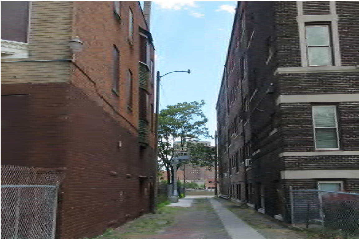
Figure #08: Exterior, Alley between 427 and 439 Henry, Looking South. 10/28/20.
