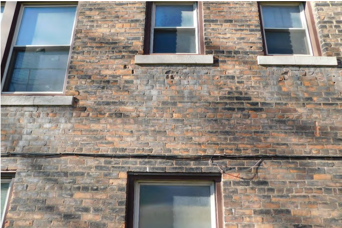
Figure #12: Exterior, East façade masonry detail, Looking West. 10/28/20.
