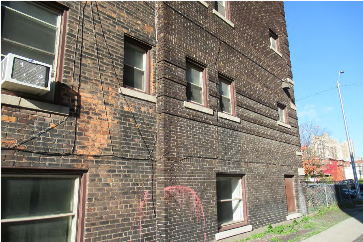
Figure #13: Exterior, East façade masonry detail, Looking Northwest. 10/28/20.
