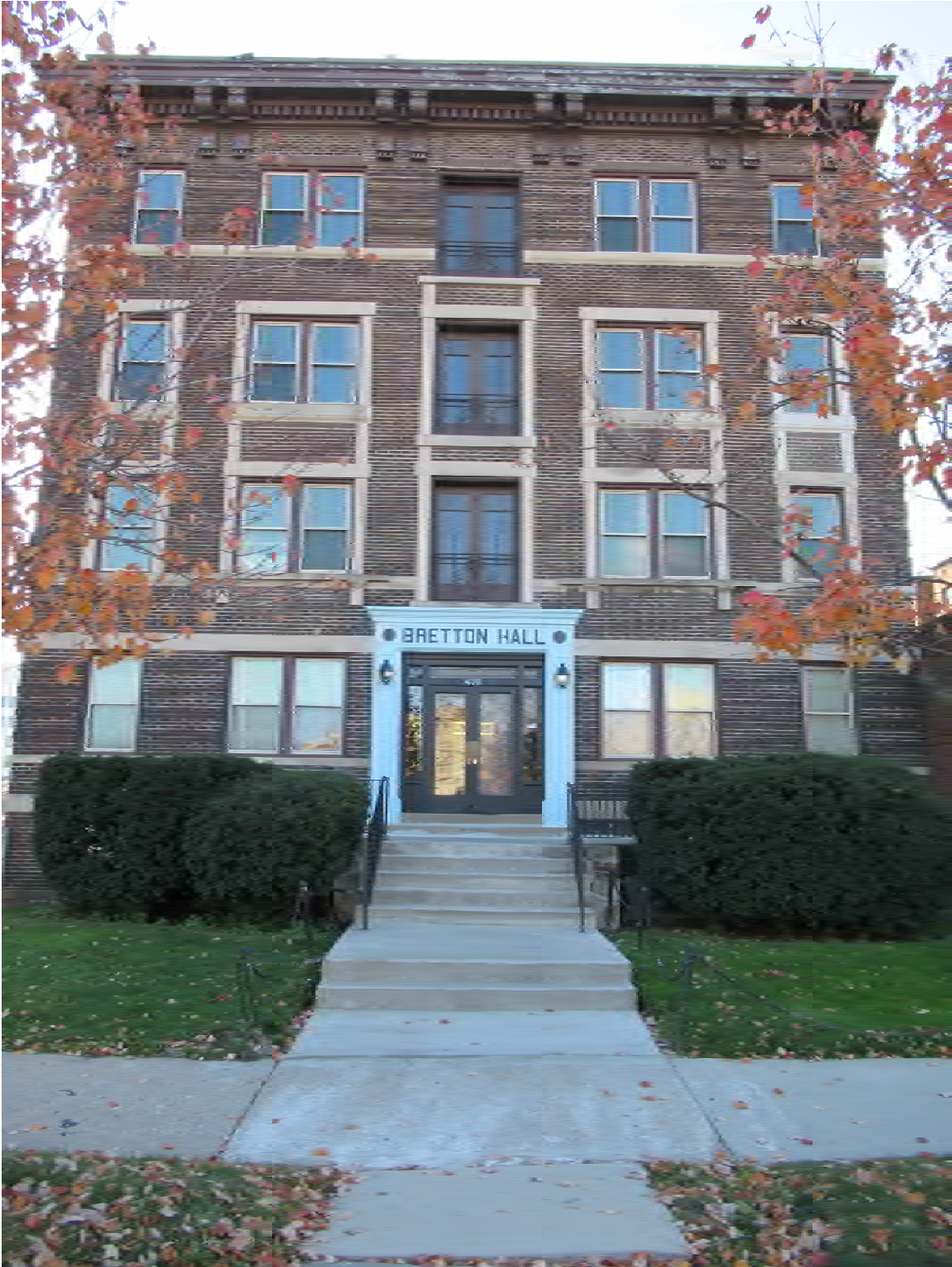
Figure #01: Exterior, North façade, Looking South. 10/28/20.
