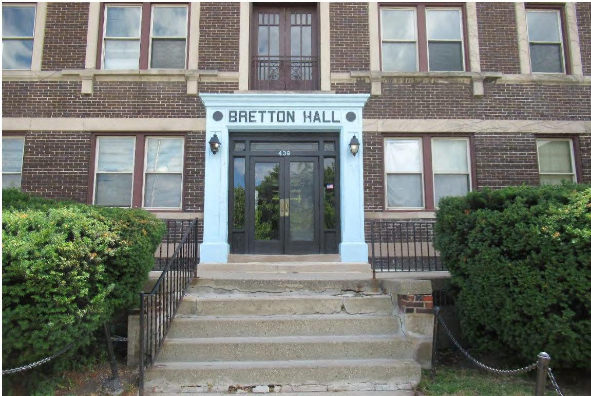
Figure #06: Exterior, North façade main entrance, Looking South. 10/28/20.
