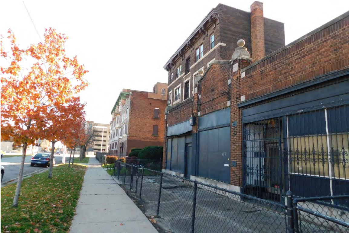
Figure #03: Exterior, Henry Street streetscape, Looking East. 10/28/20.
