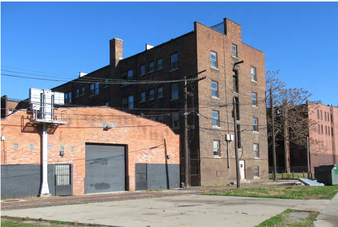
Figure #04: Exterior, South and West façades, Looking Northeast. 10/28/20.
