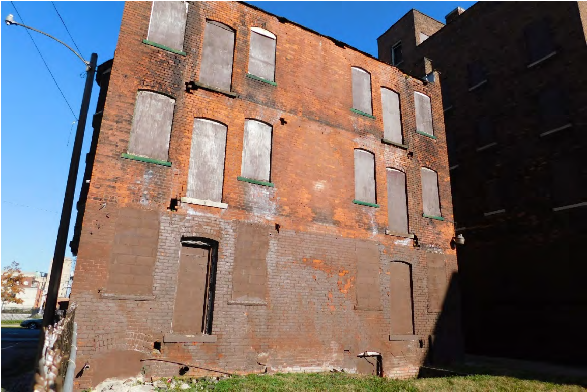
Figure #05: Exterior, South façade, Looking North. 10/28/20.
