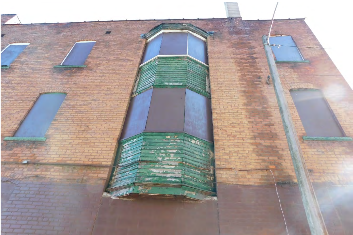
Figure #13: Exterior, West façade bay window detail, Looking Up. 10/28/20.
