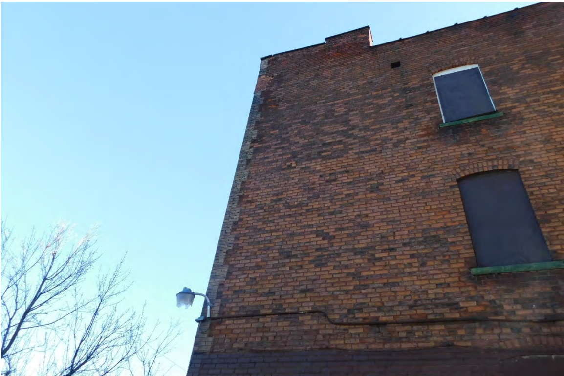
Figure #17: Exterior, West façade masonry detail, Looking East. 10/28/20.
