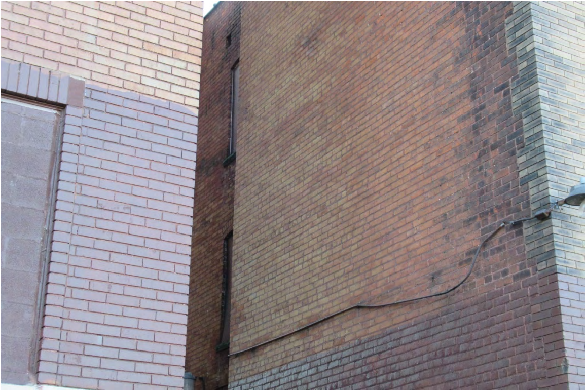
Figure #18: Exterior, East façade masonry detail, Looking Southwest. 10/28/20.
