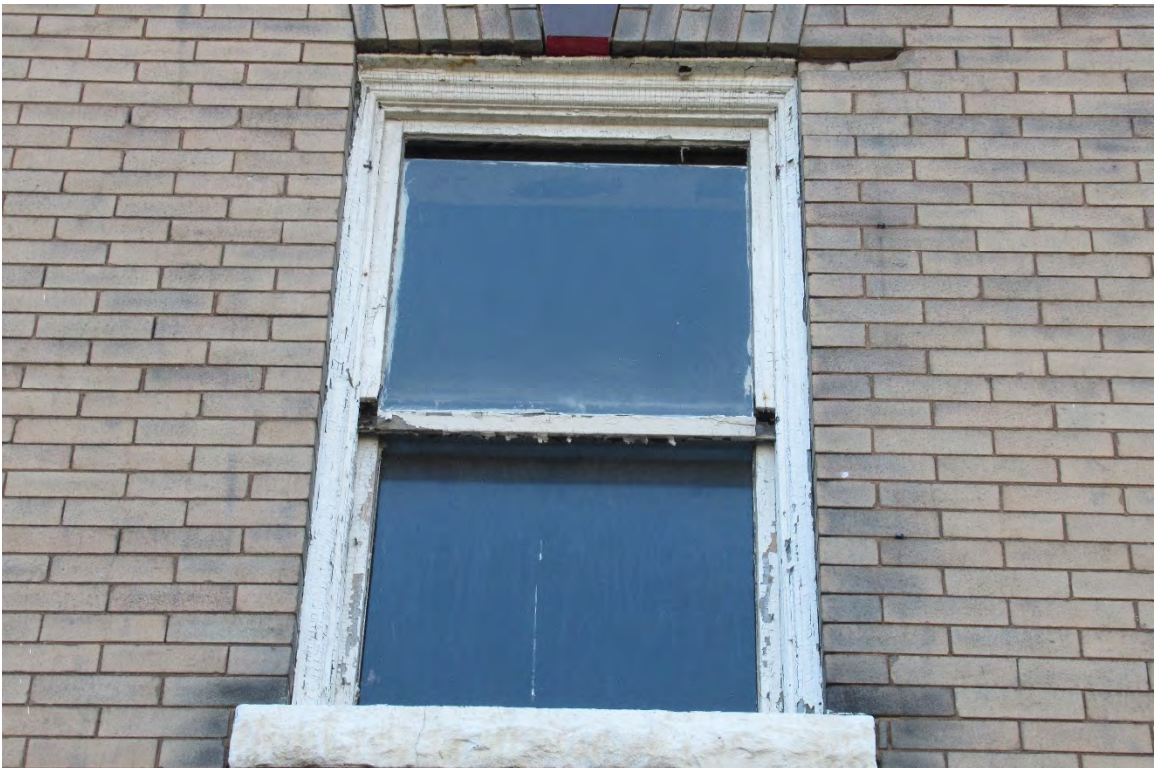
Figure #11: Exterior, North façade wood window detail, Looking Up. 10/28/20.
