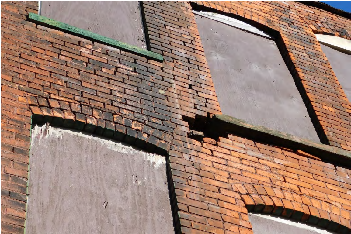
Figure #19: Exterior, South façade masonry detail, Looking Up. 10/28/20.
