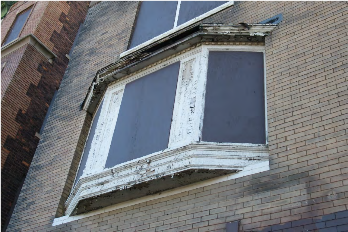
Figure #12: Exterior, North façade bay window detail, Looking Up. 10/28/20.
