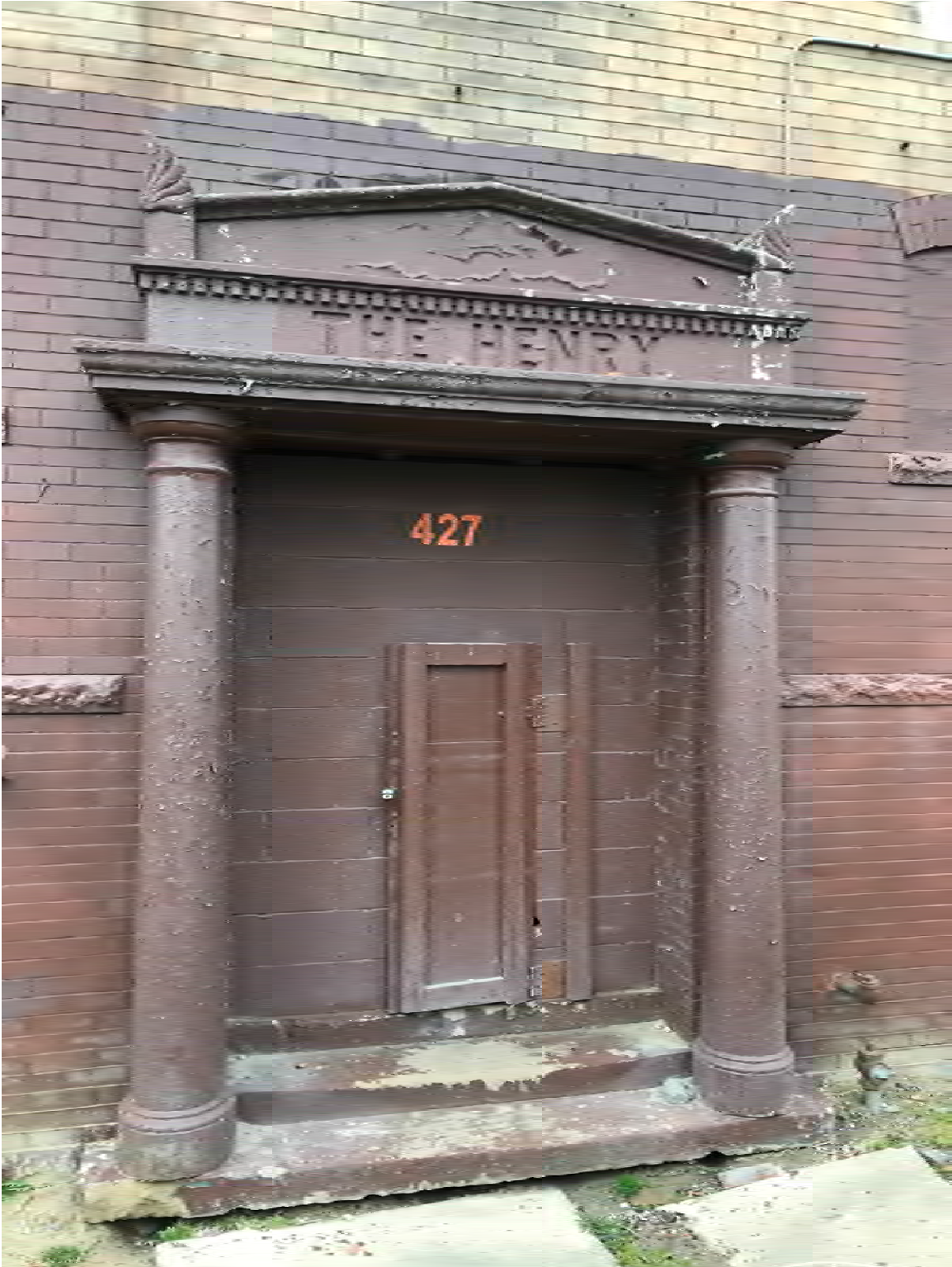
Figure #07: Exterior, North façade Main Entrance, Looking South. 10/28/20.
