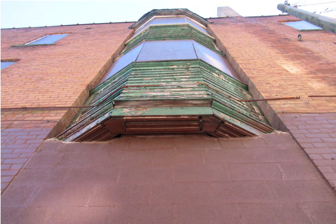
Figure #14: Exterior, West façade bay window detail, Looking Up. 10/28/20.
