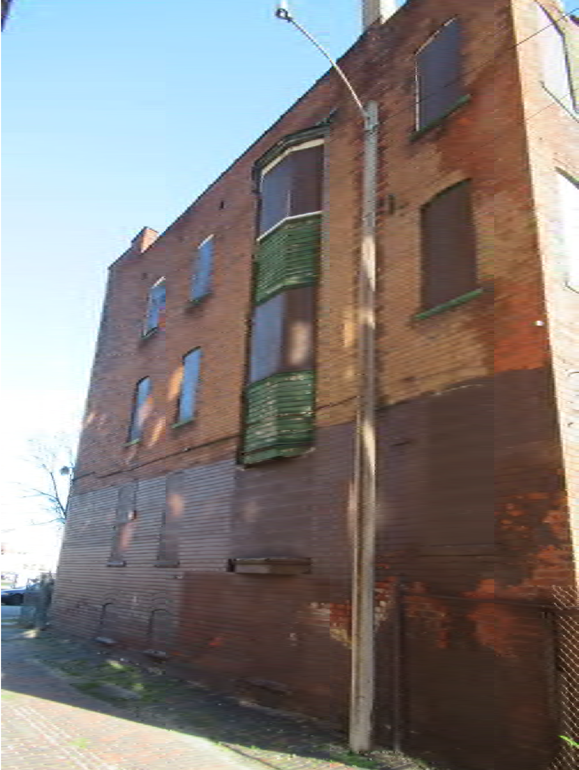
Figure #03: Exterior, West façade, Looking Northeast. 10/28/20.
