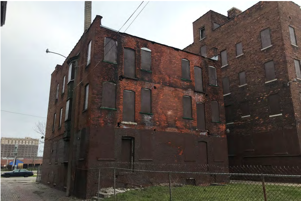
Figure #06: Exterior, South façade, Looking Northeast. 04/24/20.
