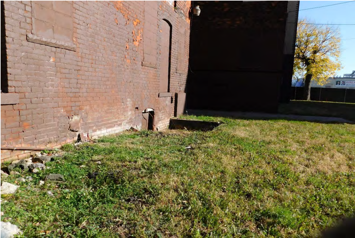
Figure #20: Exterior, South façade first floor, Looking East. 10/28/20.
