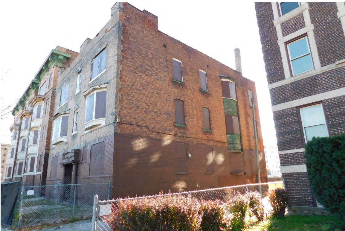
Figure #02: Exterior, West façade, Looking Southeast. 10/28/20.
