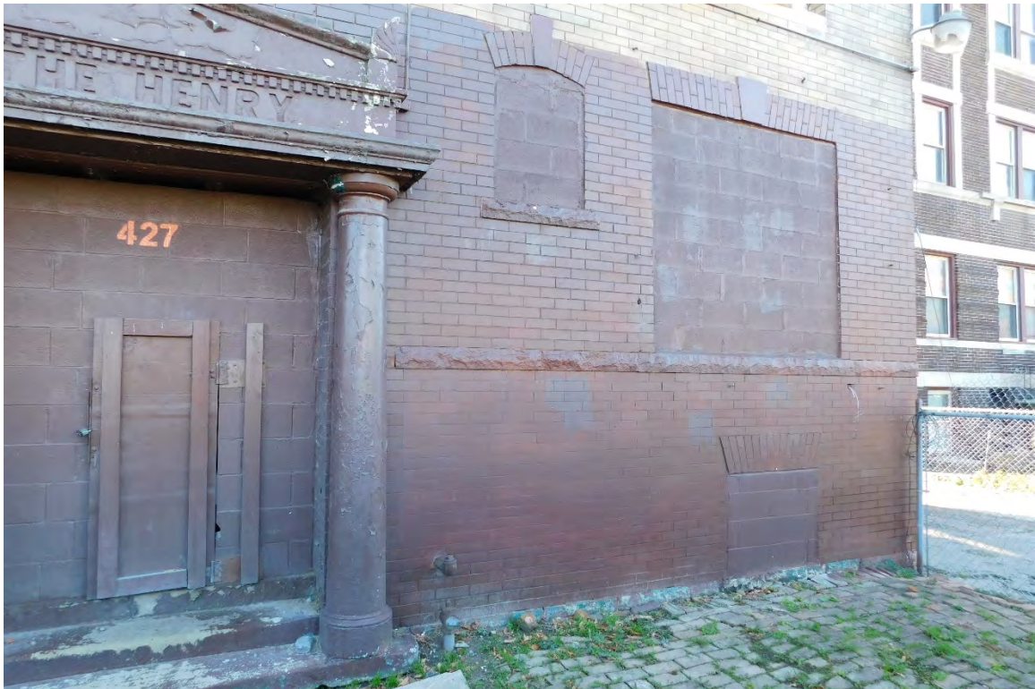
Figure #08: Exterior, North façade first floor, Looking Southwest. 10/28/20.
