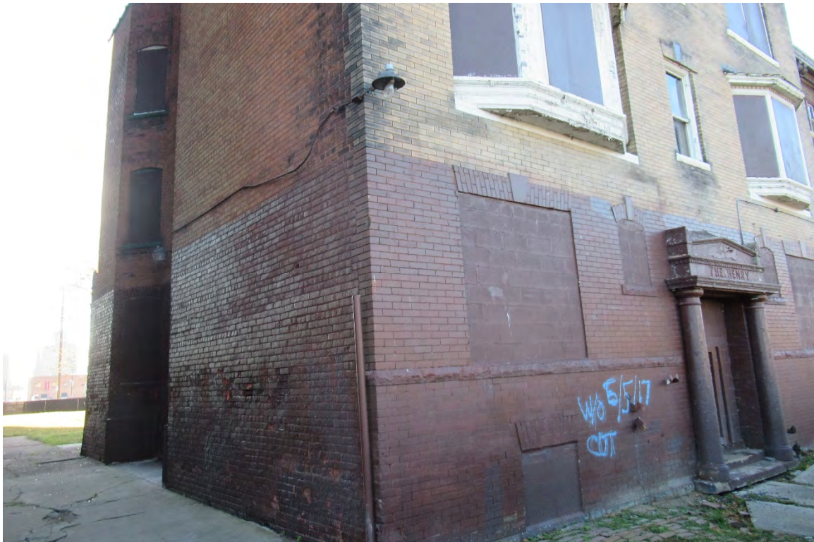
Figure #09: Exterior, North and East façades first floor, Looking Southwest. 10/28/20.
