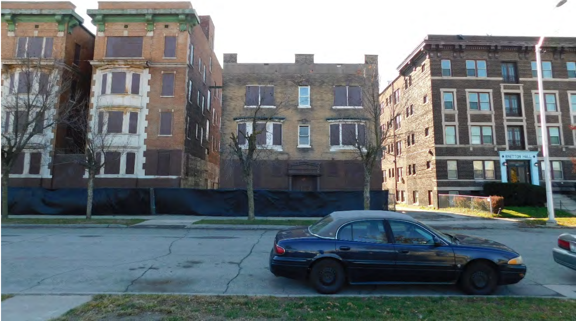
Figure #01: Exterior, North façade, Looking South. 10/28/20.
