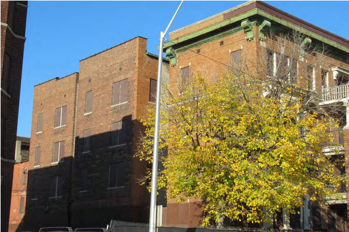
Figure #05: Exterior, South façade, Looking Northwest. 10/28/20.
