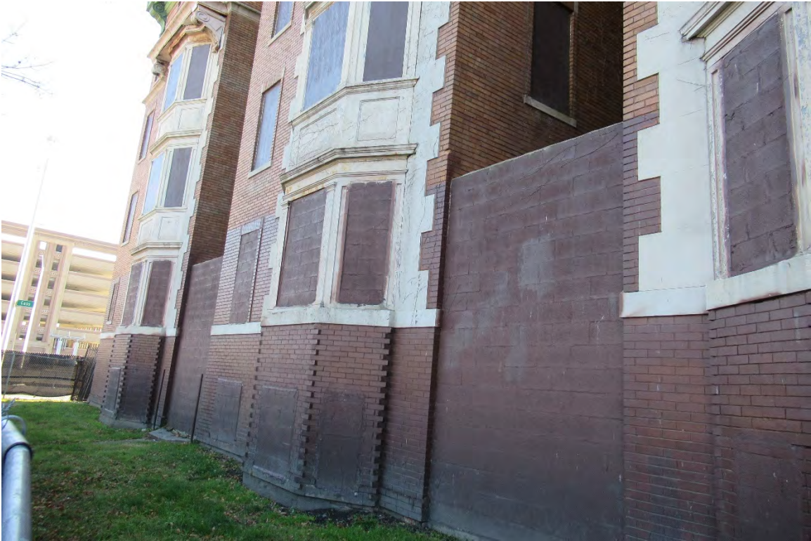
Figure #18: Exterior, North façade first floor masonry detail, Looking South. 10/28/20.
