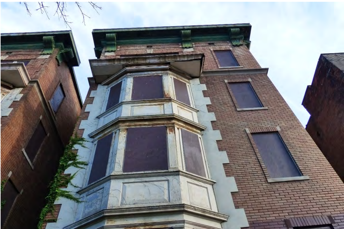
Figure #17: Exterior, North façade bay window detail, Looking South. 10/28/20.
