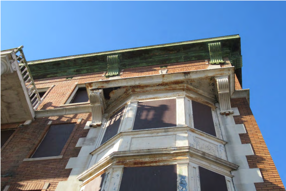
Figure #12: Exterior, East façade first floor bay window detail, Looking Up, 10/28/20.
