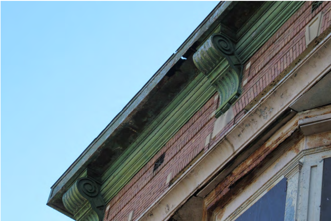
Figure #19: Exterior, North façade cornice detail, Looking Up. 10/28/20.
