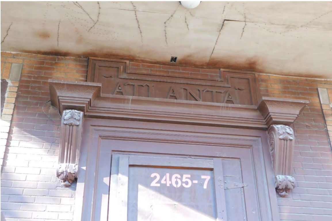
Figure #09: Exterior, East façade first floor entablature detail, Looking Up. 10/28/20.
