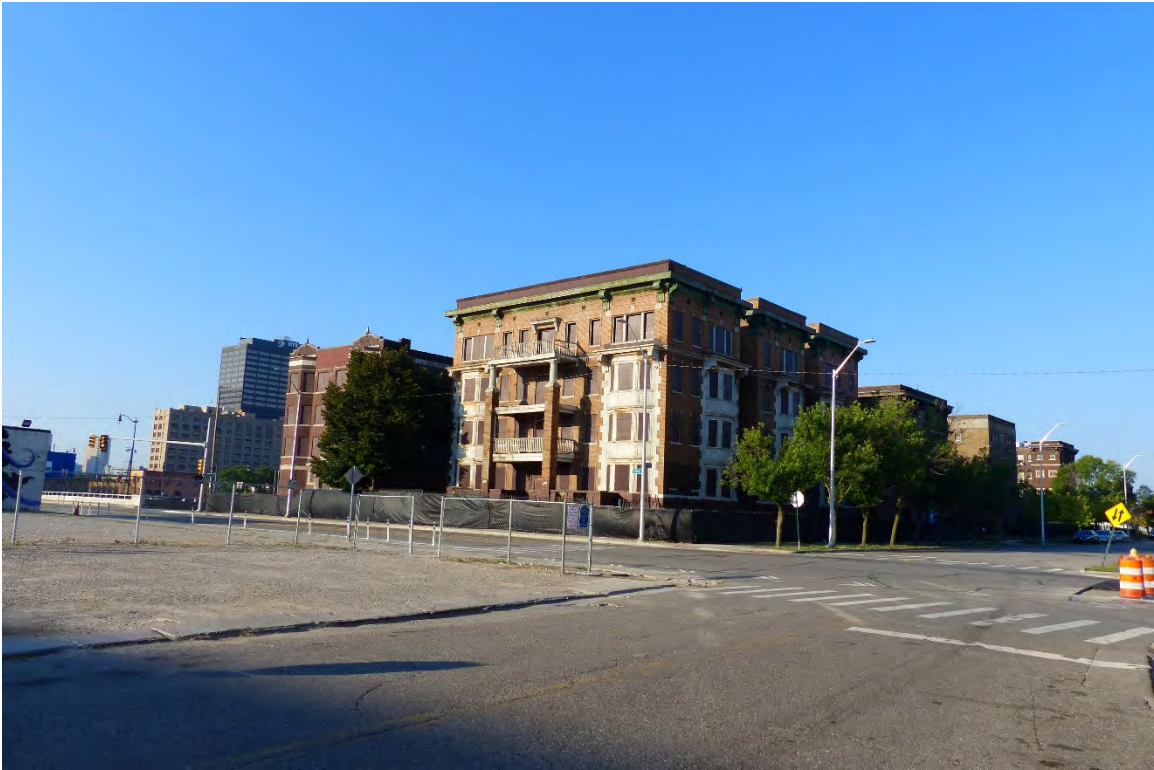
Figure #01: Exterior, Overall context, Looking Southwest. 08/23/20.
