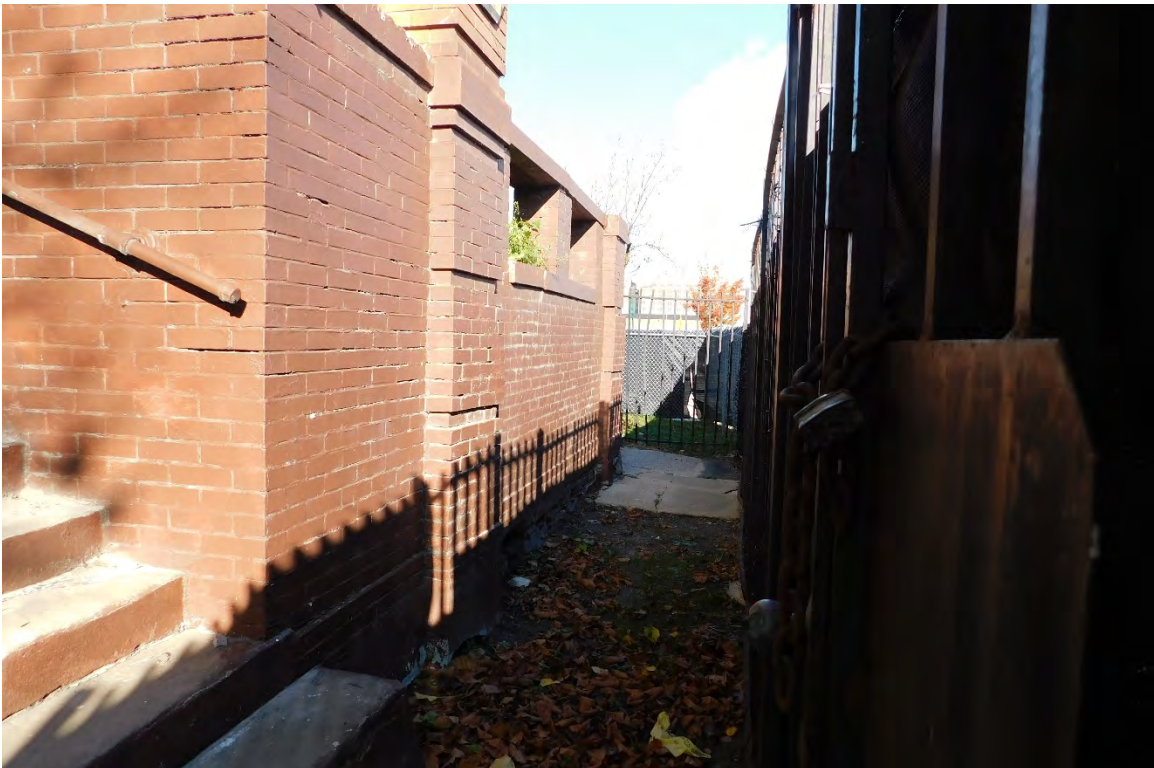
Figure #11: Exterior, East façade first floor masonry wall, Looking North, 10/28/20.
