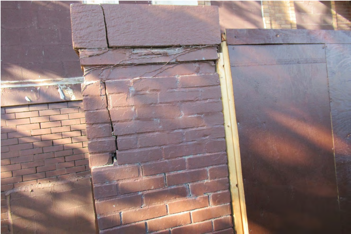
Figure #10: Exterior, East façade first floor masonry pier detail , Looking West, 10/28/20.
