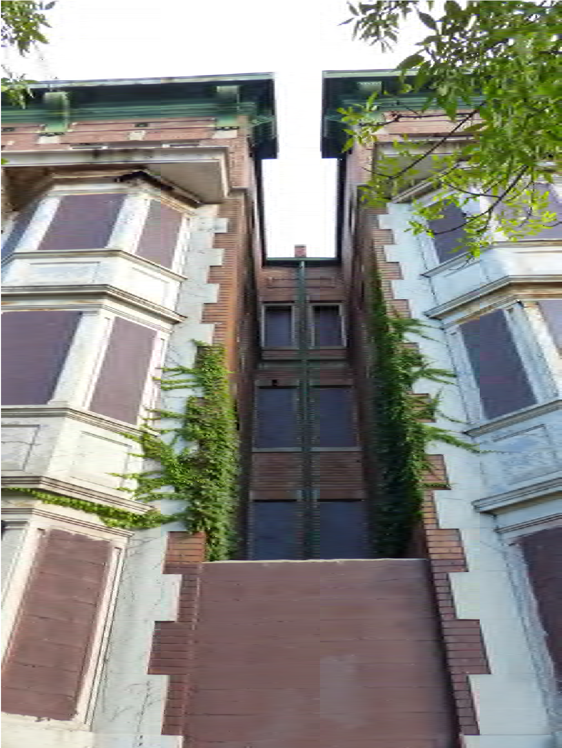
Figure #15: Exterior, North façade detail, Looking Up. 08/25/20.
