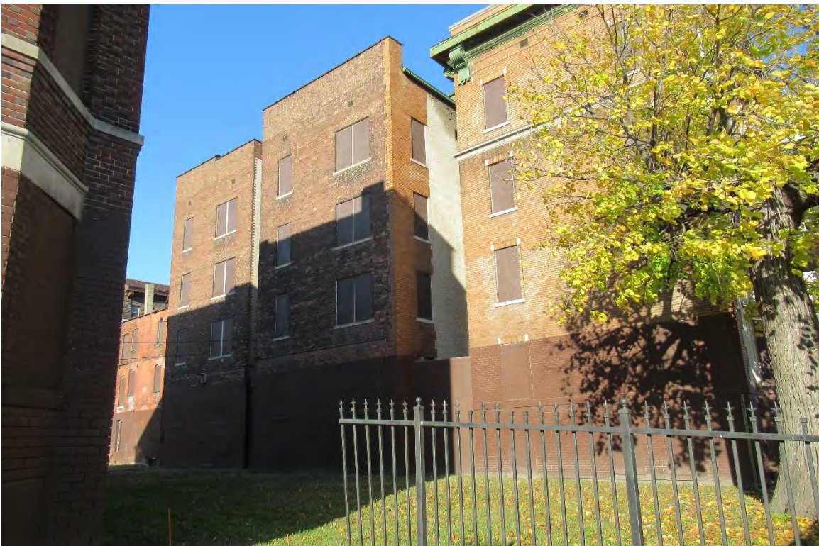
Figure #06: Exterior, South façade, Looking Northwest. 10/28/20.
