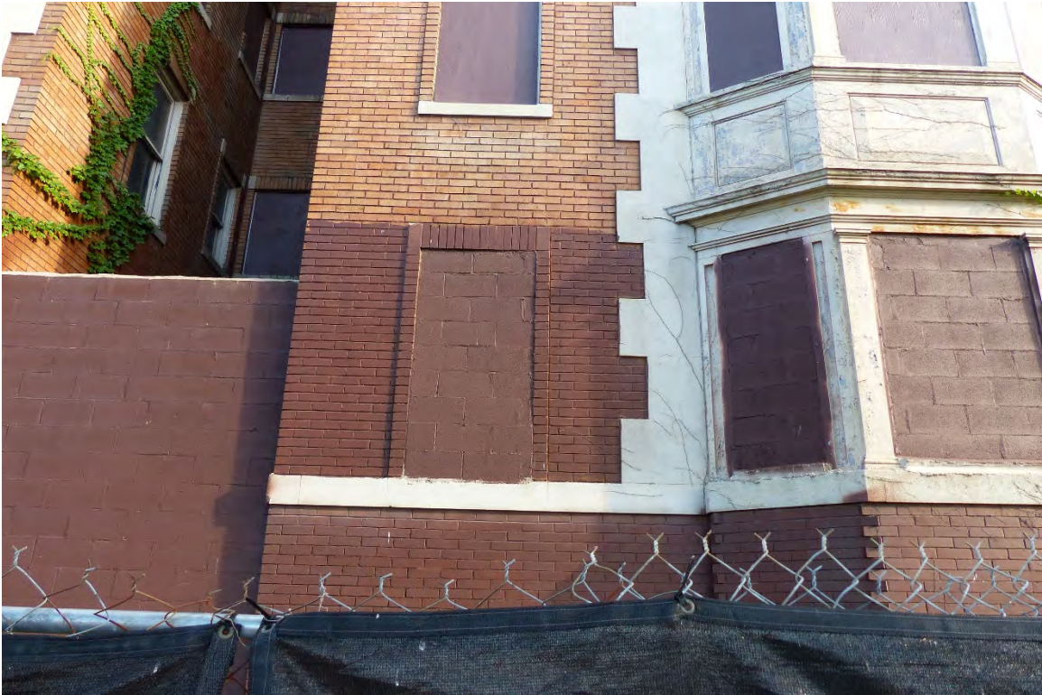
Figure #16: Exterior, North façade first floor masonry infilled opening detail, Looking South. 10/28/20.
