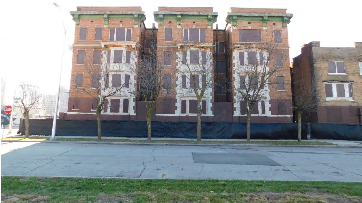
Figure #04: Exterior, North facade, Looking South. 10/28/20.
