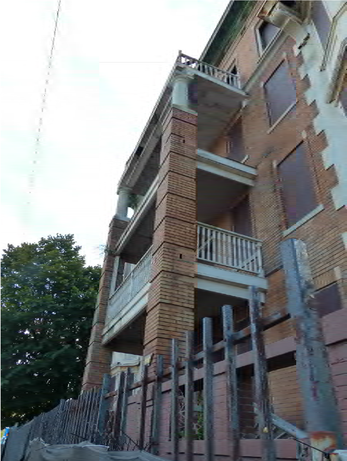
Figure #14: Exterior, East façade stacked porch detail, Looking Southeast, 10/28/20.
