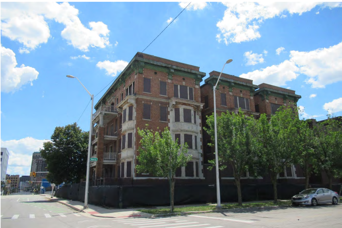
Figure #02: Exterior, Overall Context, Looking Southwest. 07/28/20.
