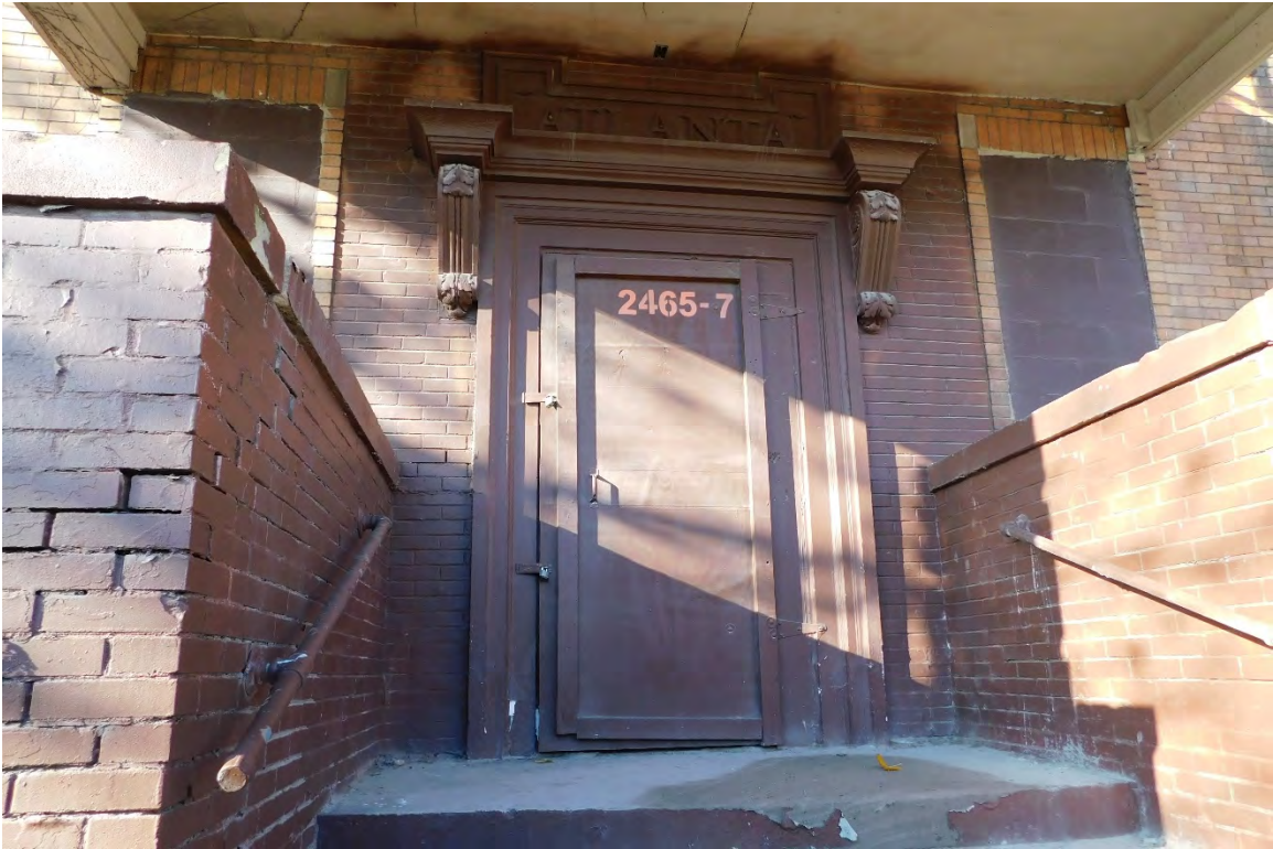
Figure #08: Exterior, East façade first floor main entrance detail, Looking West. 10/28/20.
