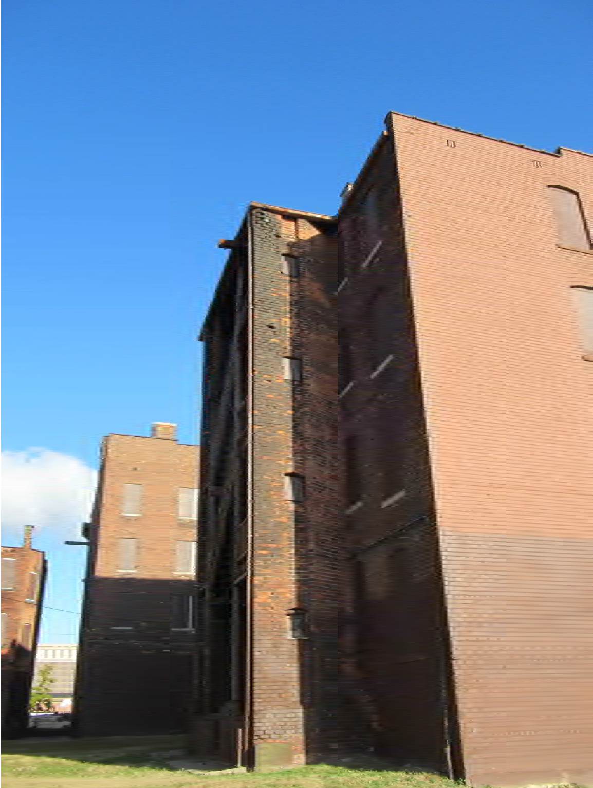
Figure #10: Exterior, West façade exterior stair enclosure detail, Looking North, 10/28/20.
