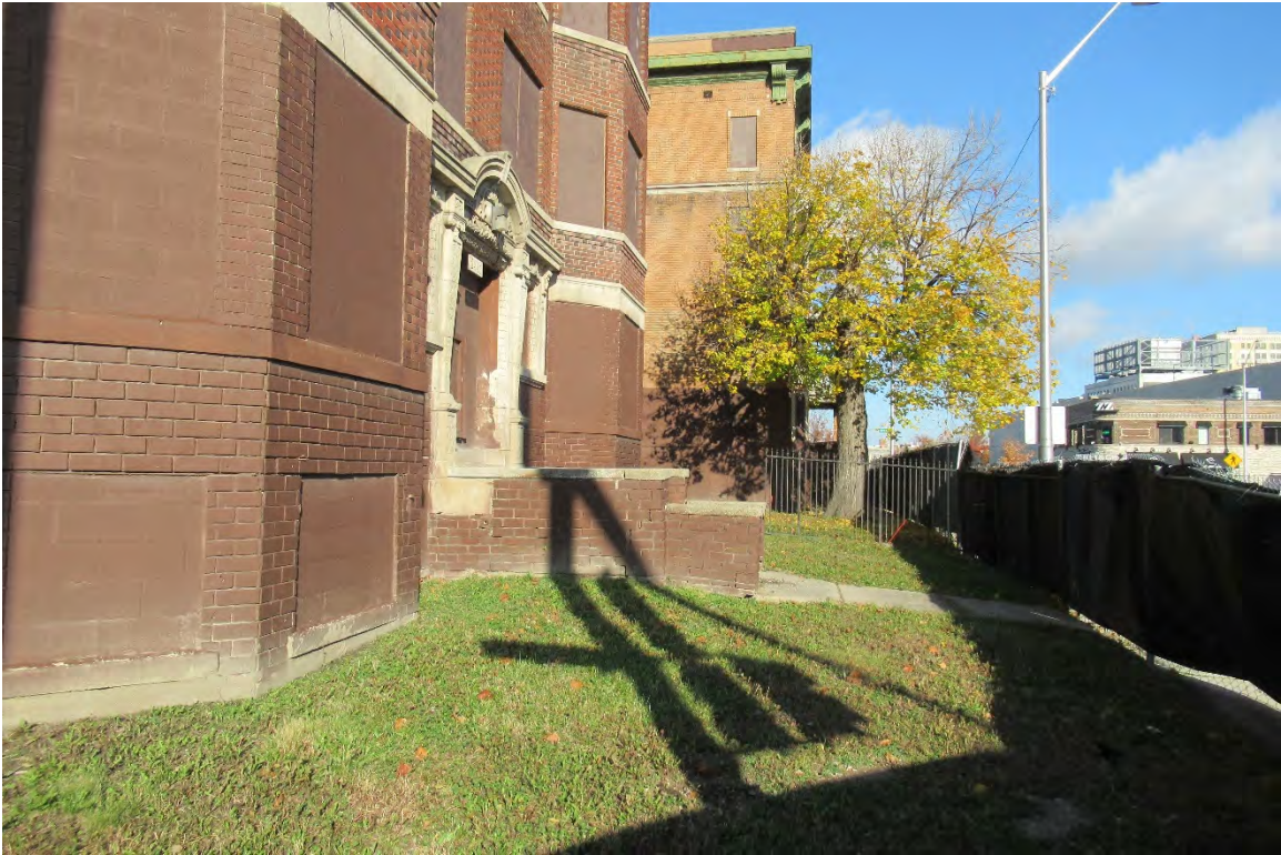
Figure #08: Exterior, East façade, Masonry infilled opening detail, Looking North. 10/28/20.
