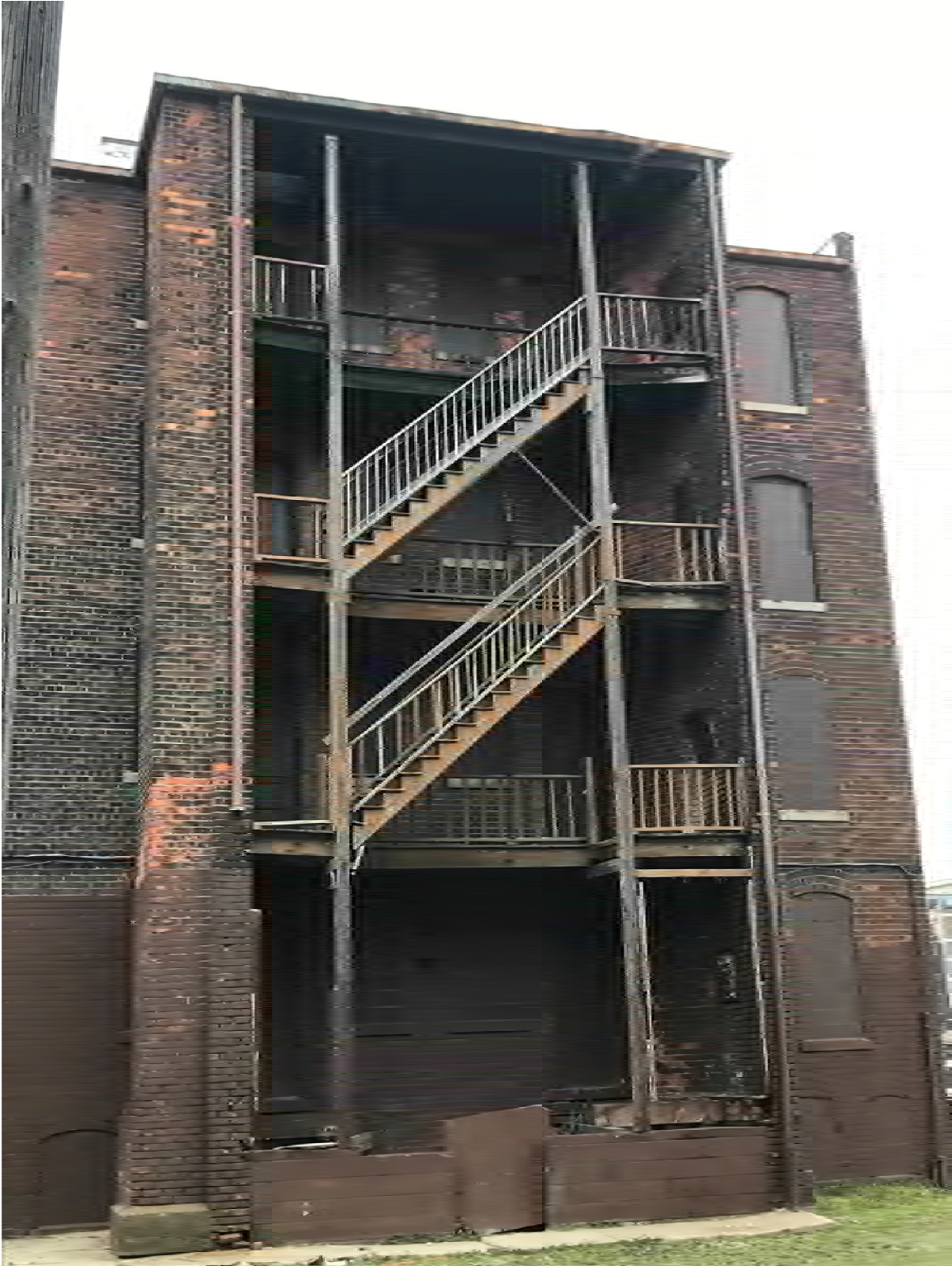
Figure #12: Exterior, West façade exterior stair detail, Looking East. 04/24/20.
