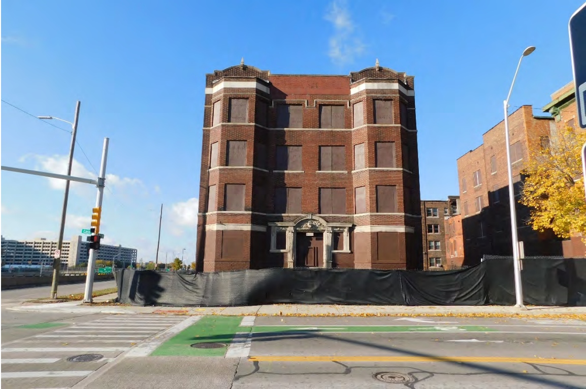
Figure #01: Exterior, East façade, Looking West. 10/28/20.
