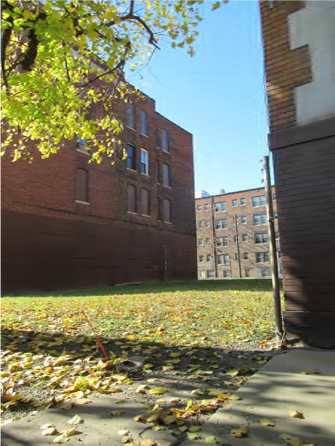
Figure #11: Exterior, North façade, Looking Southwest, 10/28/20.
