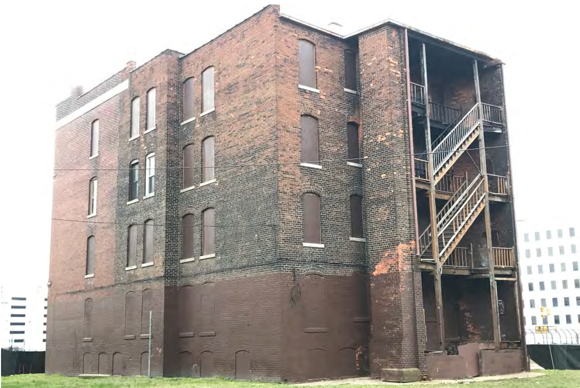
Figure #04: Exterior, North and West facades, Looking Southeast. 04/24/20.
