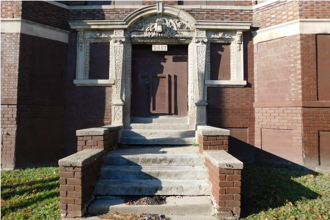
Figure #05: Exterior, East façade Main Entrance, Looking West. 10/28/20.
