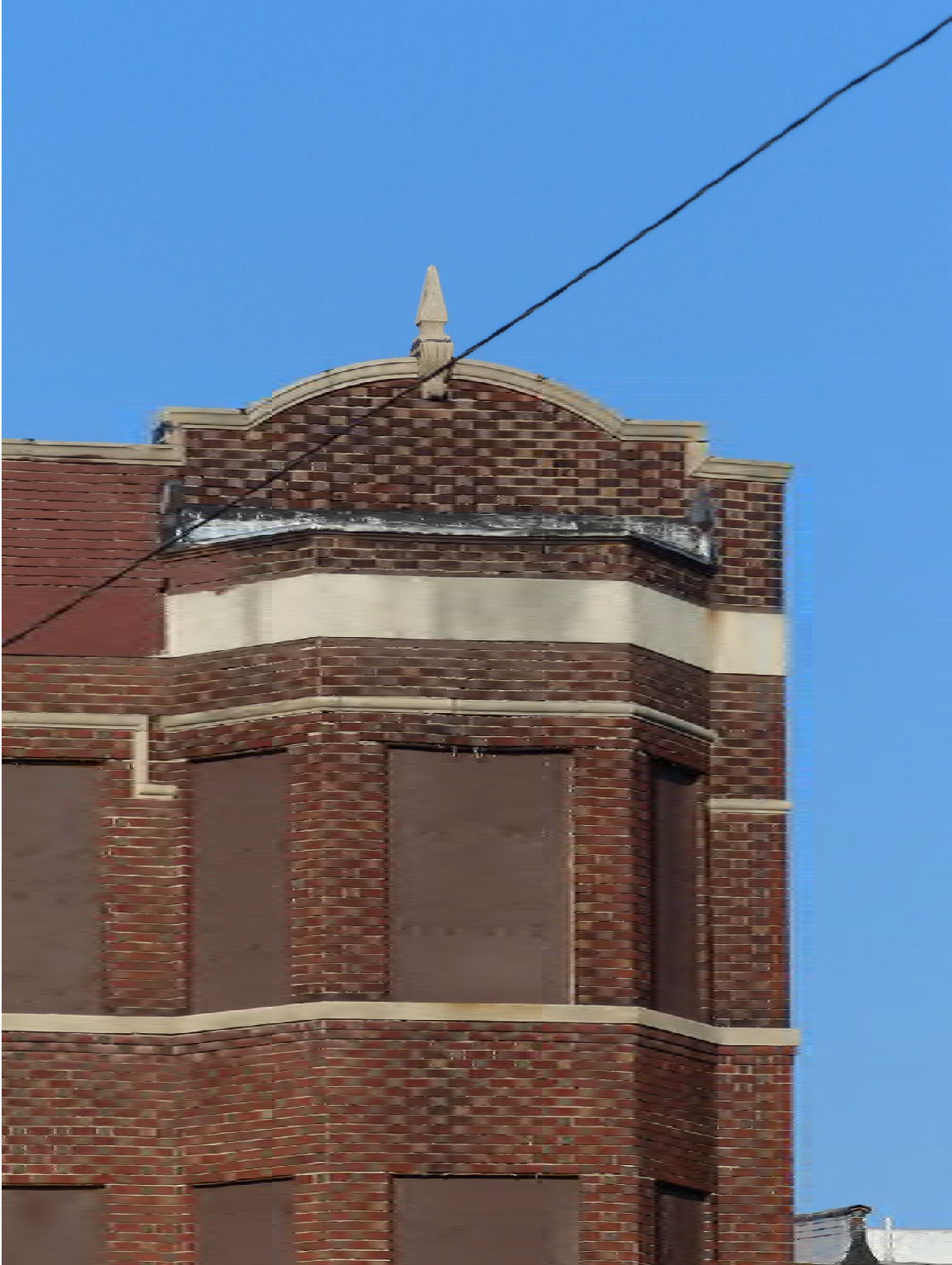
Figure #07: Exterior, East façade masonry and stone detail , Looking Up 10/28/20.
