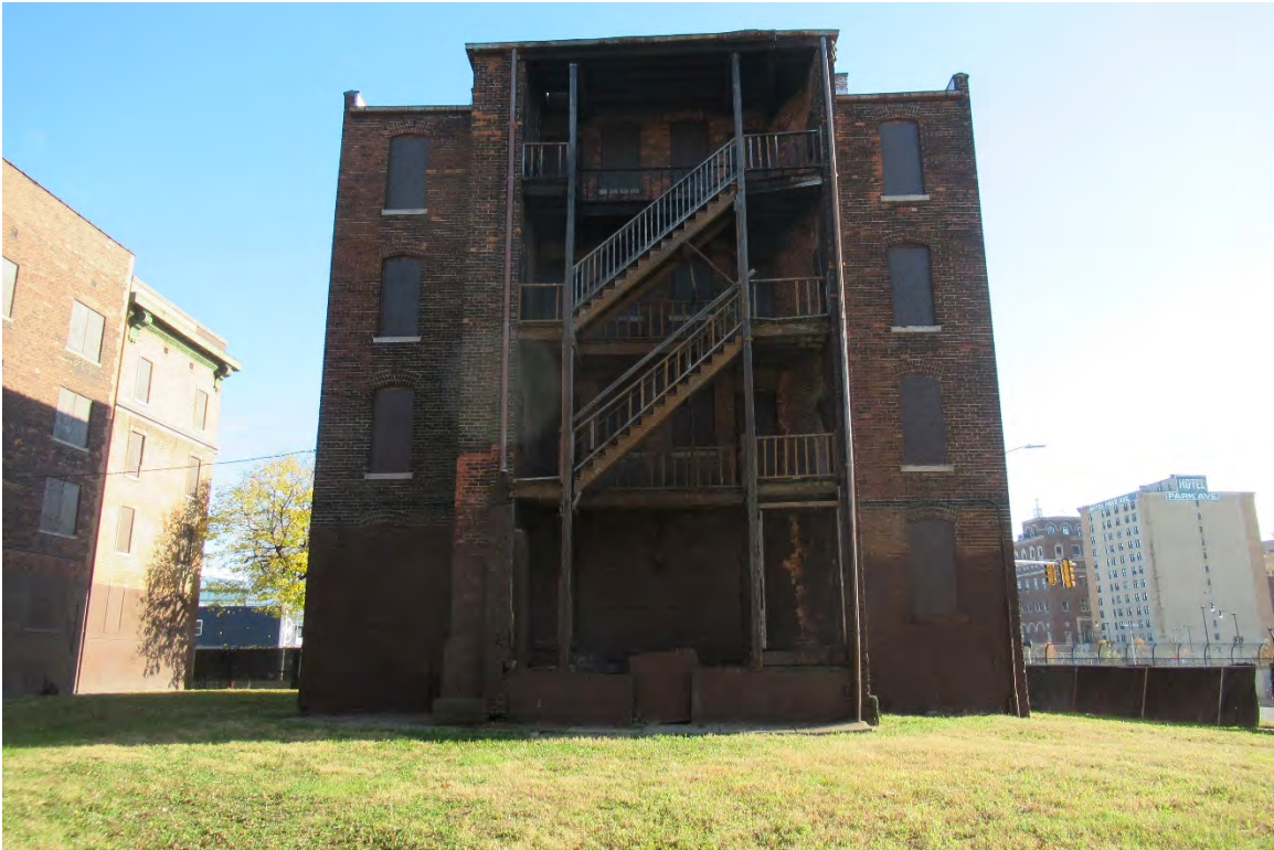
Figure #03: Exterior, West facade, Looking East. 10/28/20.
