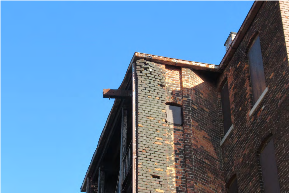
Figure #13: Exterior, West façade exterior stair enclosure masonry detail, Looking Up, 10/28/20.
