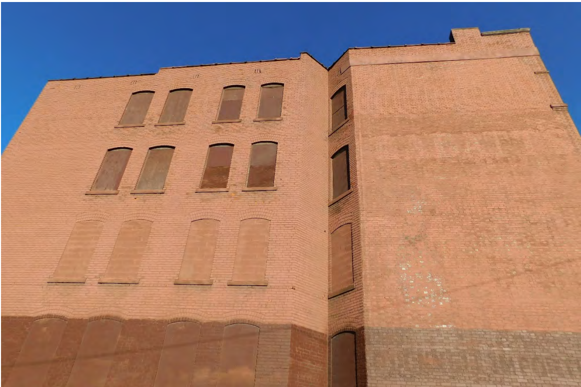
Figure #09: Exterior, South façade, Masonry detail, Looking Up. 10/28/20.
