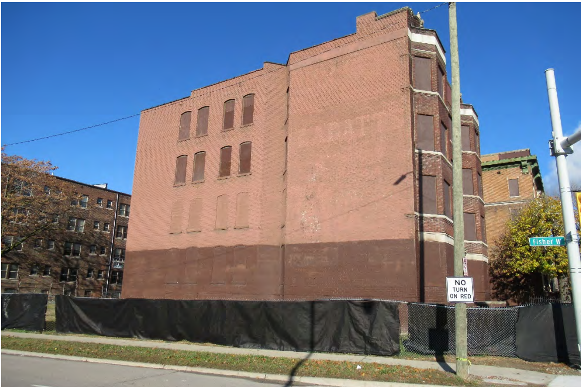
Figure #02: Exterior, South façade, Looking Northwest. 10/28/20.
