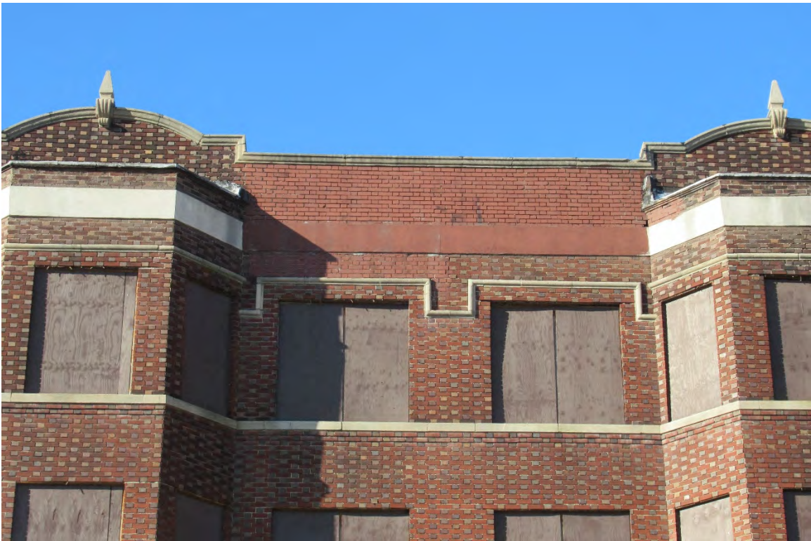
Figure #06: Exterior, East façade window and stone detail, Looking Up. 10/28/20.
