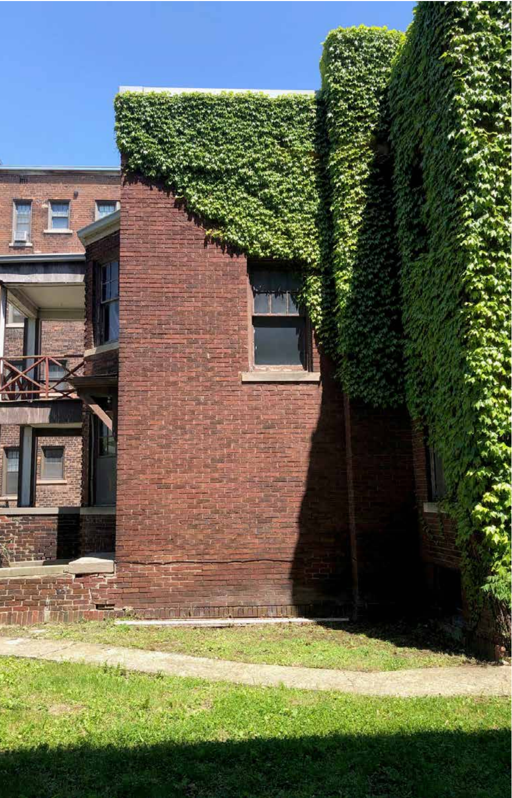
WEST FACADE (SIDE)
