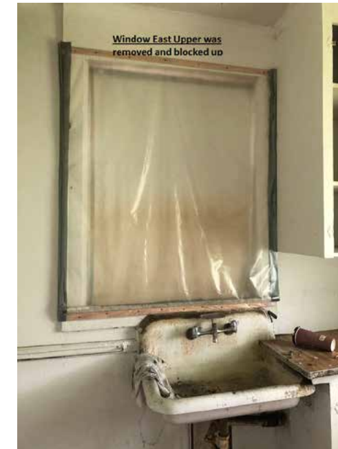
WINDOW S-13 INTERIOR
