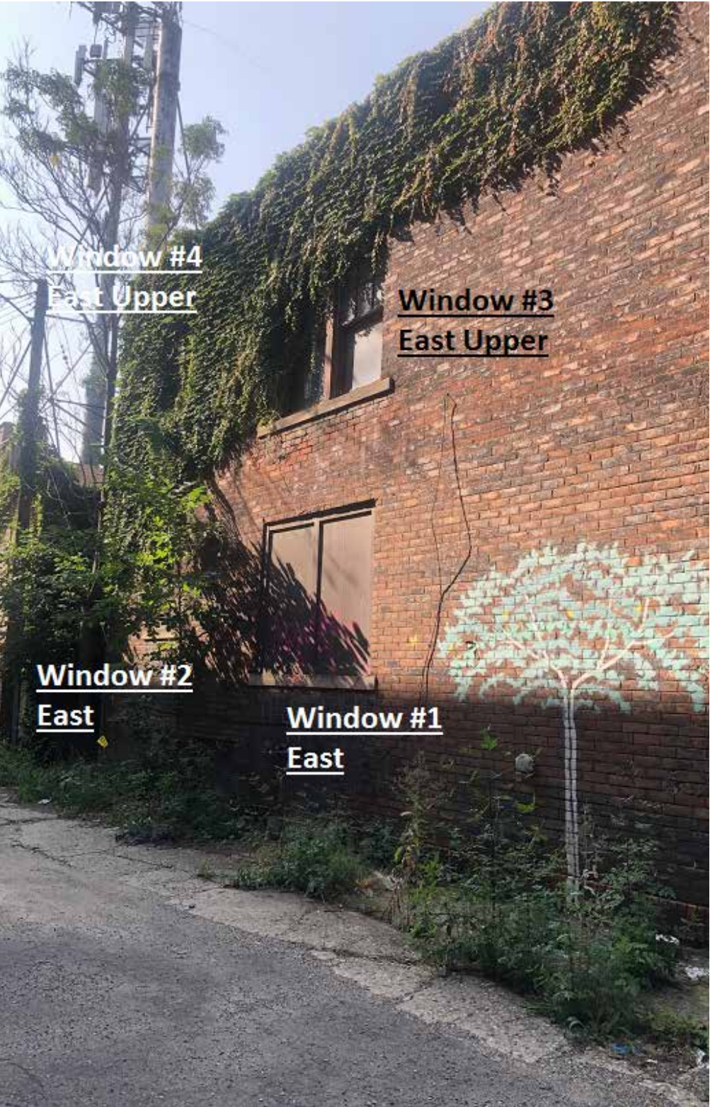
EAST FACADE (SIDE)
