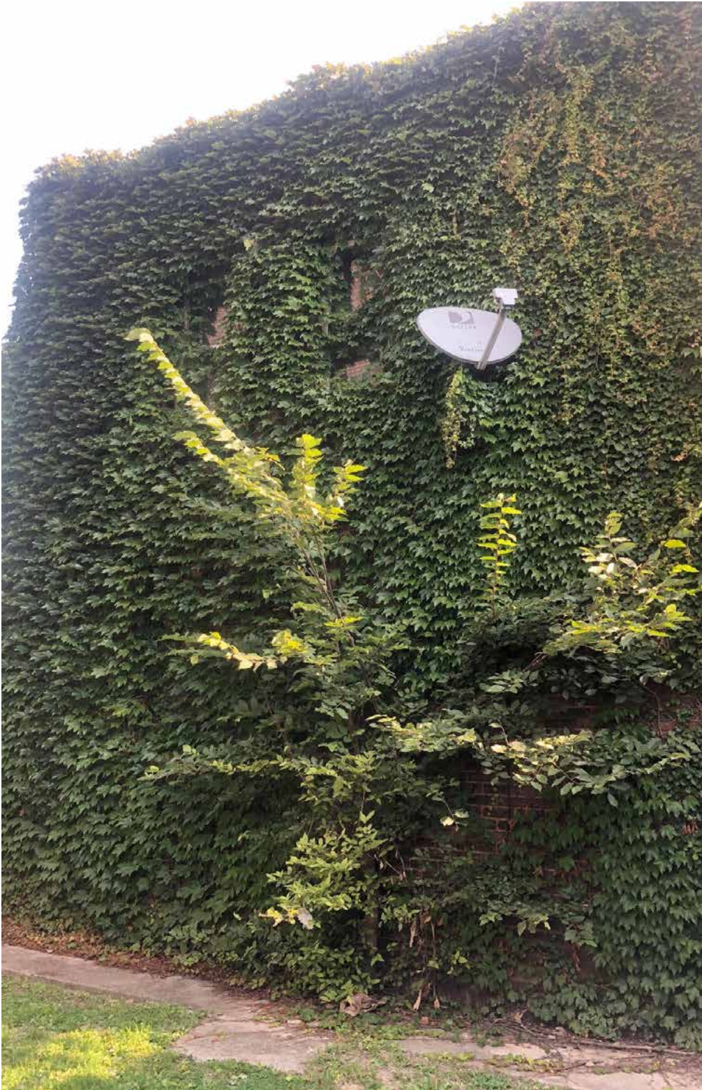
WEST FACADE (SIDE)
