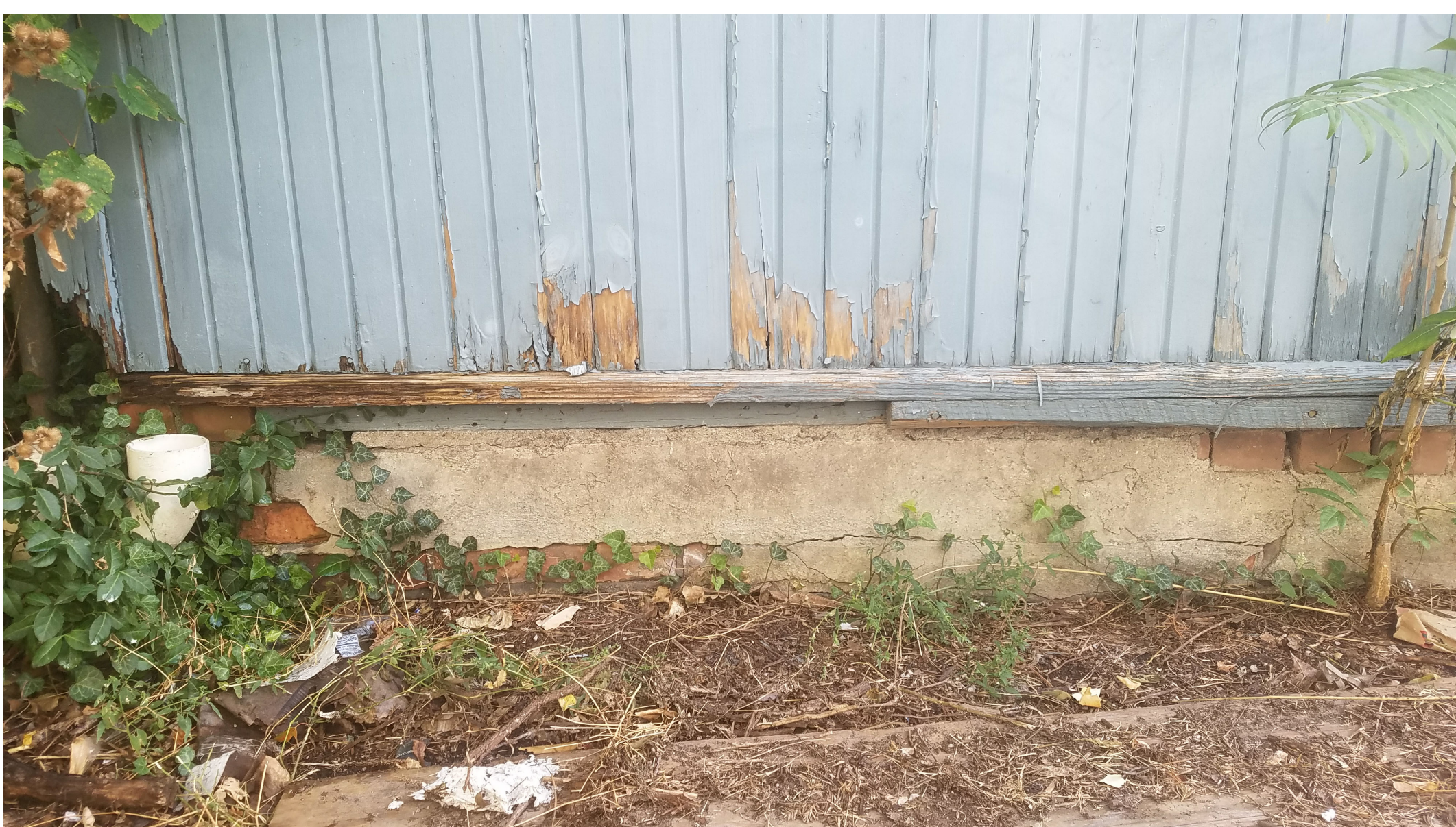
BASEMENT STAIR BRICK ENCLOSURE/FOUNDATION
