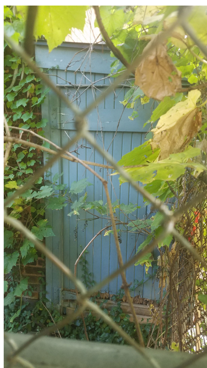
REAR ENTRY TO BASEMENT STAIR
