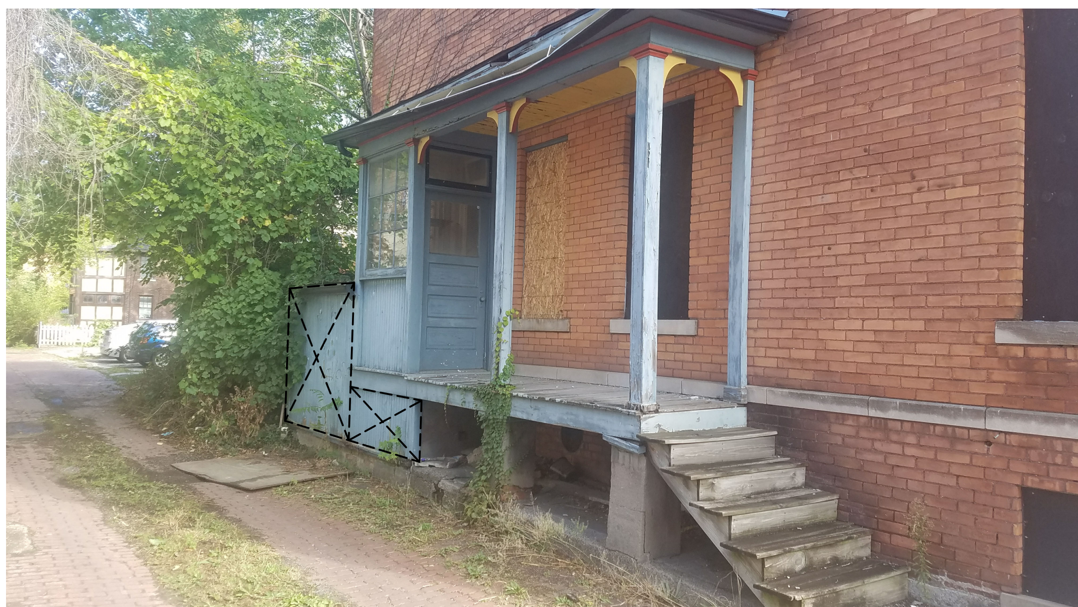
EXISTING PORCH AND BASEMENT STAIR ENCLOSURE (IDENTICAL ON BOTH SIDES OF THE BUILDING)
