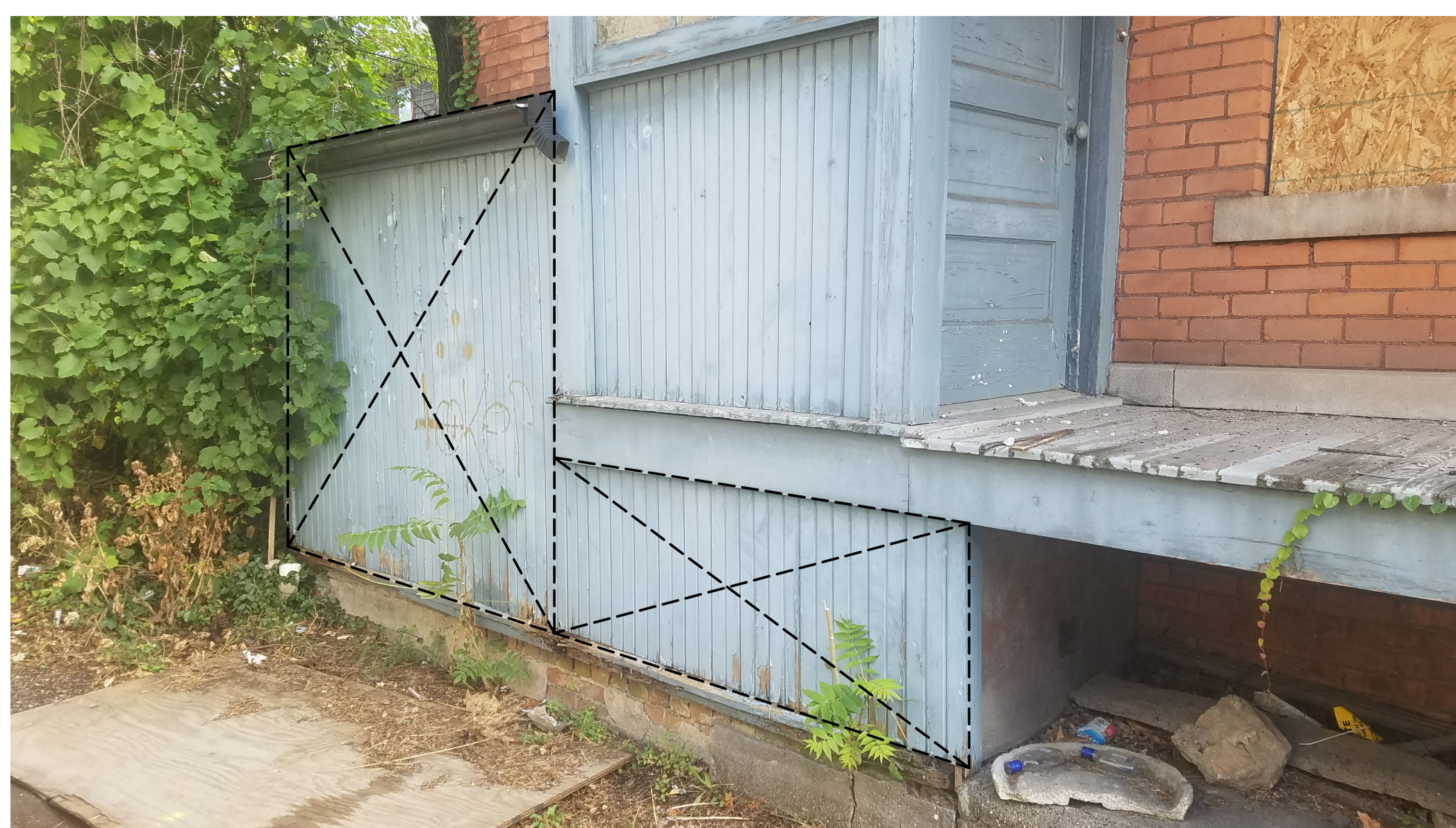
BASEMENT STAIR ENCLOSURE CLADDING TO BE REMOVED
