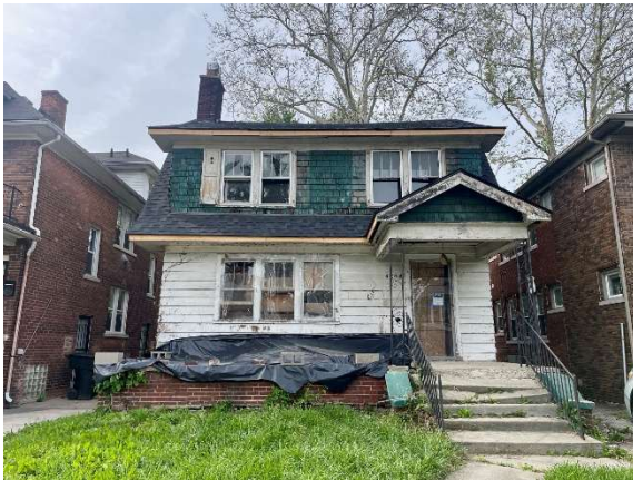
Staff photo, south elevation, 05-26-2026
