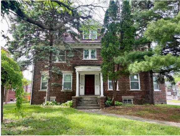
Staff photo, south elevation, 05-26-2026
