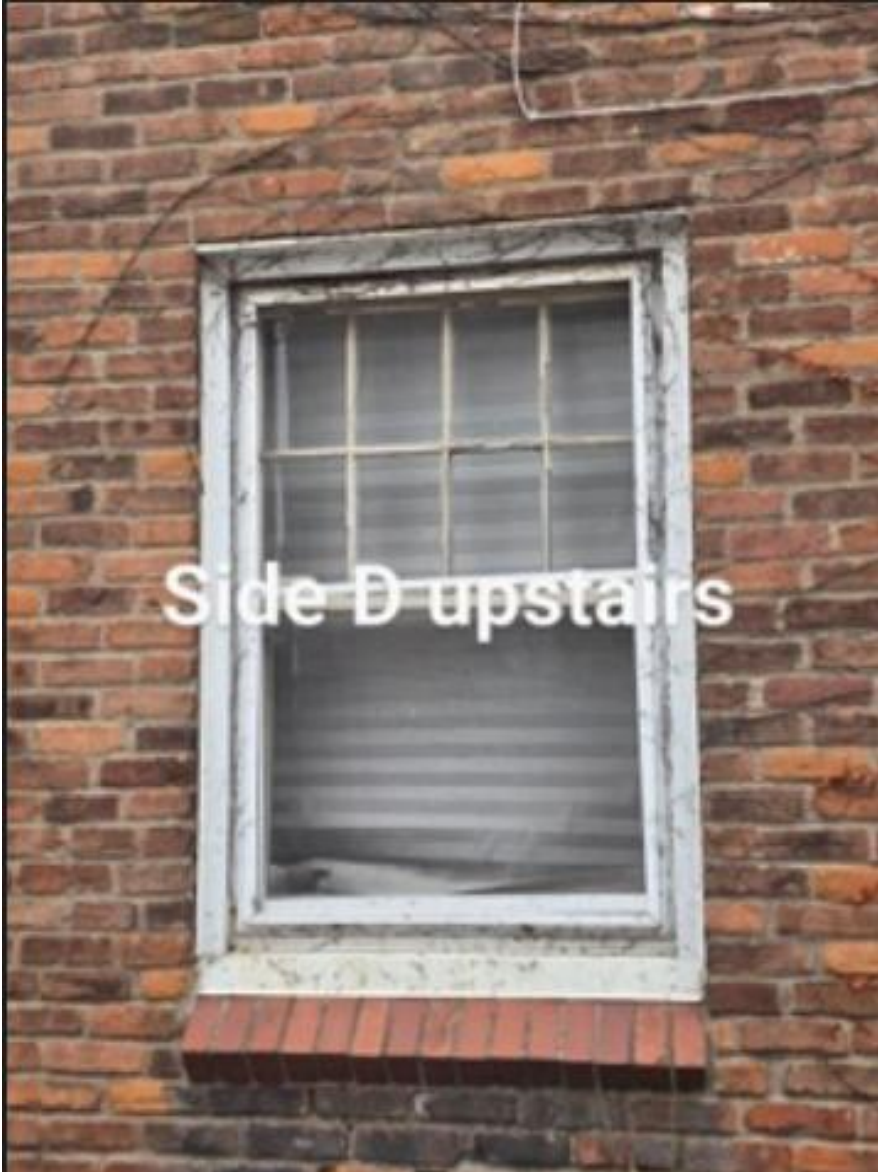
According to staff's window identification, this is either Window 13 or 14 .
