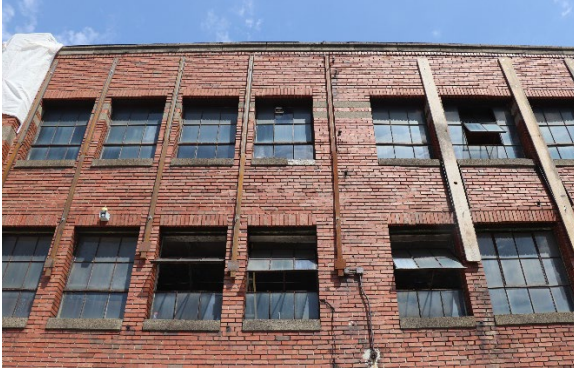
Staff photo, South-Facing Elevation, 04/22/26
