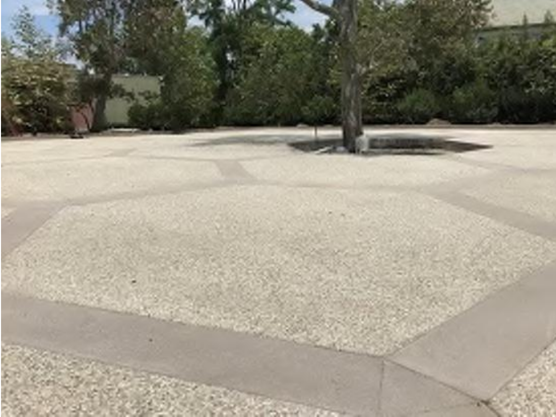
Proposed exposed aggregate concrete (sample) with limestone banding to replace the concrete and brick pavers around the octagon fountain.
