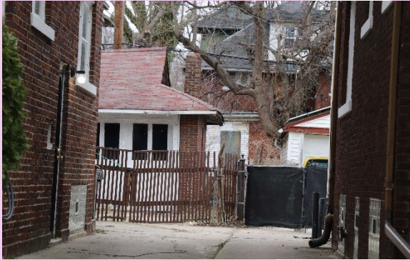
Staff photo, view of garage, 03/23/2026
