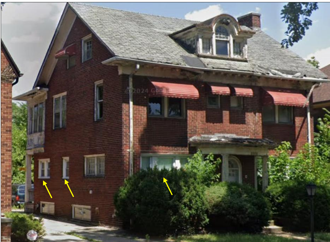
The above Google street view image of the front and west-side walls shows that most of the architectural details were still intact, however some replacement windows appear at the first floor, identified by the brightness of the window frames/trim and lack of division of glass. July 2022.
