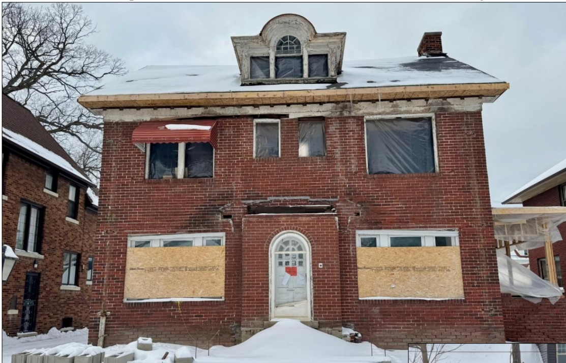
Above: Front wall of the house facing Longfellow.
