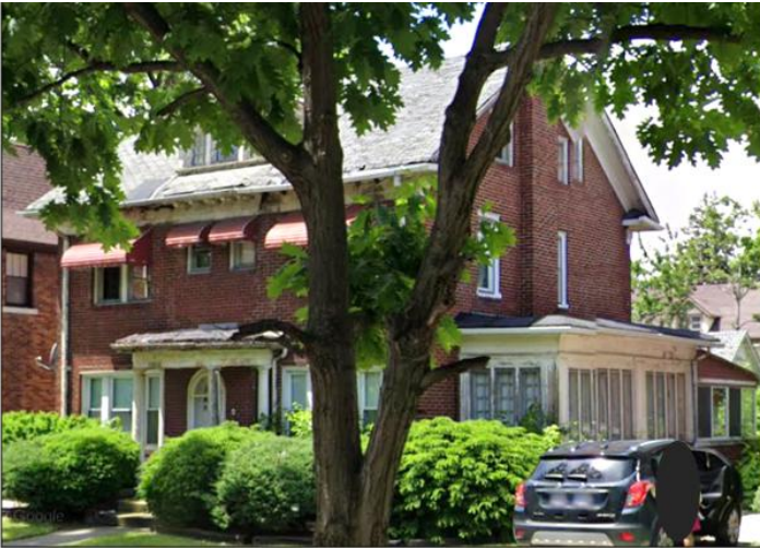
This Google street view confirms replacement windows were in place at both grouped window openings at the first floor and that the original side porch walls and windows remained intact. June 2019.
