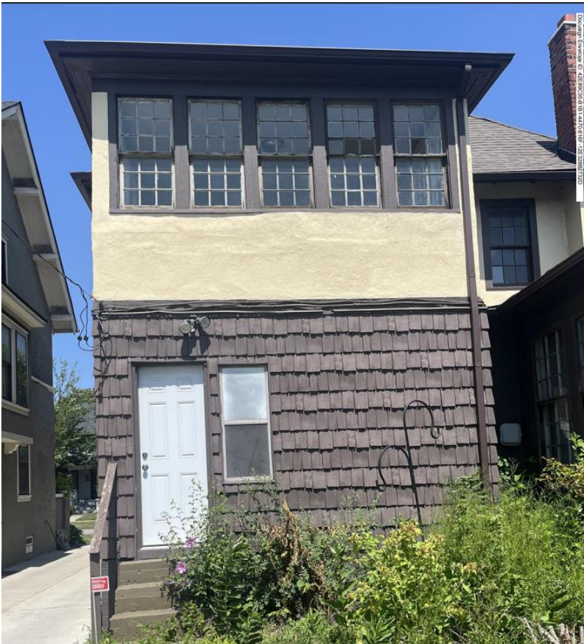
899 Edison, rear two-story wing to be demolished and rebuilt. Historic windows are to be preserved and reused. A new steel door is proposed to replace the existing steel door. The adjacent one-story rear wing to the east (sun parlor) is just visible to the right. (Photo from applicant's materials.)
