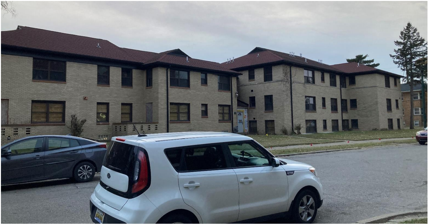
North side of 761 Whitmore, along Whitmore. The door centered here was replaced without approval and will be replaced with a rebuilt entry door that matches the historic design. The low porch walls toward the northeast corner are historic, character-defining features of the building. The chimneys that were visible in the designation photo have since been replaced with short, metal exhaust pipes. Air conditioning units and a 6-foot-high black fence are proposed along Whitmore. (Staff photo, November 2025)
