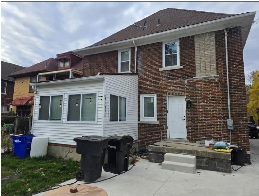
4325 Leslie, photo provided by applicant. Rear sunroom addition with new vinyl siding and new vinyl windows, new vinyl windows on the historic house, brick-infilled opening at second floor, and new back door are all pictured. (The infilled opening next to the new back door with reddish bricks has been infilled since at least 2011, so it is not part of this proposal or the violations process.)
