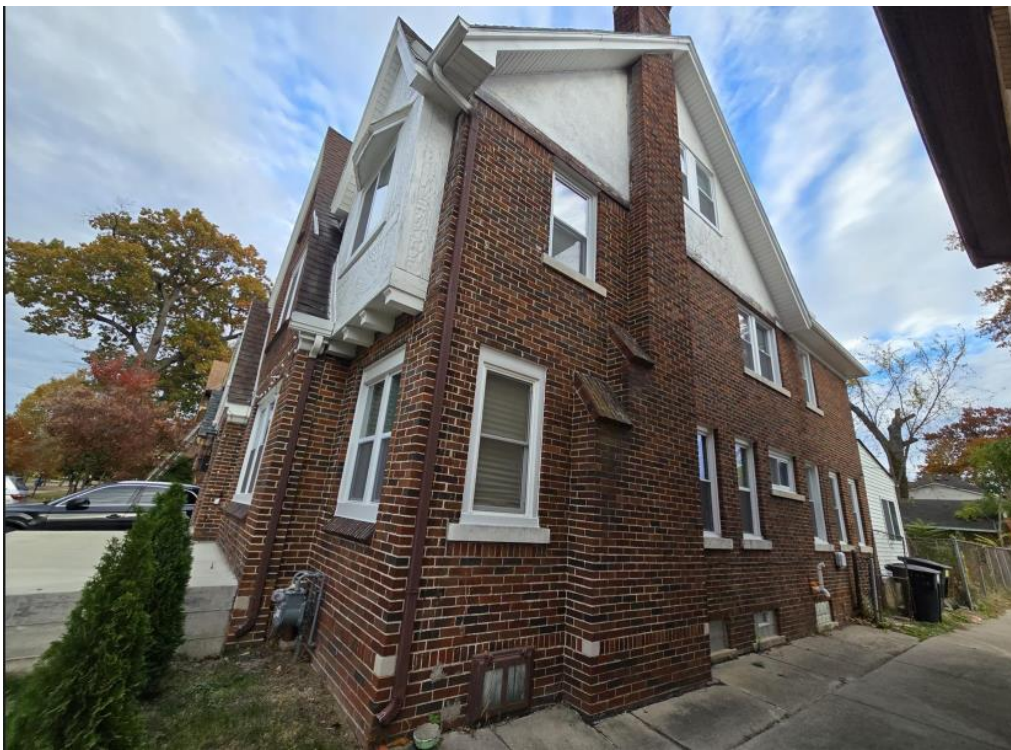
4325 Leslie, west side of house. Vinyl windows on side of house and vinyl windows and vinyl siding on rear sunroom addition are shown. Also visible are the white-painted half-timbering details on the front of the house, near the northwest corner. (Applicant's photo from materials.).
