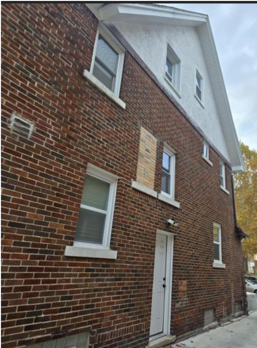
4325 Leslie, east side, photo provided by applicant. Vinyl windows, infilled window opening, and new side door are all visible.
