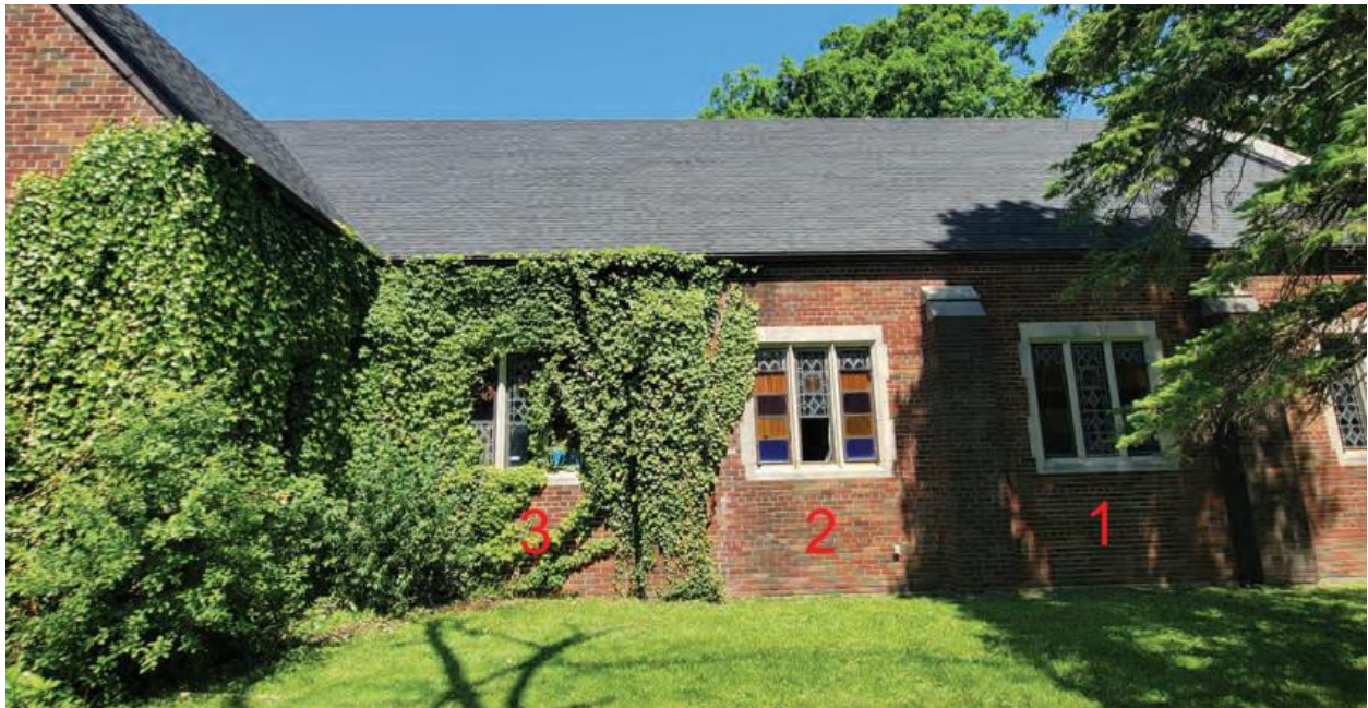
South wall, casement windows at openings 1-3 proposed for replacement. Annotated photo by applicant
