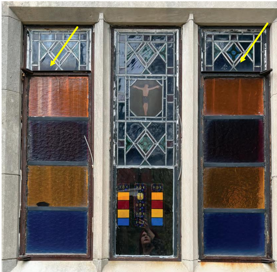
Photo provided by applicant. Note that the transoms panes appear to be slightly more inset within the opening than the operable sash. Staff notes that the submitted drawings do not provide dimensions of the top portion of the existing casement window frame (see yellow arrows).
