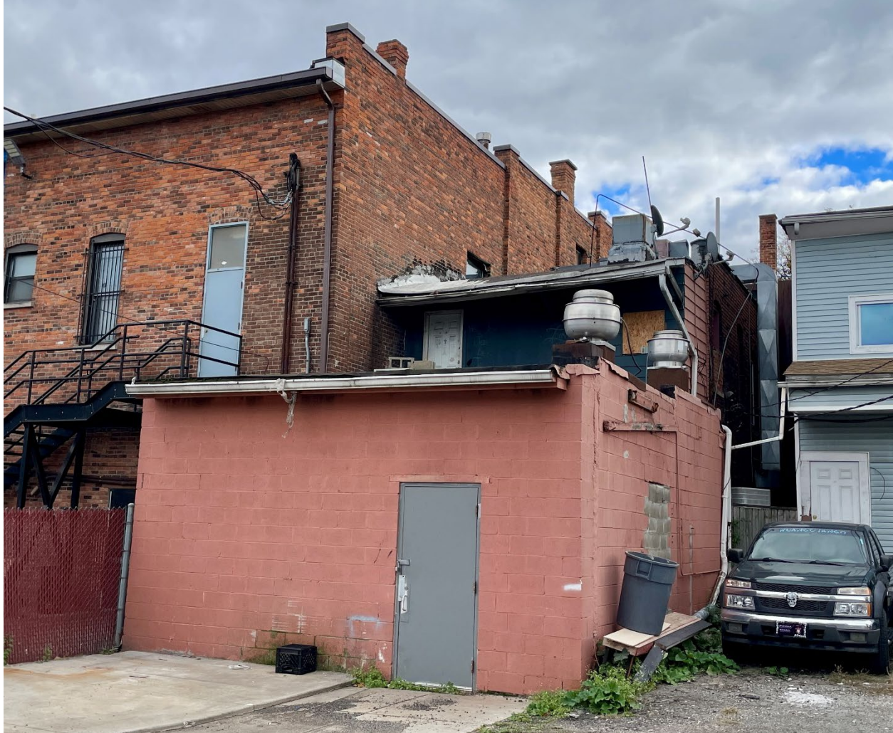
Staff photo, 10/24/2025. Rear of the building, taken from the alleyway to the North of the building.
