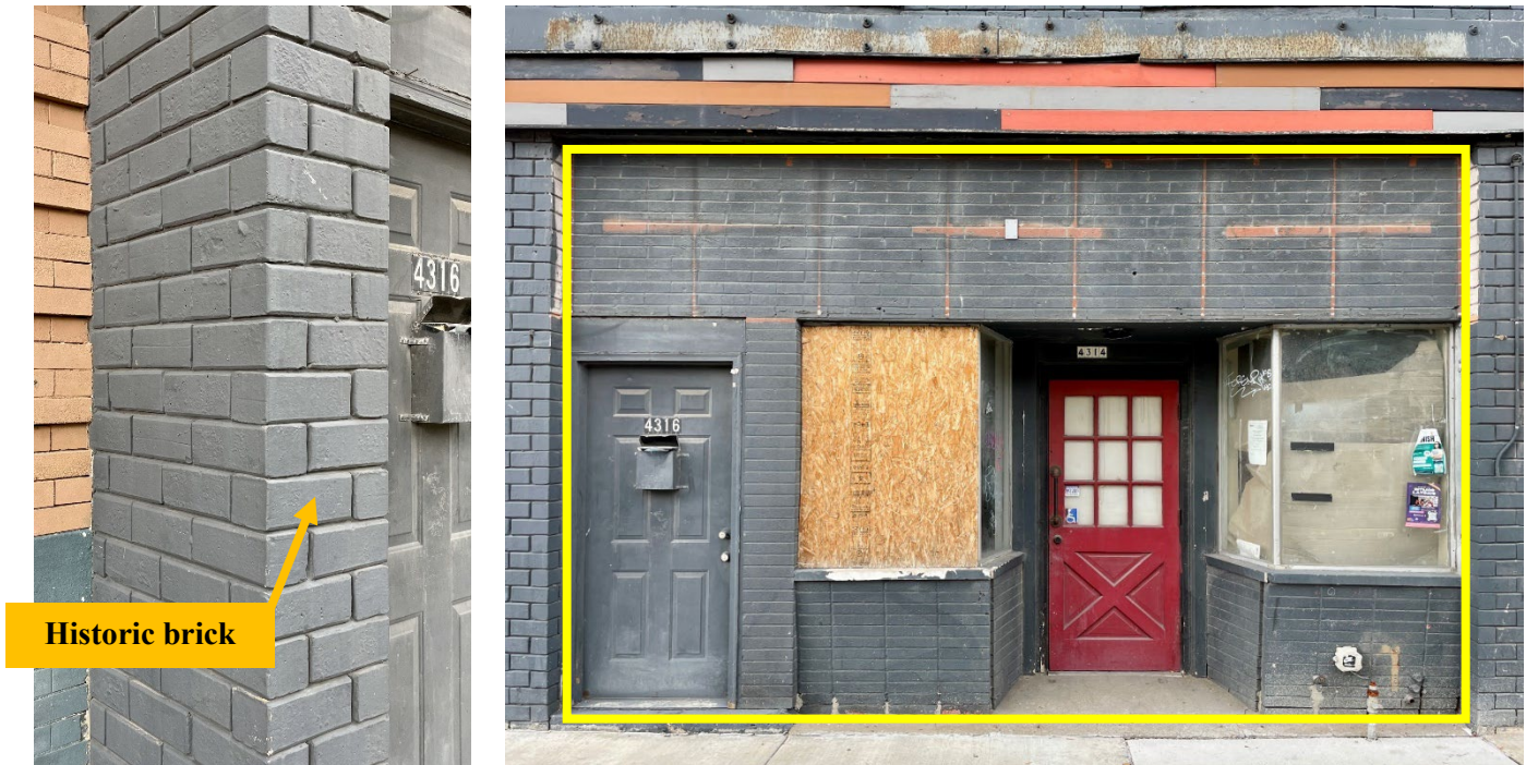
Staff photos, 10/24/2025. No elements within the yellow box are historic.
