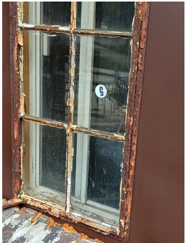
Photos provided by applicant, show the historic steel casement window with significant rust and peeling paint on the trim and muntins
