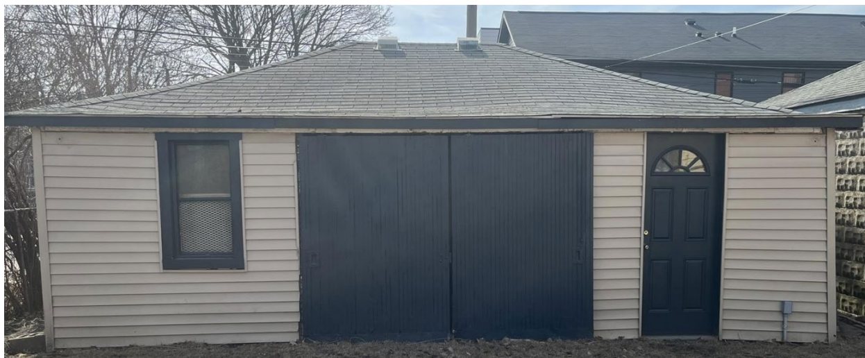
1613 Leverette garage, current appearance. Side facing the rear of the house, not visible from the alley. Photo provided by the applicant.
