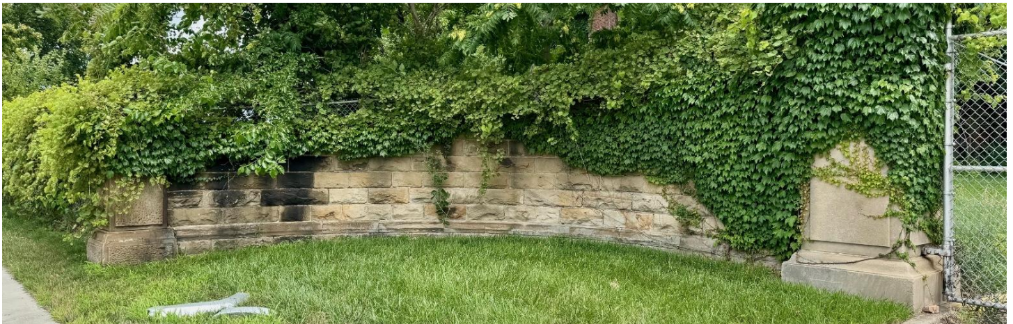
West side wall. Staff photo, July 17, 2025
