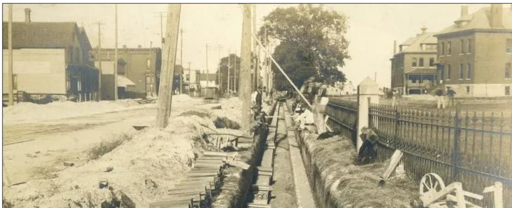
This 1898 photo is looking east down West Jefferson. A trench has been dug, and the street's first electrical conduit is being installed. The position of this picture is about half-way between the fort's east and west entrances. The wooden fence (visible in the 1861 photo of the east entrance) has been replaced with a wrought iron fence and obelisk-shaped concrete or stone posts. The two barracks buildings visible within the fort are on Cram, just south of the east entrance (both of which are shown in the 1974 image on the previous page).
