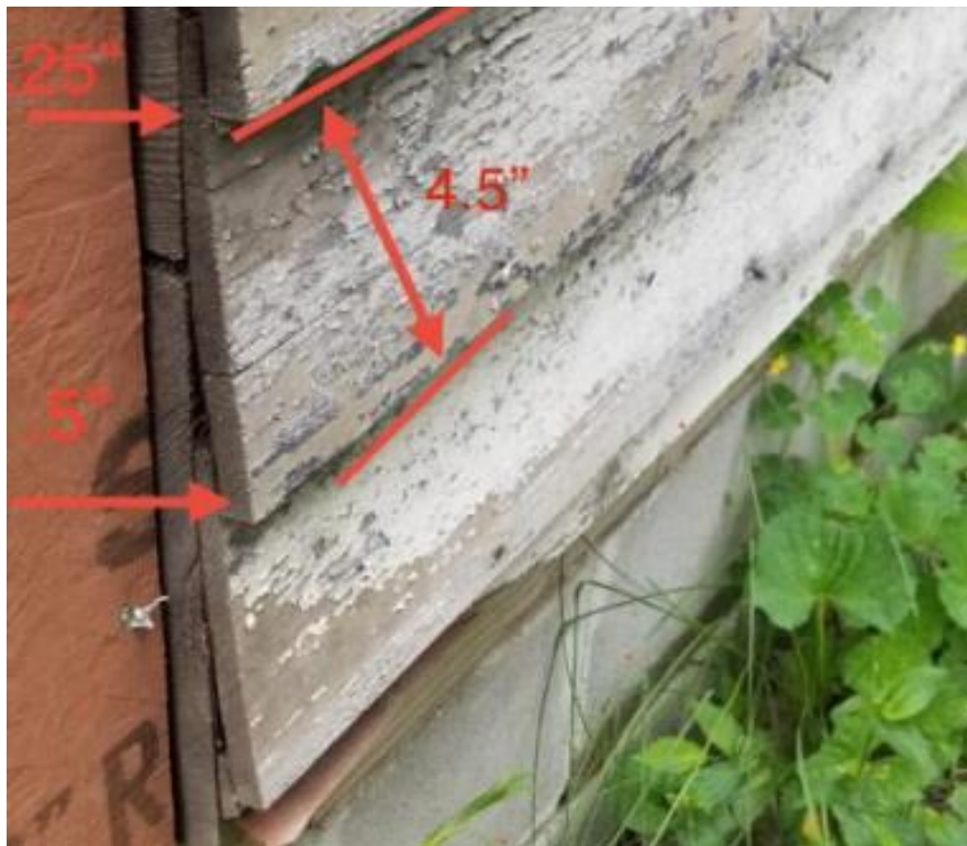
Detail, showing extant historic lapped wood siding at east/side wall. Dimensions noted in red. Image by applicant.
