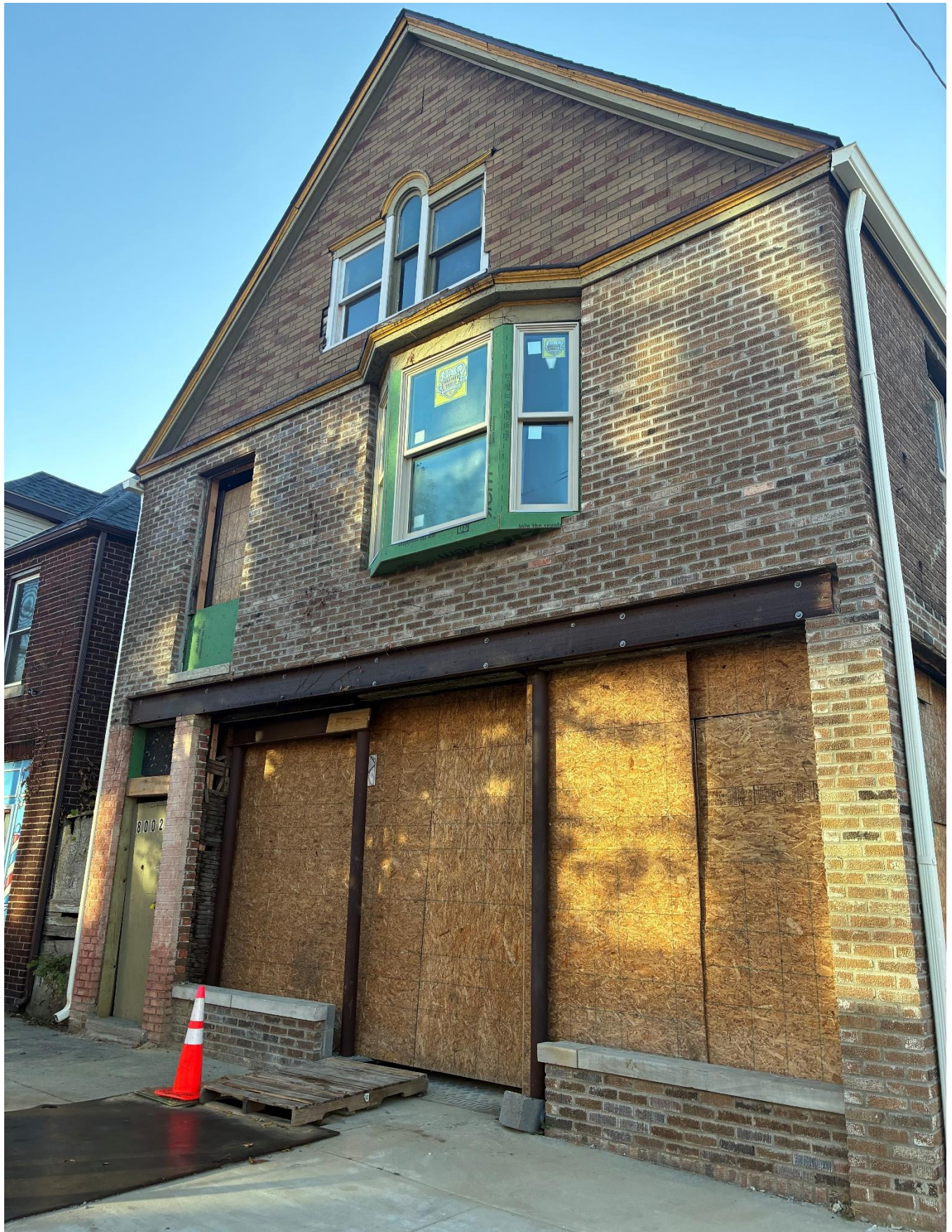
8002 Kercheval, front facade. Showing brick veneer at first and second stories. Asphalt/Insulbrick siding is present at the third-story gable end. Current condition. Photo by HDC staff, 10/27/2025.
