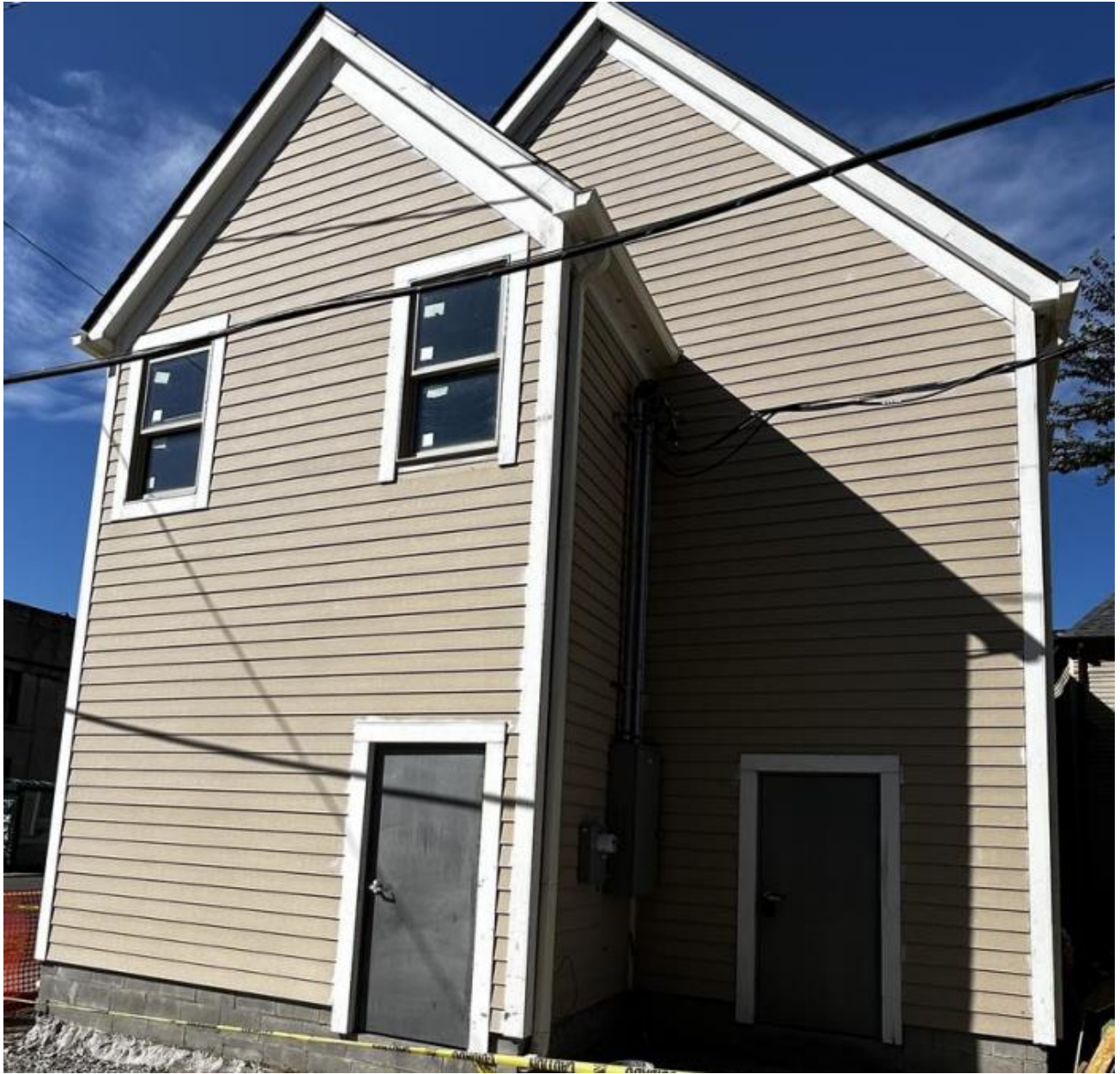
Rear addition, erected ca. 2021 showing extant composite/Smartside LP siding, installed in violation and latter approved by the Commission. Photo by applicant.
