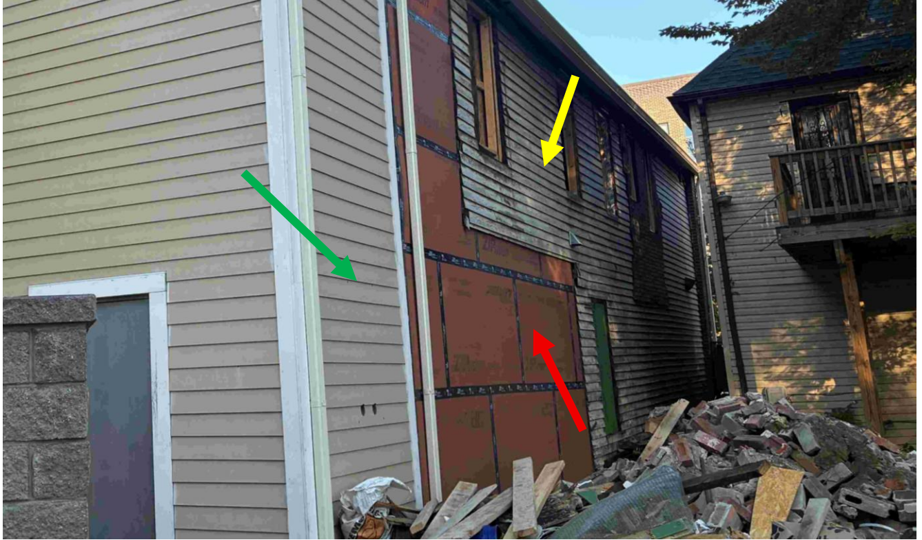
8002 Kercheval, east/side elevation. Showing historic wood siding (yellow arrow) which was revealed when Insulbrick/asphalt siding was removed ca. 2021; Zip sheathing, installed ca. 2021 (red arrow); and composite/Smartside LP siding installed ca. 2021 (green arrow) when rear addition was erected. Current condition. Photo by HDC staff, 10/27/2025.
