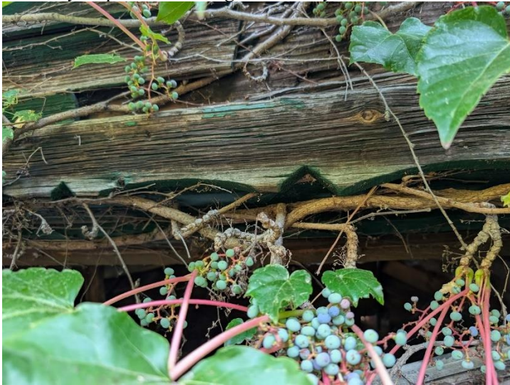
3768 Tyler, garage, west side, detail of scalloped trim below the gable roof and above the overhead doors. This kind of trim is typically found at primary elevations of midcentury garages. (Staff site visit, September 2025)
