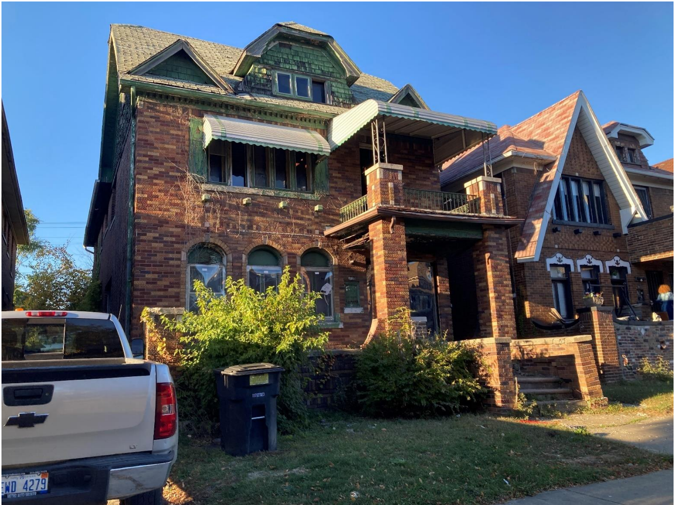
3768 Tyler, south end and some of the west side. The decorative curved brickwork at the front edge of the front porch originally had cast stone coping and the iron guardrail was installed between these curved features. Staff photo, October 2025.
