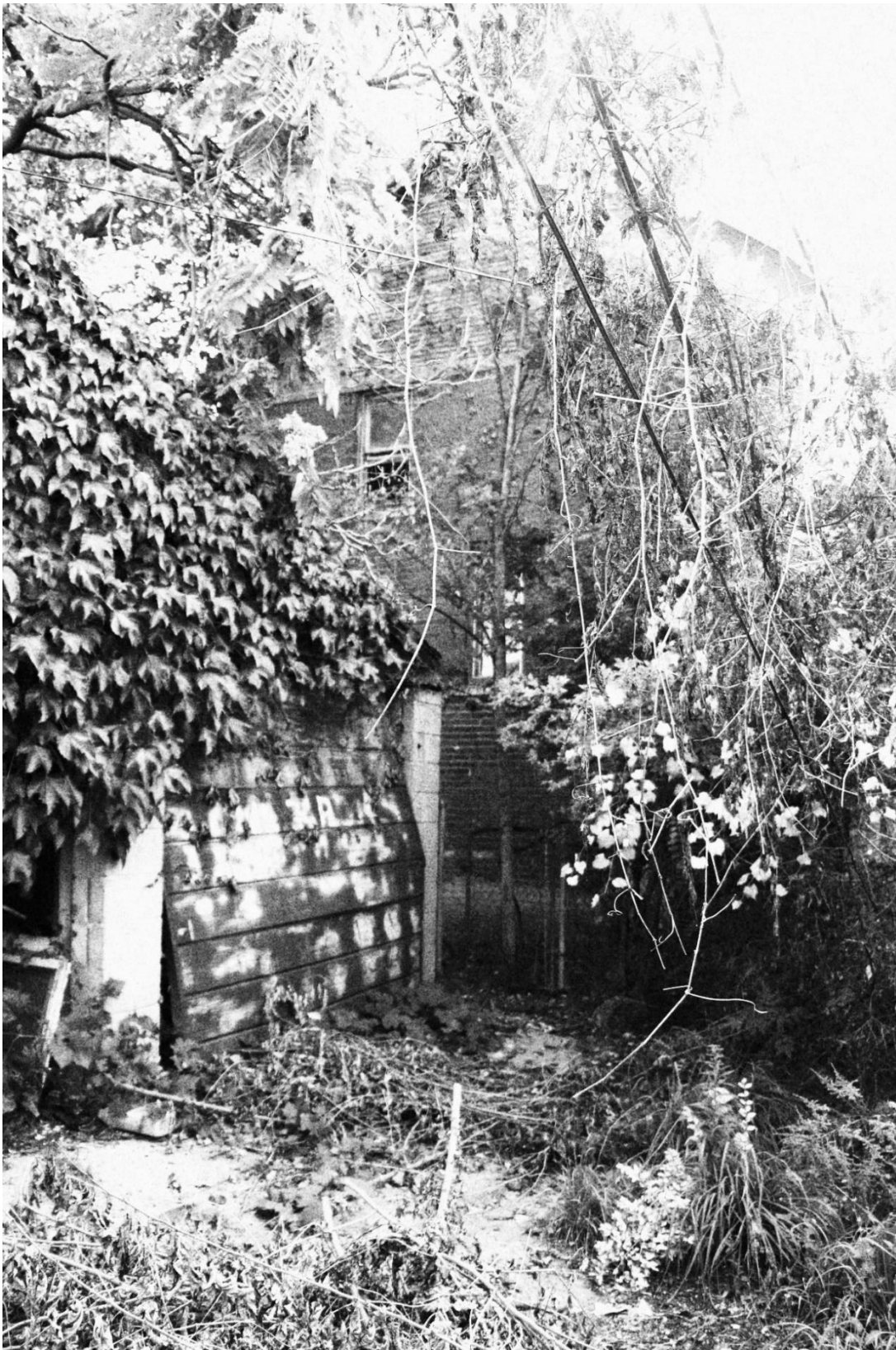
3768 Tyler, garage, southern portion of the west side shown, along with the overgrowth and state of driveway/pad adjacent to the alley. An overall photo of the garage was difficult, even for staff, given the extreme overgrowth around the structure. (Staff site visit photo, October 2025)
