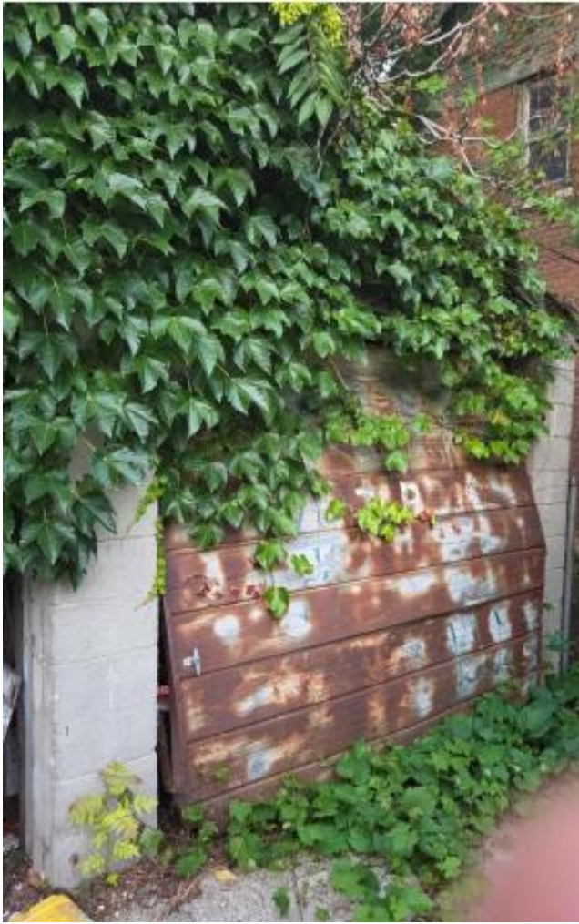
3768 Tyler, garage, west side near southwest corner, applicant-provided photo from materials. This door was also shown in the 2006 aerial photo. These overhead doors on the garage's west side open onto a concrete driveway or pad connecting to the alley.
