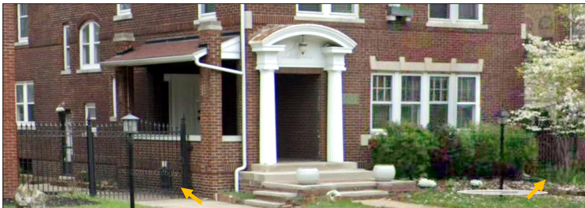
The jalousie windows and front door/sidelights were removed by 2019. Google streetview.
