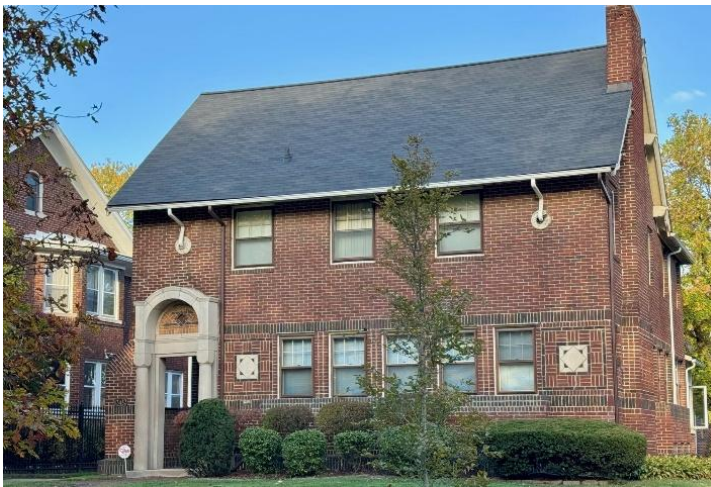
Adjacent house to the south of 3460 (3452 Iroquois).
