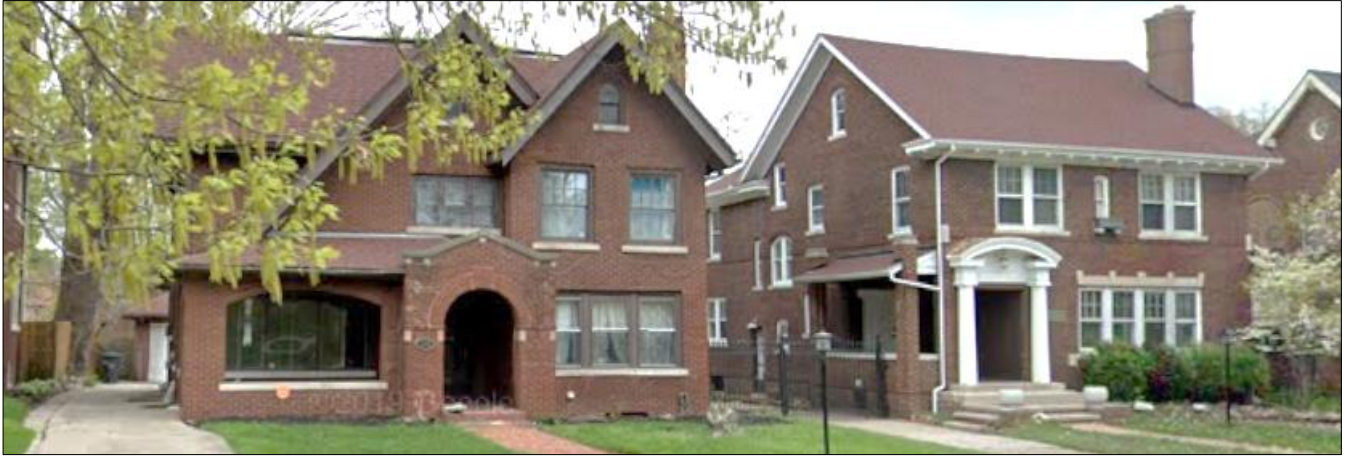
Adjacent house to the north (3470 Iroquois) with front-facing open porch and arched entry. Google streetview, 2019.
