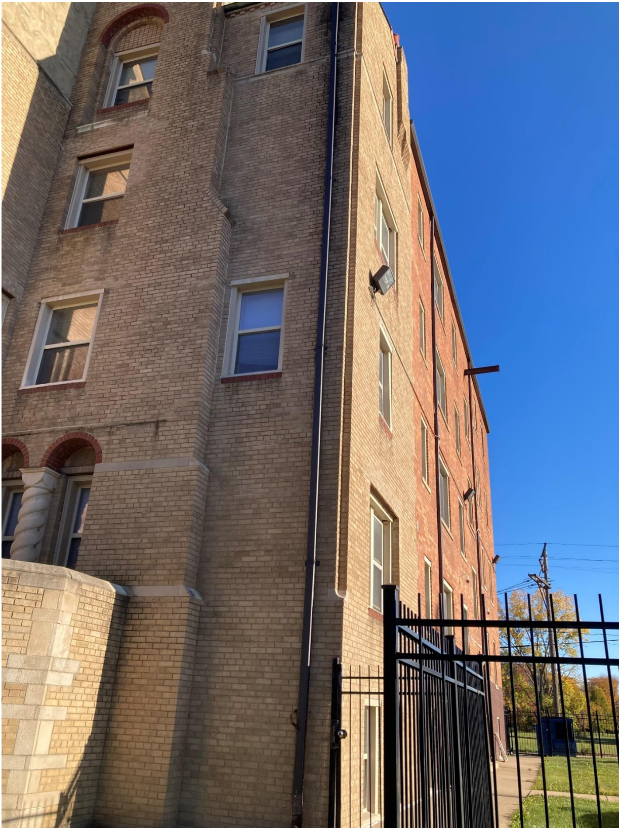
2725 W Boston, northwest corner. A downspout is shown and all of these are proposed for replacement. Staff photo, October 2025.
