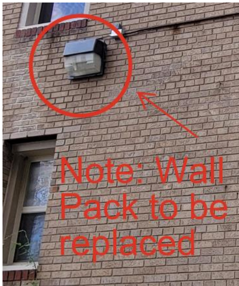
Existing typical security lights.
