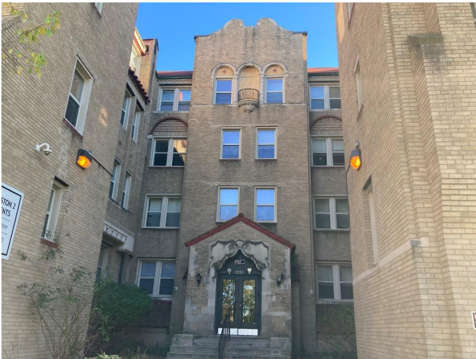
2725 W Boston, central courtyard and main entrance. Some of the building's rich architectural features are visible, including the balconette or Juliet balcony centered on the fourth floor between stone columns, the herringbone masonry in the arch over the windows on the third floor, and the ornamented masonry Arabesque arch over the main entrance. Staff photo, October 2025.
