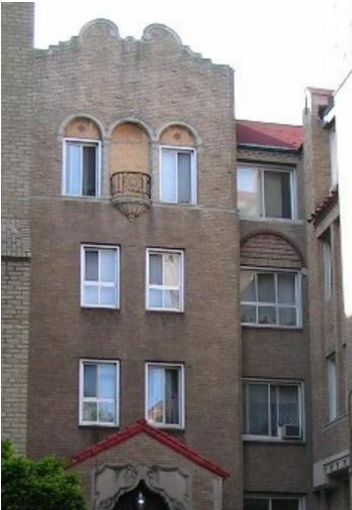
The designation slide photo from c. 2006 shows the red asphalt roofing, echoed by the red diamond tiles in the arches and red clay tiles on the right and again below, over the front entrance.
