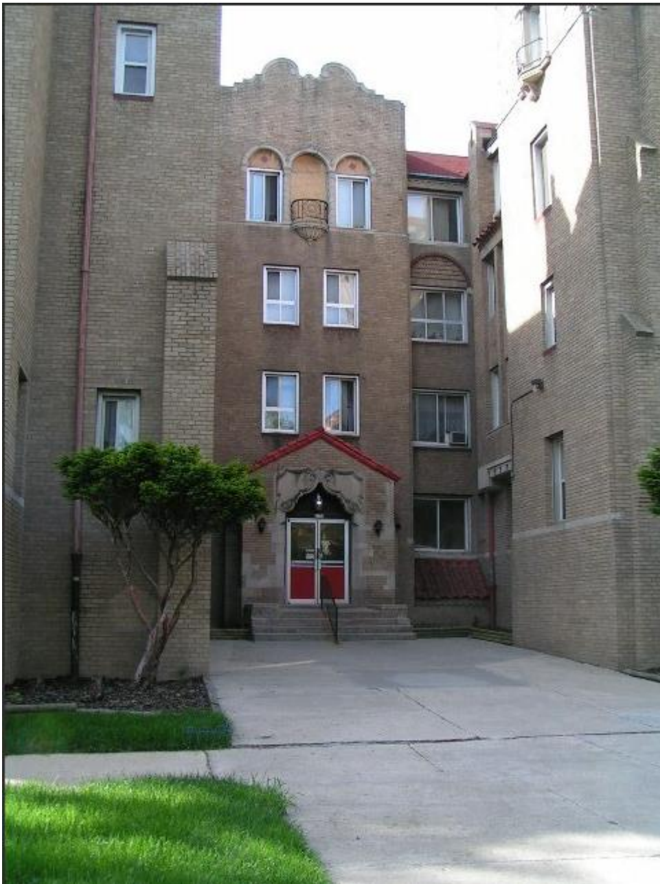
2725 W Boston, HDAB designation slide, c. 2006. Pictured are some of the inappropriate changes the report referred to, including slider windows. These inappropriate windows shown have since been replaced with double-hung vinyl windows.
