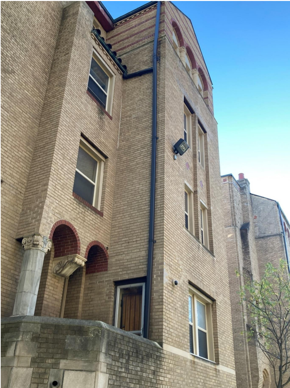
2725 W Boston, detail at northeast corner. The door shown is proposed for replacement with a door and storm door. Its corollary at the northwest corner is also proposed for replacement. Also shown are character-defining features including arches, a bracket, and a marble column. The brick staining here would likely be included in the proposed masonry cleaning. Staff photo, October 2025.
