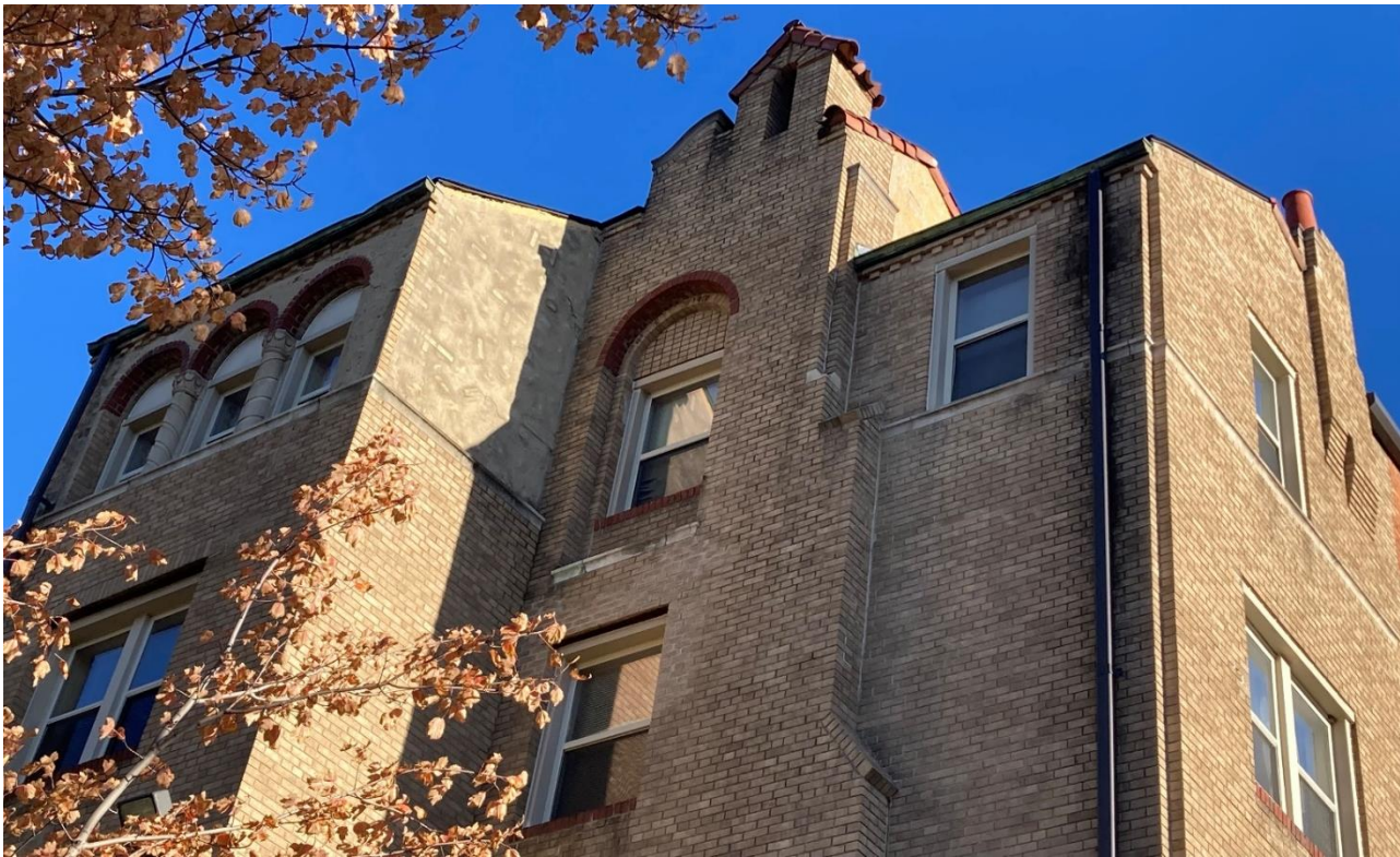
2725 W Boston, north side of west tower and northwest corner. Copper gutters and a nonhistoric downspout are shown and all of these are proposed for replacement. Some of the building's rich architectural features are also shown, including the tripartite arched window with columns, patterned masonry inset above the window in the arch, dentil molding, and the clay tile and varied roofline. Staining behind the downspout here would likely be targeted in the proposed cleaning efforts. Staff photo, October 2025.
