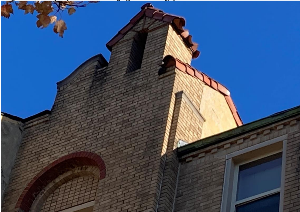
2725 W Boston, north wall of west tower, detail. Shown here is a detail of some dentil molding, copper gutter, the patterned masonry inset in the arched opening, the varied roofline, and some of the clay tile. Staff photo, October 2025.
