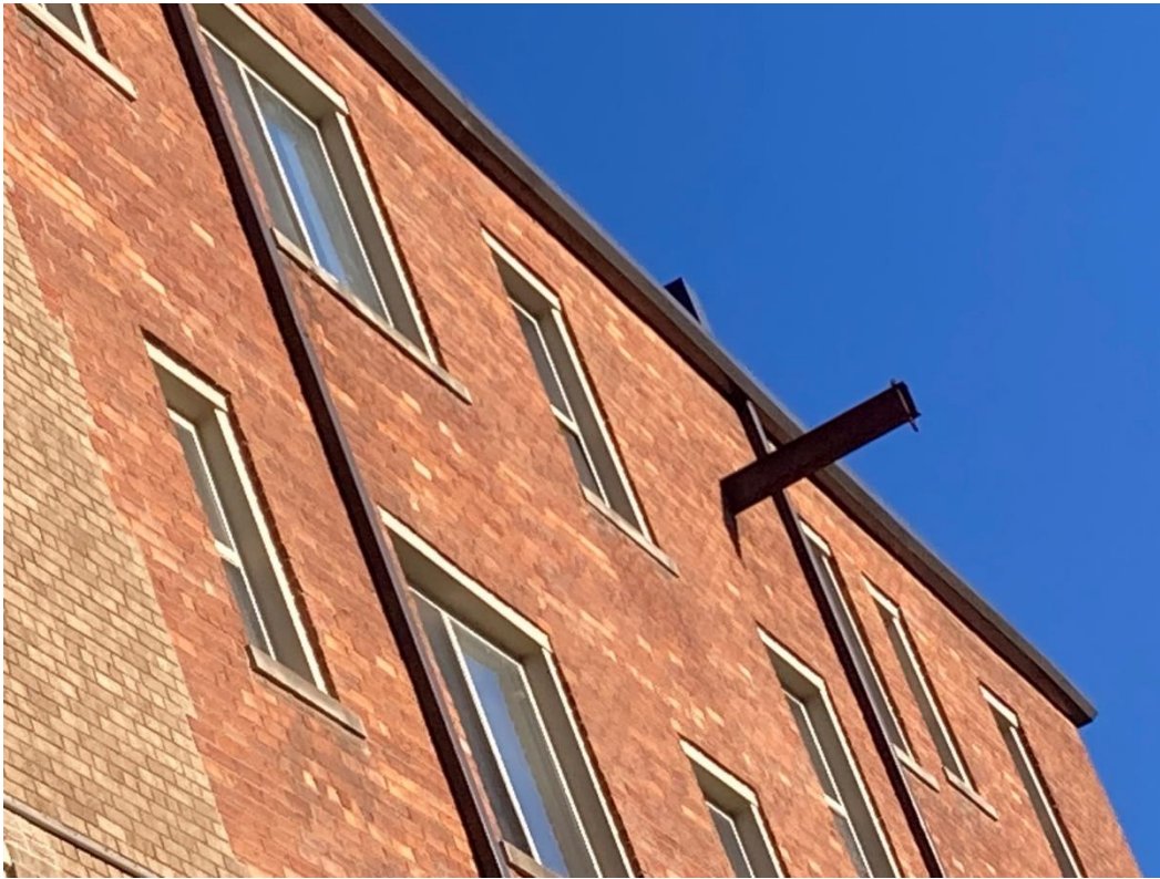
2725 W Boston, west wall, detail of gutter and downspouts. All gutters and downspouts are proposed for replacement. Nonhistoric gutter and downspouts appear brown here. Staff photo, October 2025.
