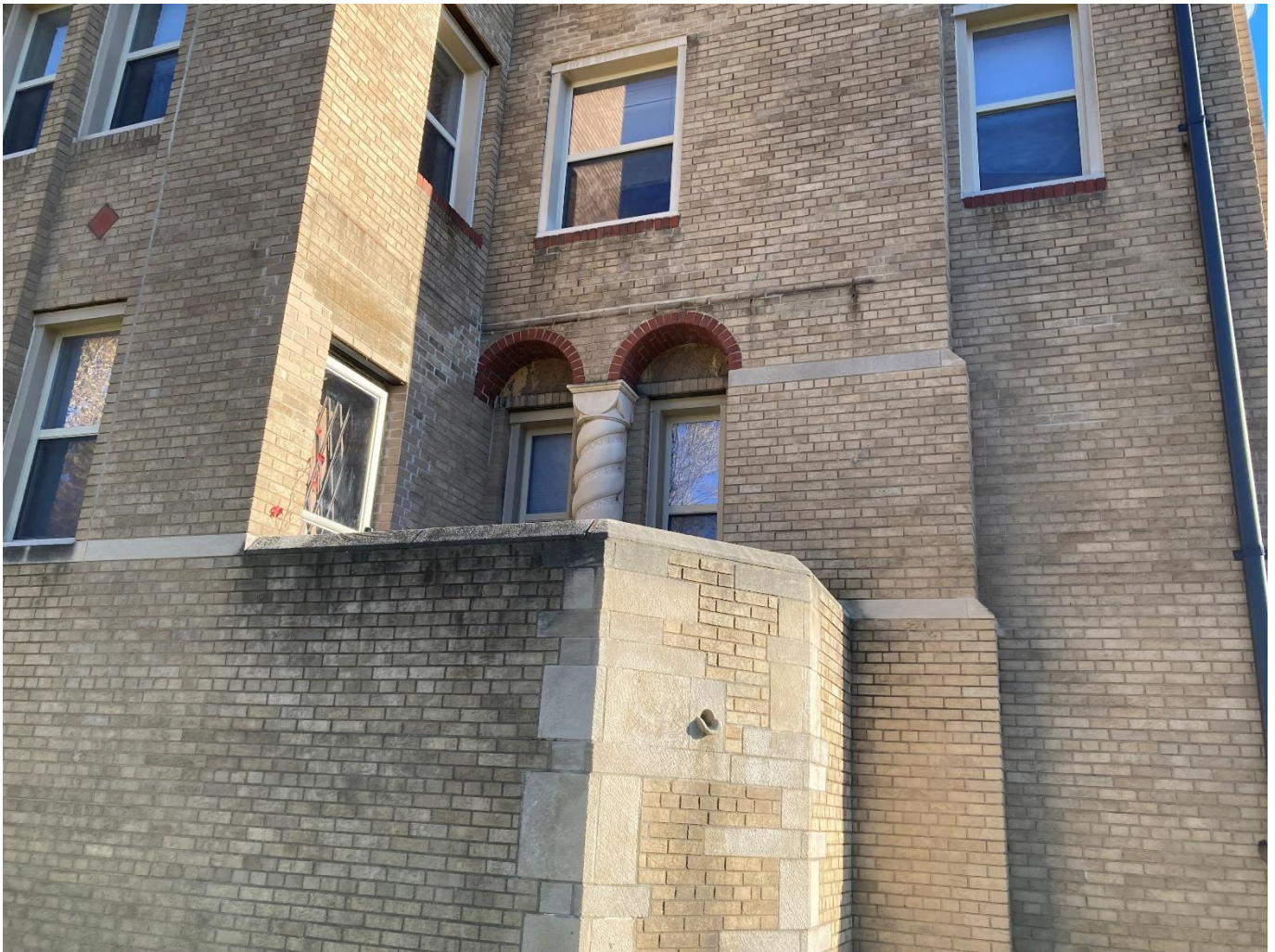
2725 W Boston, detail at northwest corner. The door shown is proposed for replacement with a door and storm door. Its corollary at the northeast corner is also proposed for replacement. Also shown here are the arches over windows, defined by red bricks, and an ornate stone column. Staff photo, October 2025.
