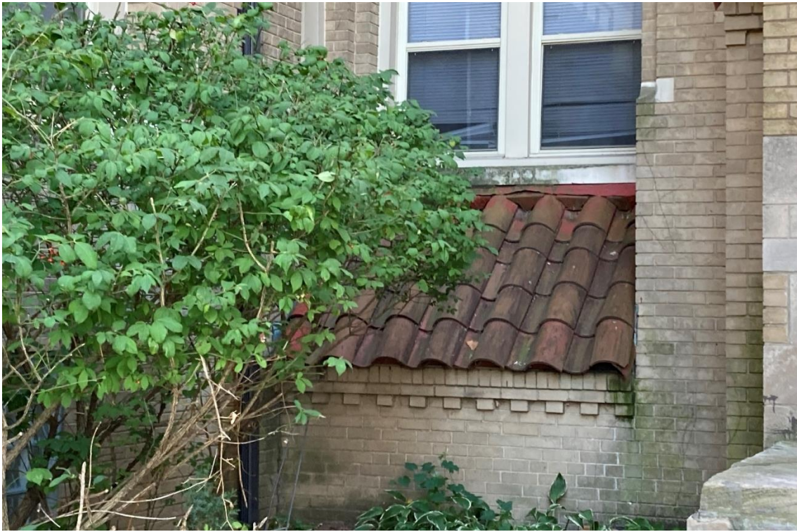
2725 W Boston, north (primary) façade, detail of pent roof covered in clay tile just east of the main entrance. Staff photo, October 2025.
