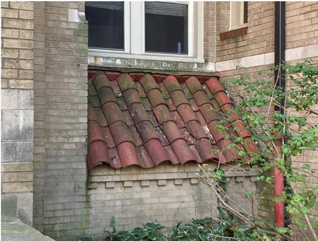
2725 W Boston, north (primary) façade, detail of pent roof covered in clay tile just west of the main entrance. Staff photo, October 2025.
