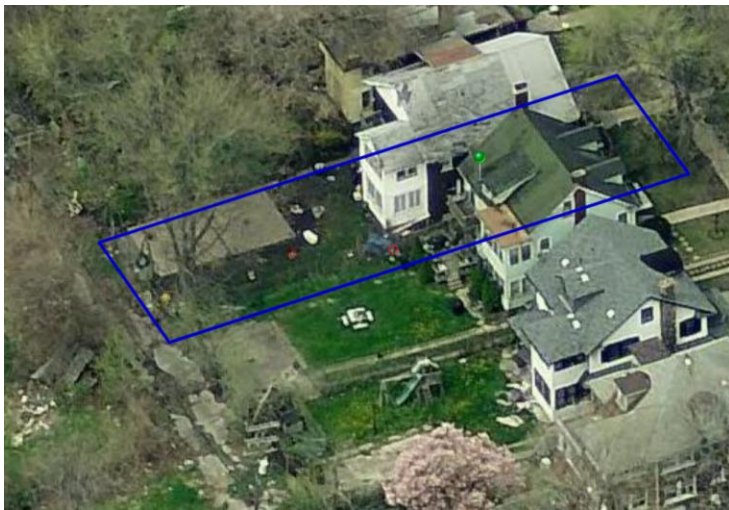
1427 Edison outlined in blue. Bird's eye view, 2011. Note that the garage has been demolished at this point, leaving only a concrete pad
