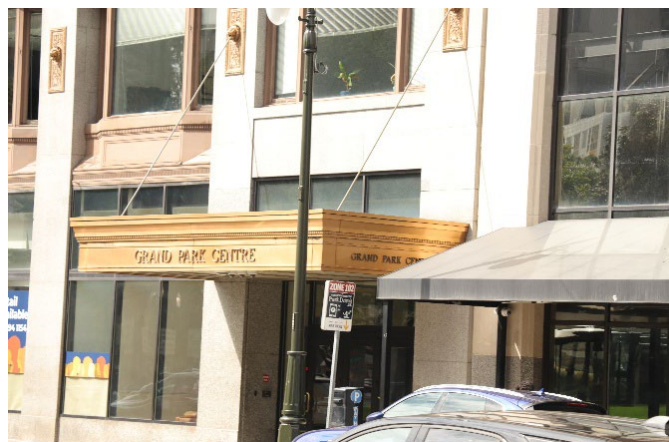
Grand Park Centre Roof Canopy Photo taken by Staff 09/24/2025
