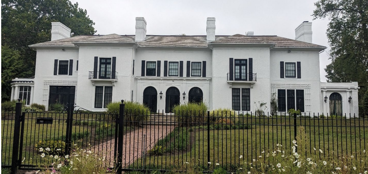
70 W. Boston - S. S. Kresge Mansion - front facade. Photo taken by staff on 09/25/2025.
