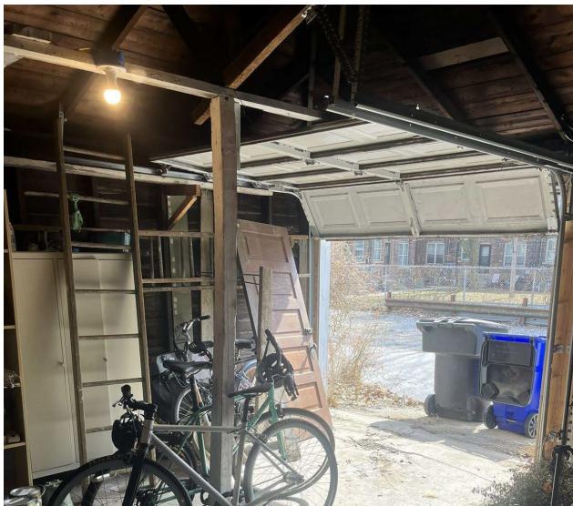
Photo provided by applicant, shows interior condition of the existing garage
