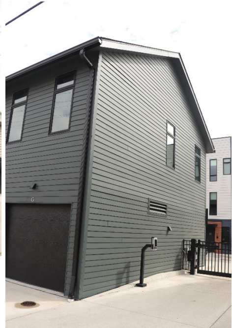
Right: New Construction, 2019 addition to neighborhood, seen on the opposite side of the alley, across from 1613 Leverette
