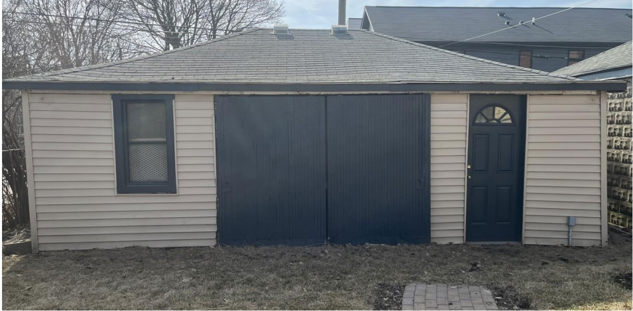
1613 Leverette garage, current appearance. Photo provided by the applicant.
