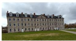
Building 507 is both the most prominent structure within the star fort and the oldest and the largest building at Fort Wayne. Located within the western perimeter of the star fort, the three-and-one-half-story building is constructed of coursed and roughly squared limestone masonry, built in the Federal/Adam style. Its front (east) façade is organized into five bays beneath a side-gabled, wood-frame roof, its center bay projecting slightly
