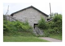
into the magazine. It retains the earthen embankment and braces the building walls with large limestone blocks located at various points around the perimeter. The building has a wood entrance door, and a thin brick barrel-vaulted ceiling with a wood framed and wood shingled roof.
