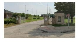
ashlar piers that have pyramidal stone caps and concrete foundations. Each pier formerly featured a metal plaque; these have since been replaced by signs identifying the site as Historic Fort Wayne, on one side, and the Army Corps of Engineers, on the other. The entrance originally had a decorative iron gate.
