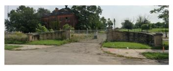
remains of the original 1905 design. Originally the wingwalls flanked chamfered ashlar piers, into which were set arched pedestrian entryways. The piers supported a pair of iron gates. Atop each pier was a stone sculpture—a mortar on the western pier and a cannon on the eastern one. Today, the piers and gate no longer exist, having been replaced with an aluminum chain-link, barbed wire gate. The mortar and canon sculptures were moved to sit atop the 1938 entrance to the star fort.
