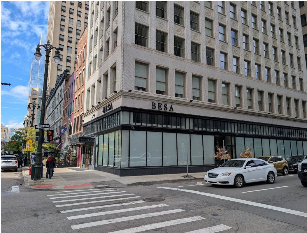
Location #2 at 600 Woodward in the Vinton Building and Financial District HD (wide view to the northeast). The Vinton Building is the corner structure. Staff photo, September 24, 2025.
