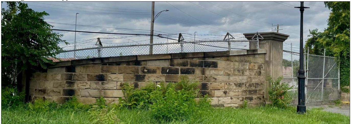
Interior view (looking northeast towards W. Jefferson) of the 1860s entry walls shows how the non-climbable fence was installed on top of the stone walls at the east entry gate, and the existing chain link gate retains barbed wire at the top. Staff photo, July 17, 2025.
