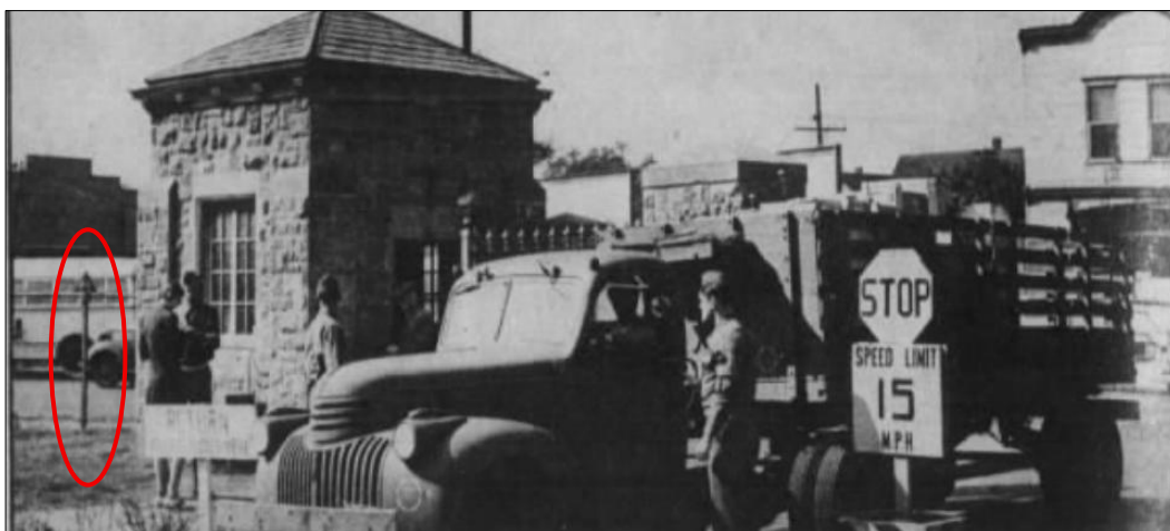
1943 interior fort photo of the primary "west" entrance looking (northwest) towards W. Jefferson. The chain link fence, visible to the left of the sentry structure now has thicker posts and "A"-shaped barbed wire toppers. Burton collection.
