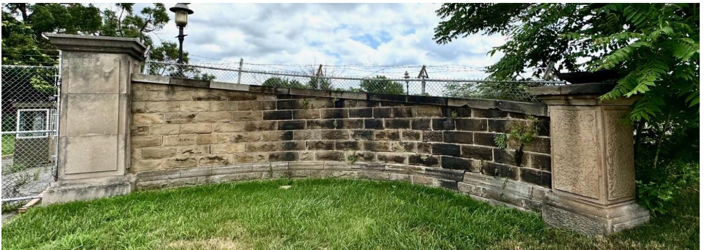
East side wall. Staff photo July, 17, 2025. This view clearly shows the different design and surface texture of the ca. 1860 pier (right) in contrast with the smooth surface texture of the taller pier (likely installed early 20 th century, or when the chain link fence was installed on the stone wall).
