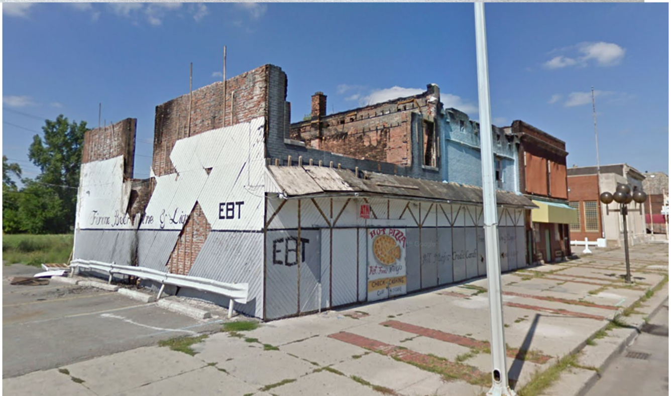
Google Street View image from August 2009, showing substantial fire damage to westernmost building. Note second story wall separating this building from the center building, apparently intact.
