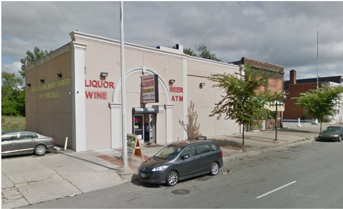
Google Street View image from September 2013, showing the store in operation with the incompatible EIFS/dryvit façade system.
