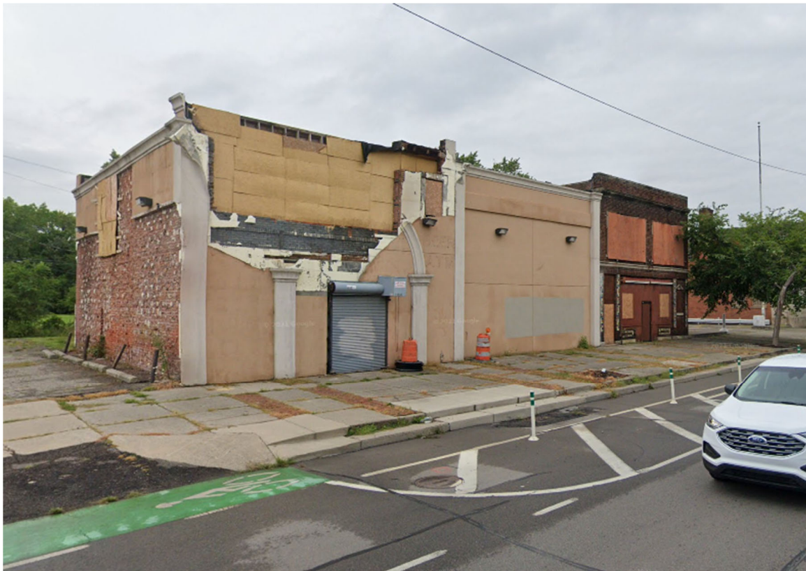
Google Street View image from August 2021. At least four years after closing the store, the unapproved façade system has apparently collapsed at the side and at the front, revealing what appear to be haphazard repairs of the original damage from 2009.
