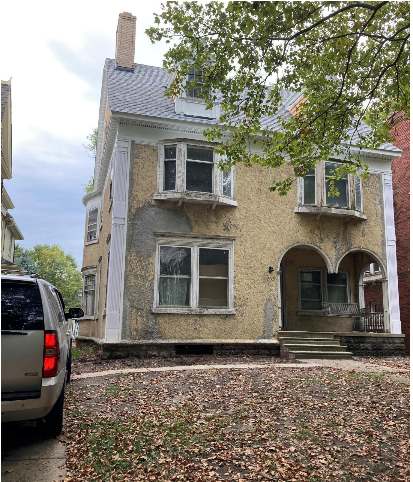
East (front) end of house, with south side barely visible, trim repairs in cornice complete, vinyl corner boards installed, some stucco repairs have been started, and porch column is missing, staff photo, September 2025.
