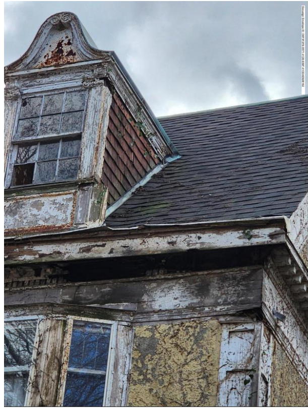
Applicant photos of wood trim conditions, April 2025. Ornate trim detailing is evident, along with missing and damaged pieces.
