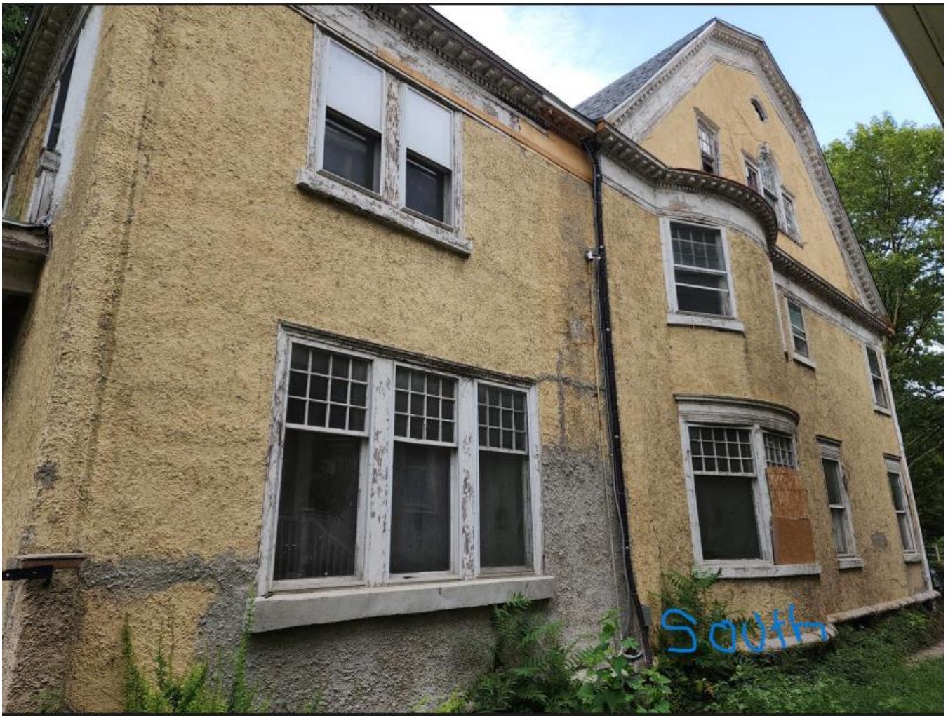
Applicant's photo, September 2025, from Cycle 4 application materials. Some like-for-like wood trim repairs are visible, as well as some of the house's highly detailed windows mentioned previously.
