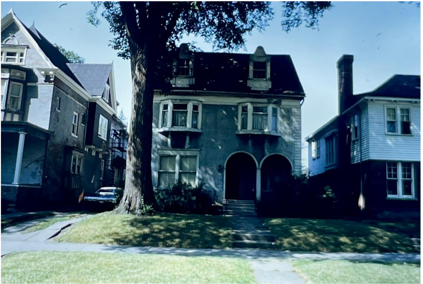
863 Iroquois, designation slide, c. 1971. Ribbon drive and quoins at northeast corner are visible.
