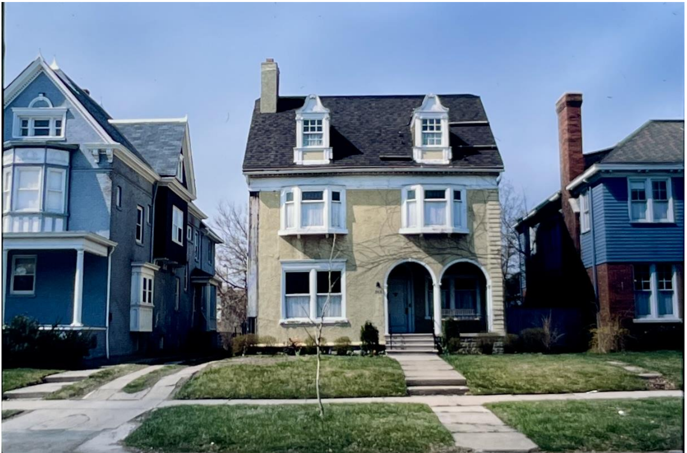
863 Iroquois, slide from PDD file, April 1980. Ribbon drive and quoins at northeast corner evident, but they are missing from the southeast corner.
