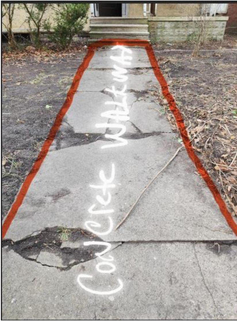
Applicant's photo, May 2025 from Cycle 3 materials, clarifying proposed walkway only in concrete.
