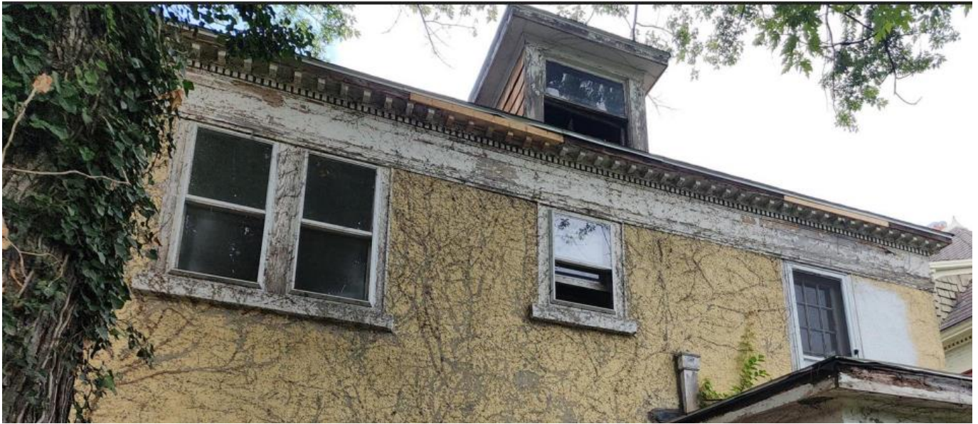
Applicant's photo, September 2025, some like-for-like wood trim repairs are visible.
