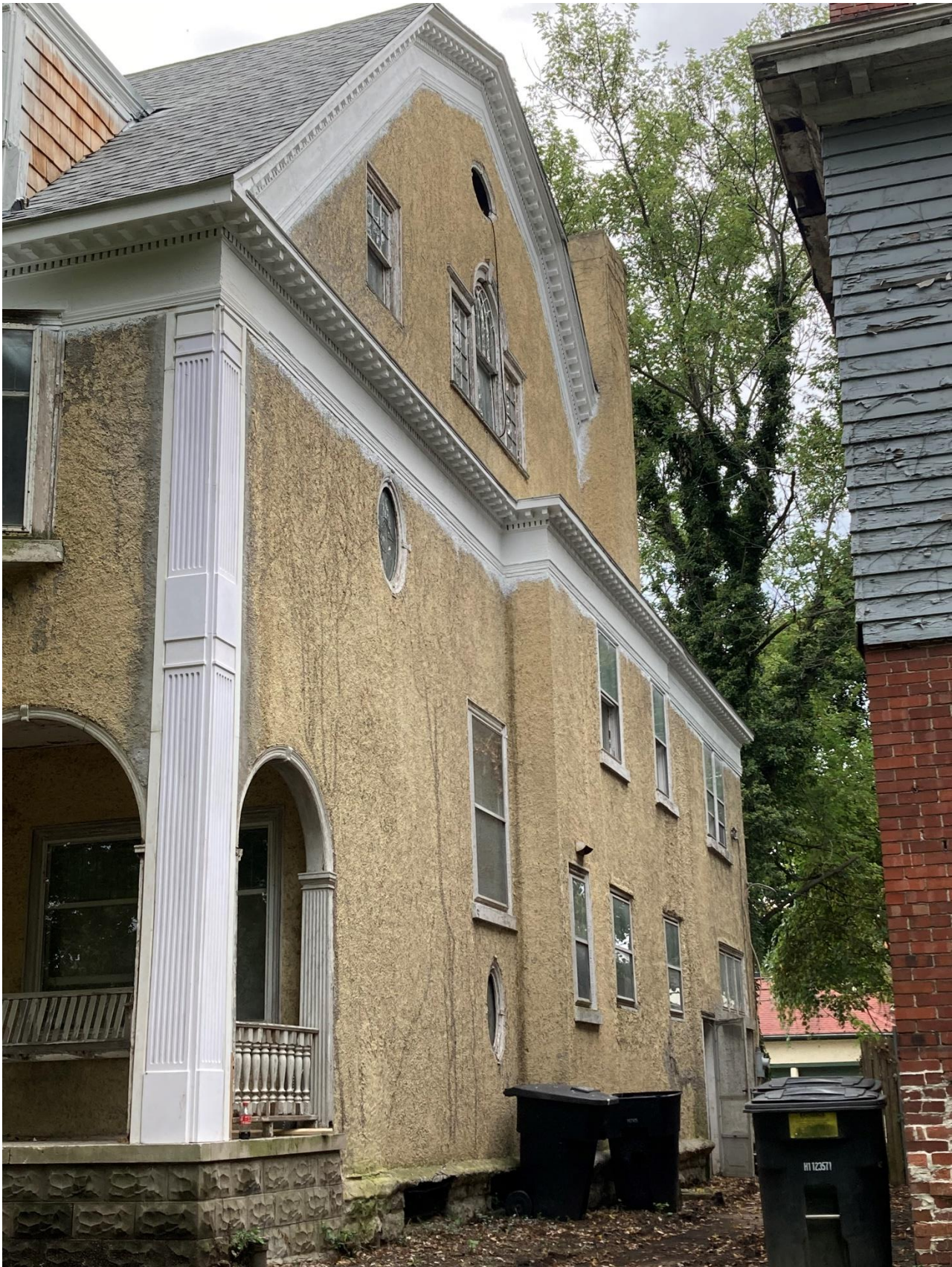
Staff photo, September 2025, northeast corner with vinyl corner board and north side visible.
