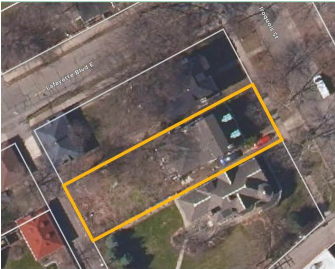
863 Iroquois, Detroit Parcel Viewer. It appears that the dormers are roofed in copper. The roof work permitted in May specifically excluded work on the dormers.
